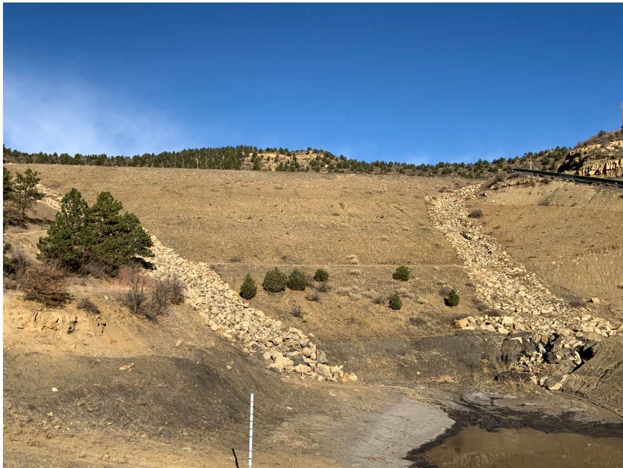
Refuse Disposal Area – Reclaimed Benches and Armored Drainage
