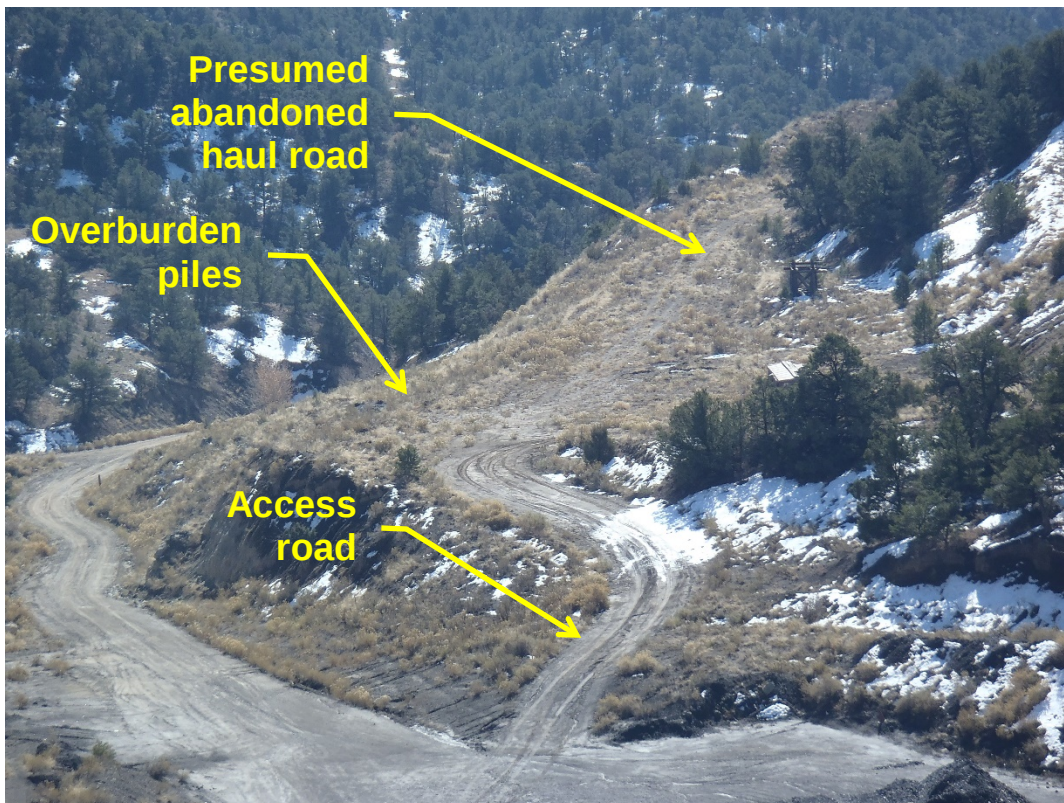
Photo 1. Revegetated overburden piles on the west side of the access road and presumed abandoned haul road (looking south).
