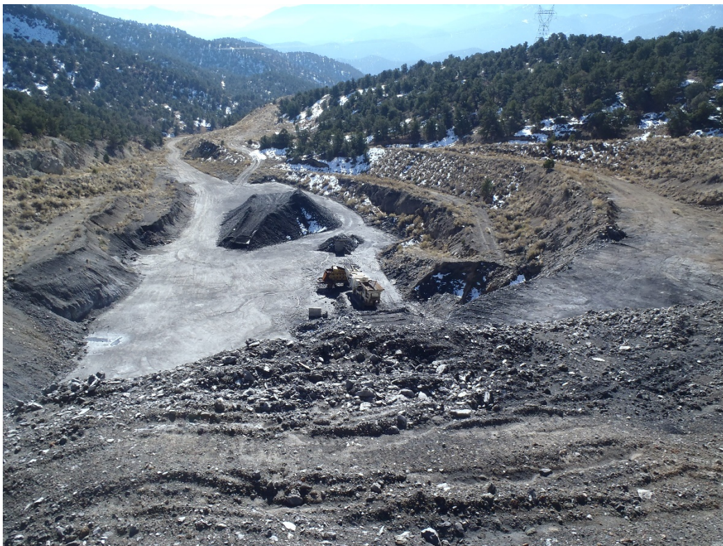
Photo 3. Mostly reclaimed benches on west side of pit (looking south).
