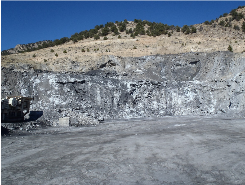
Photo 2. Active pit highwalls (looking north from pit floor).
