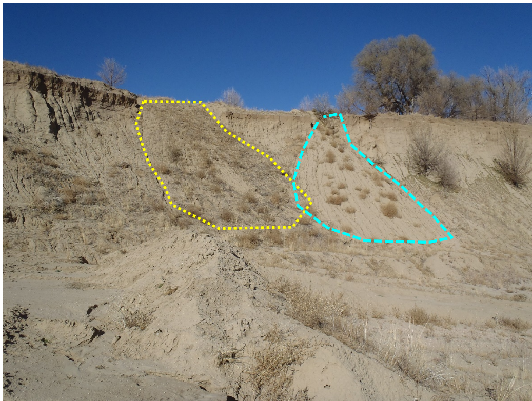
Photo 4. Previously repaired area (yellow) next to newer eroded area (blue) (looking north from NW corner of new wash pond [FMIC ditch just beyond highwall crest]).
