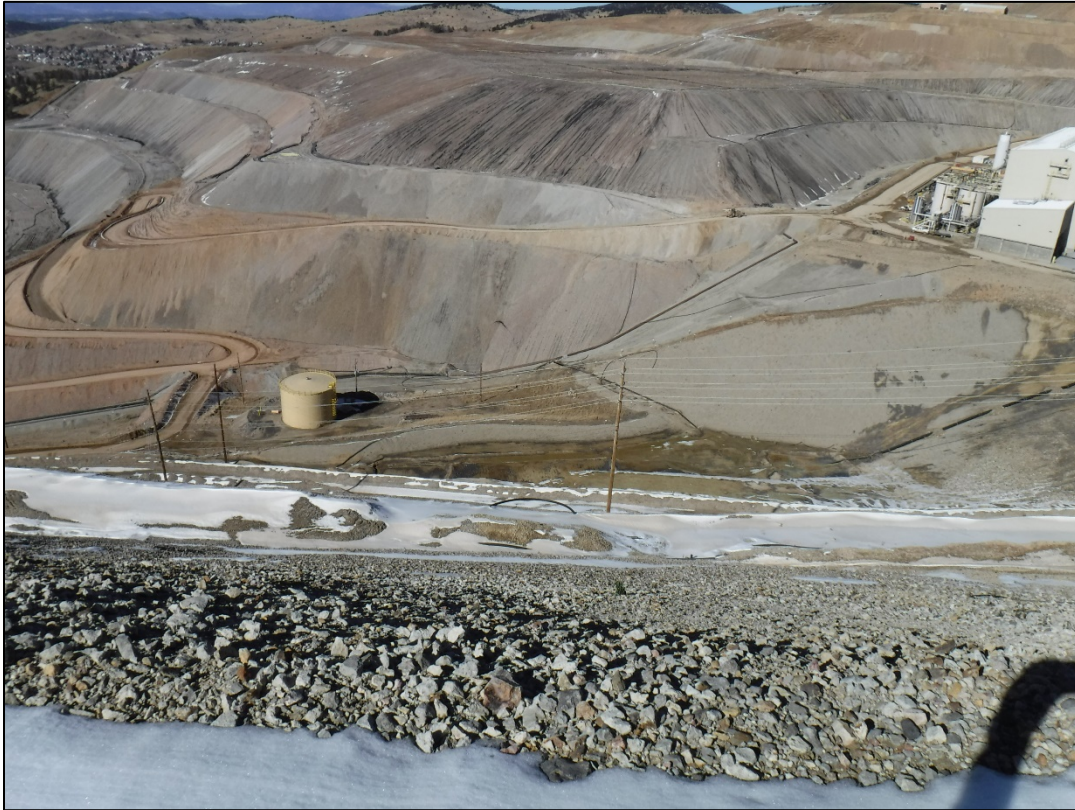
Photo 11: Water storage tank and elongated sump on VLF 1
