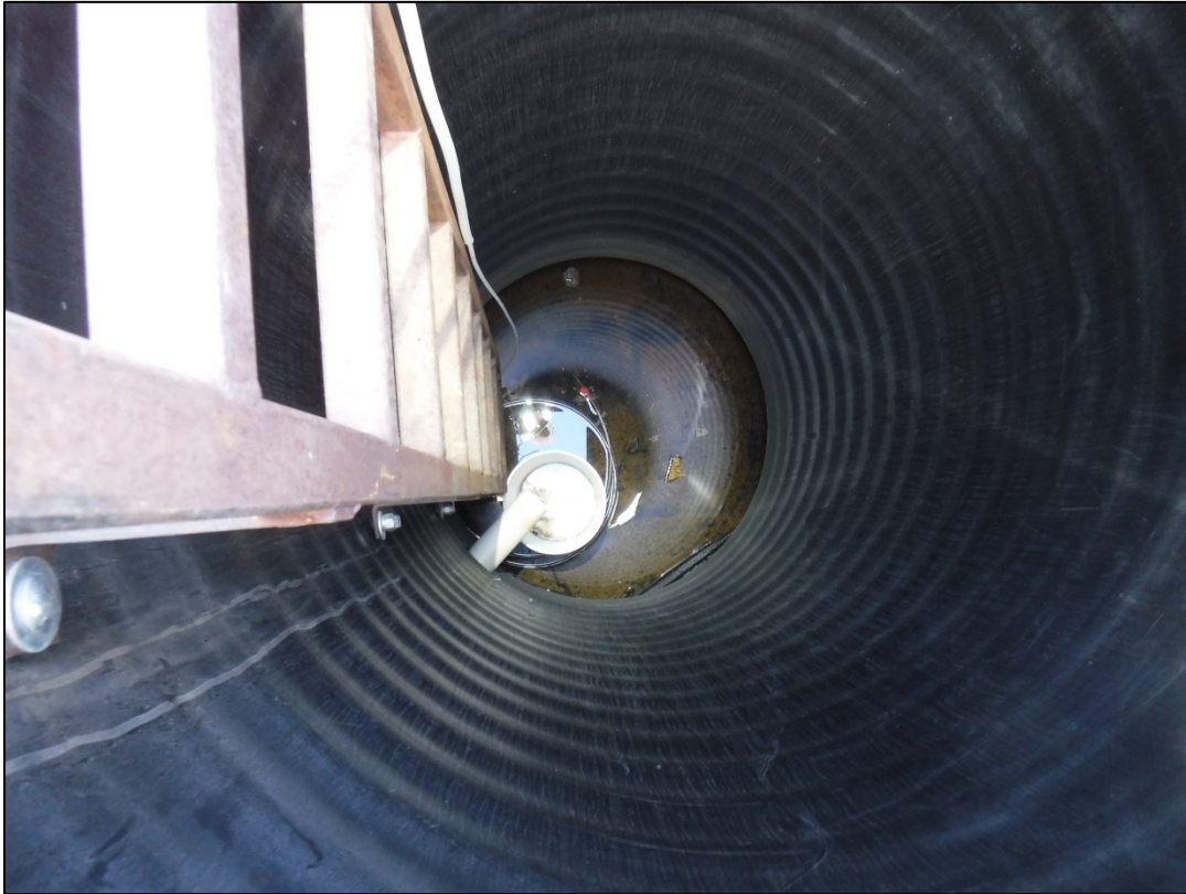
Photo 3: Inside LDS 3 note water in bottom of sump but bucket is dry
