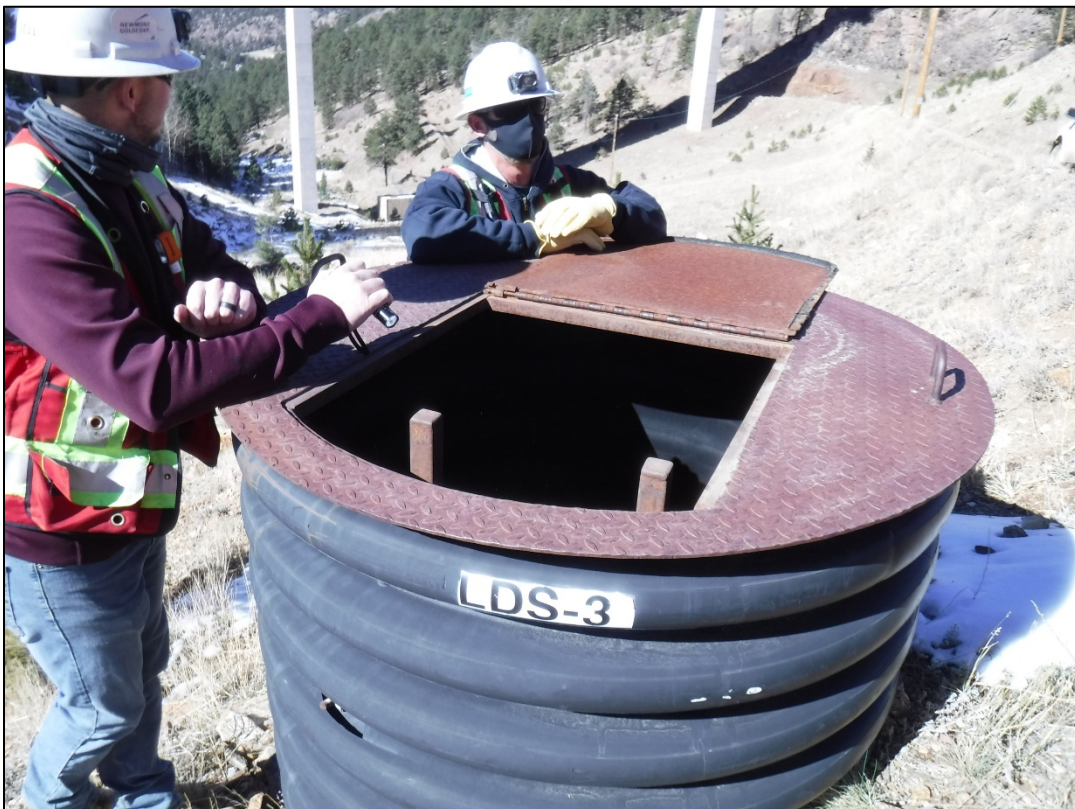
Photo 2: Leak detection system (LDS) sump number 3
