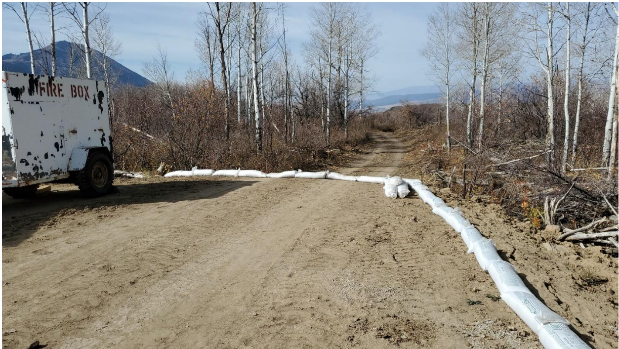
Figure 21: SS1-5 sediment control
