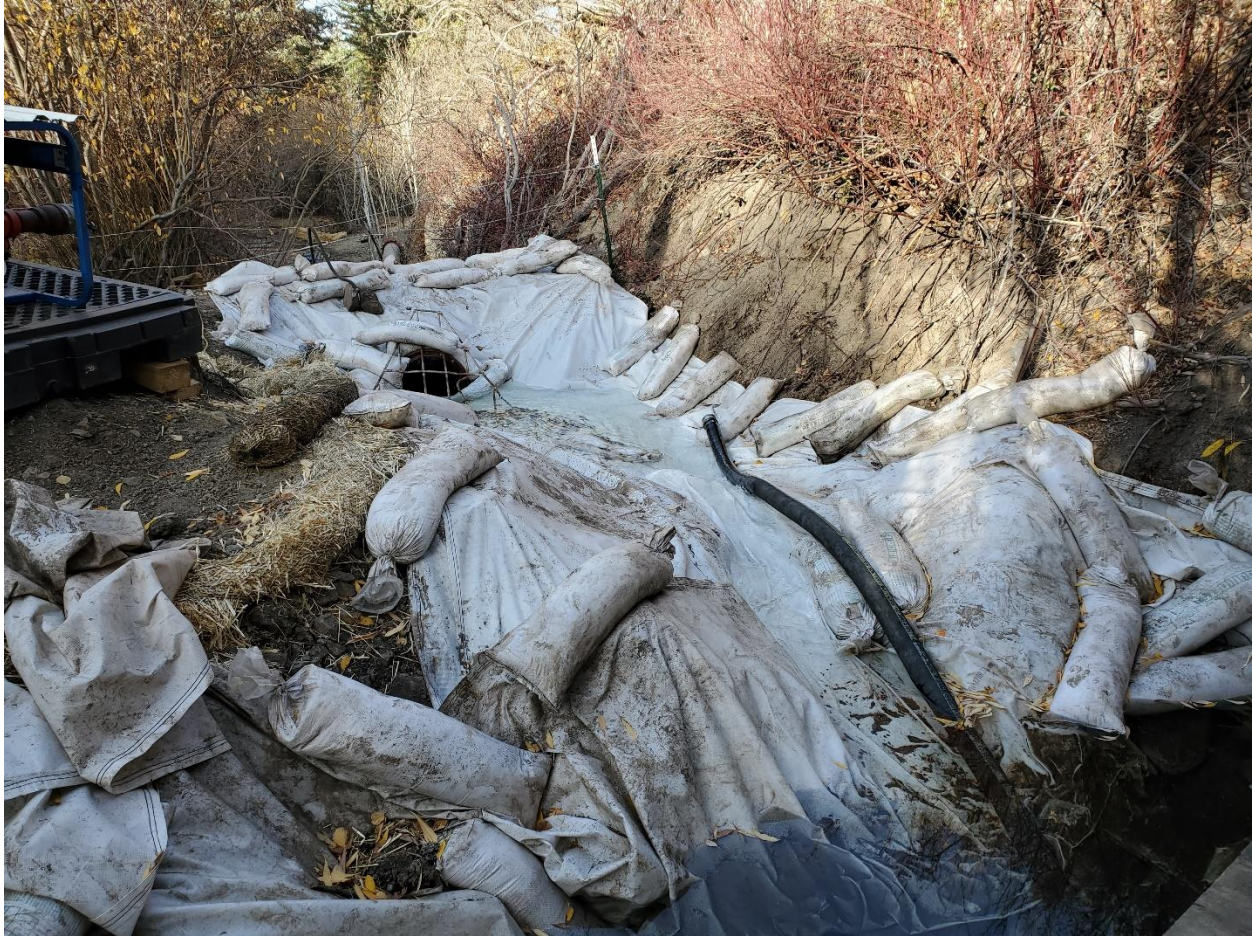
Figure 4: Sump at inlet to temporary diversion
