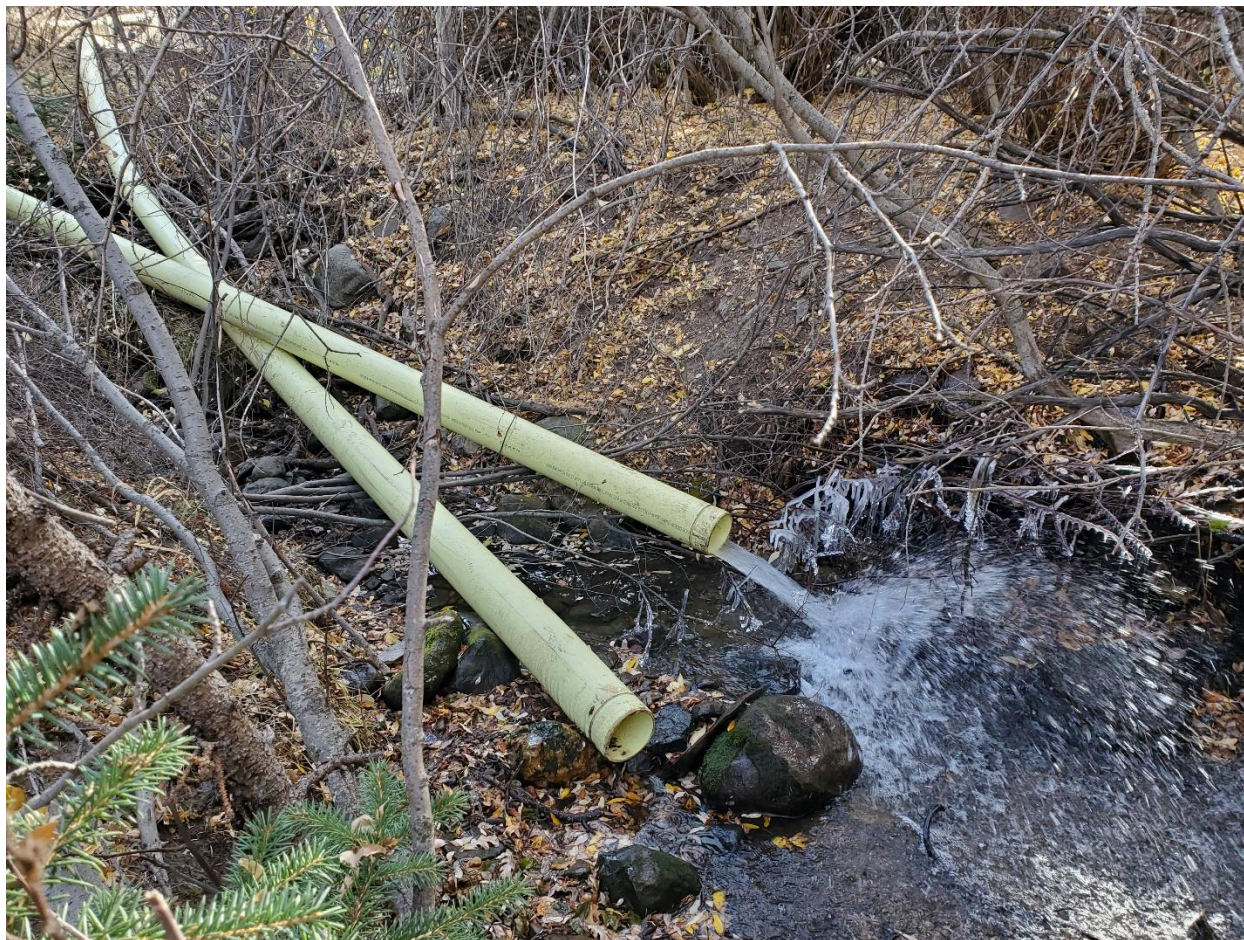
Figure 7: Outlet of temporary diversion
