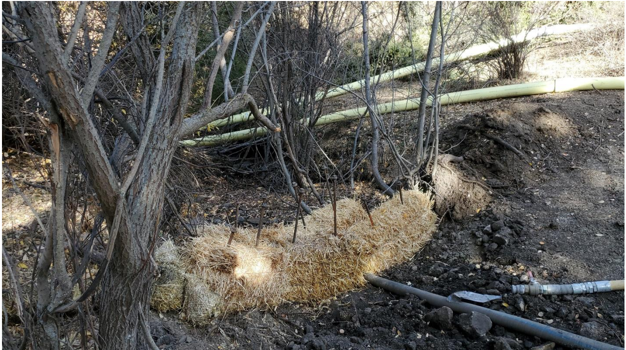
Figure 12: South Prong Creek channel protected from disturbed area run-off with straw bales
