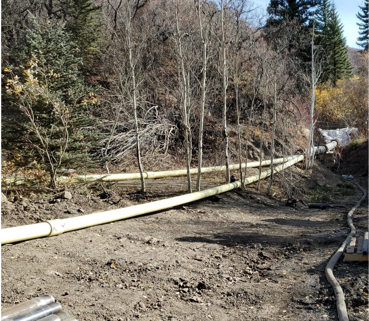
Figure 6: 16" pipe splits into two 6" pipes, one in use the other for surge capacity
