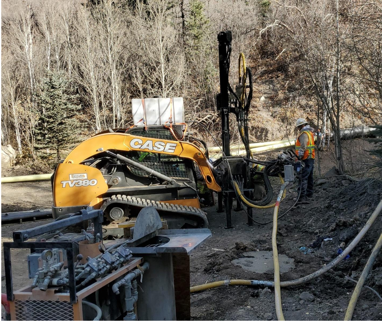
Figure 16: Skidsteer mounted drill rig, positioned over second hole. First hole visible in foreground.
