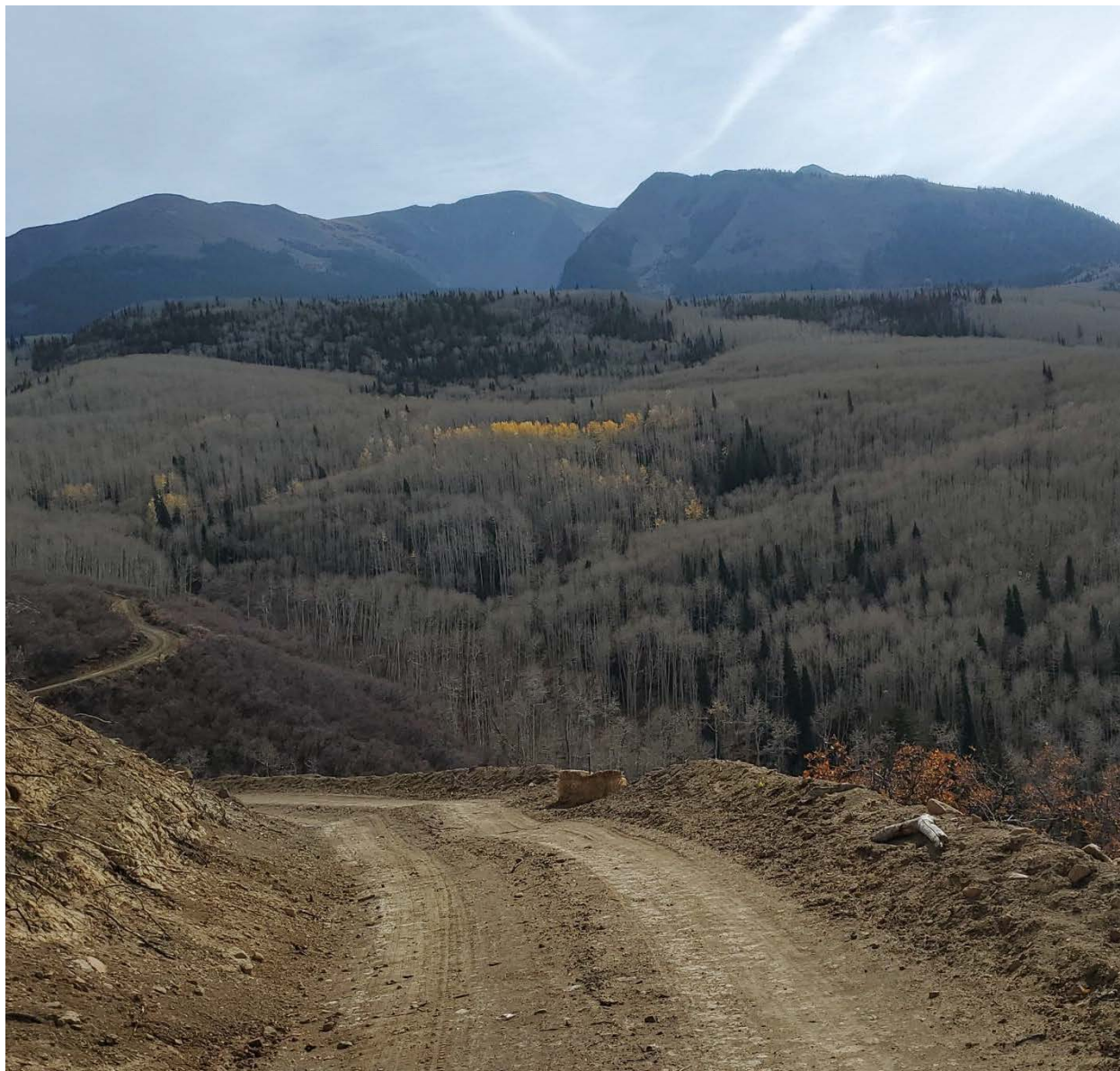
Figure 23: Refreshed straw bales for sediment control on SS1 road
