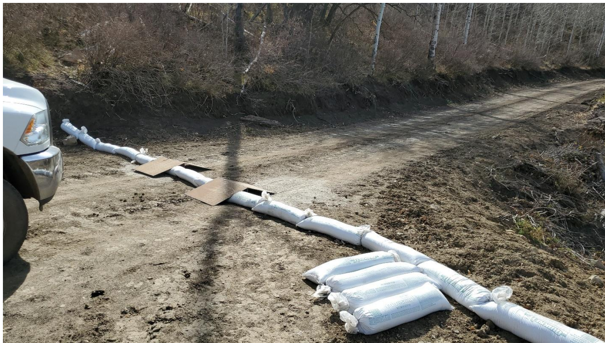
Figure 17: New sandbags for sediment control on SS1-1 pad (1)
