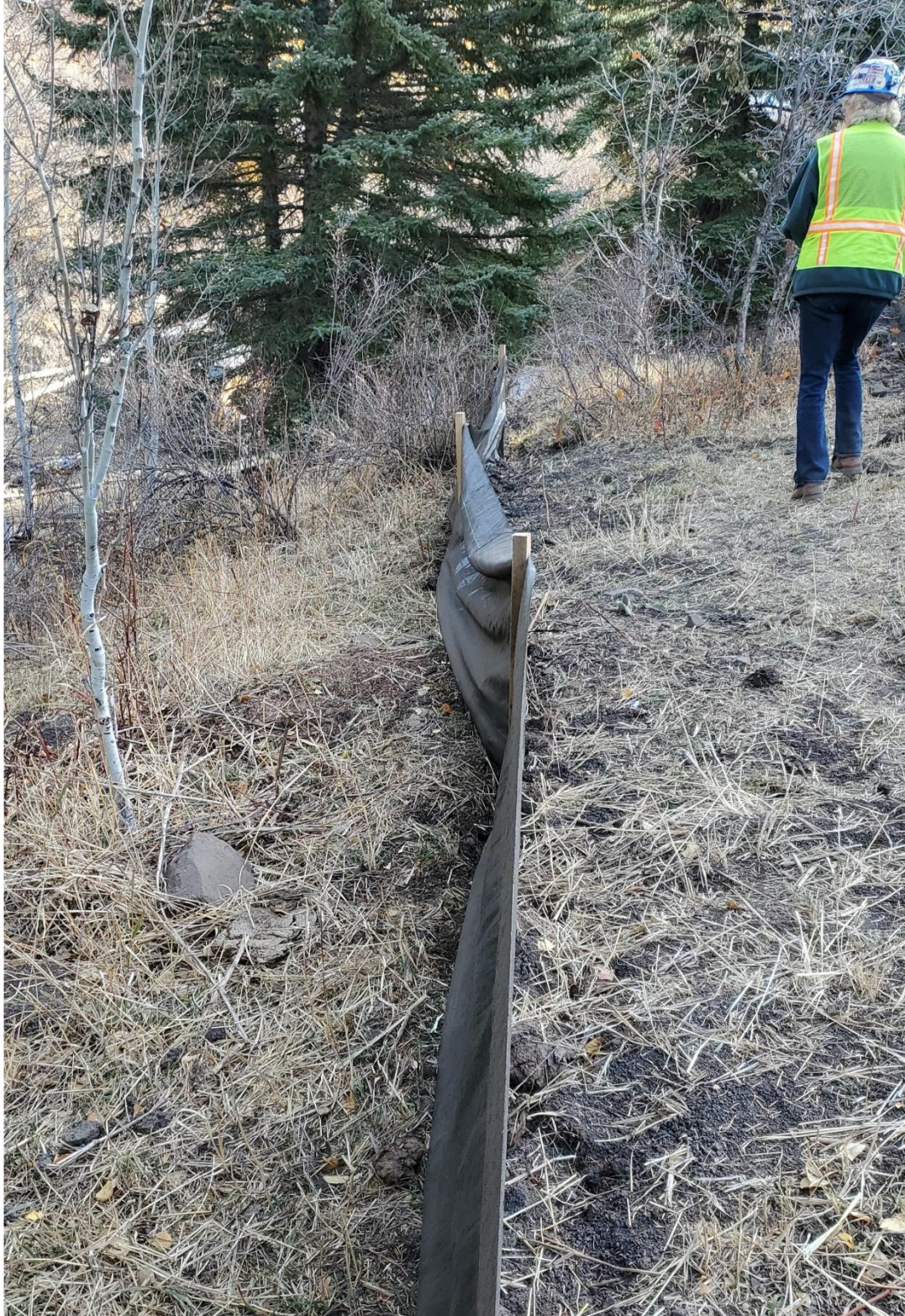
Figure 11: Disturbed area run-off controlled by silt fence (2)
