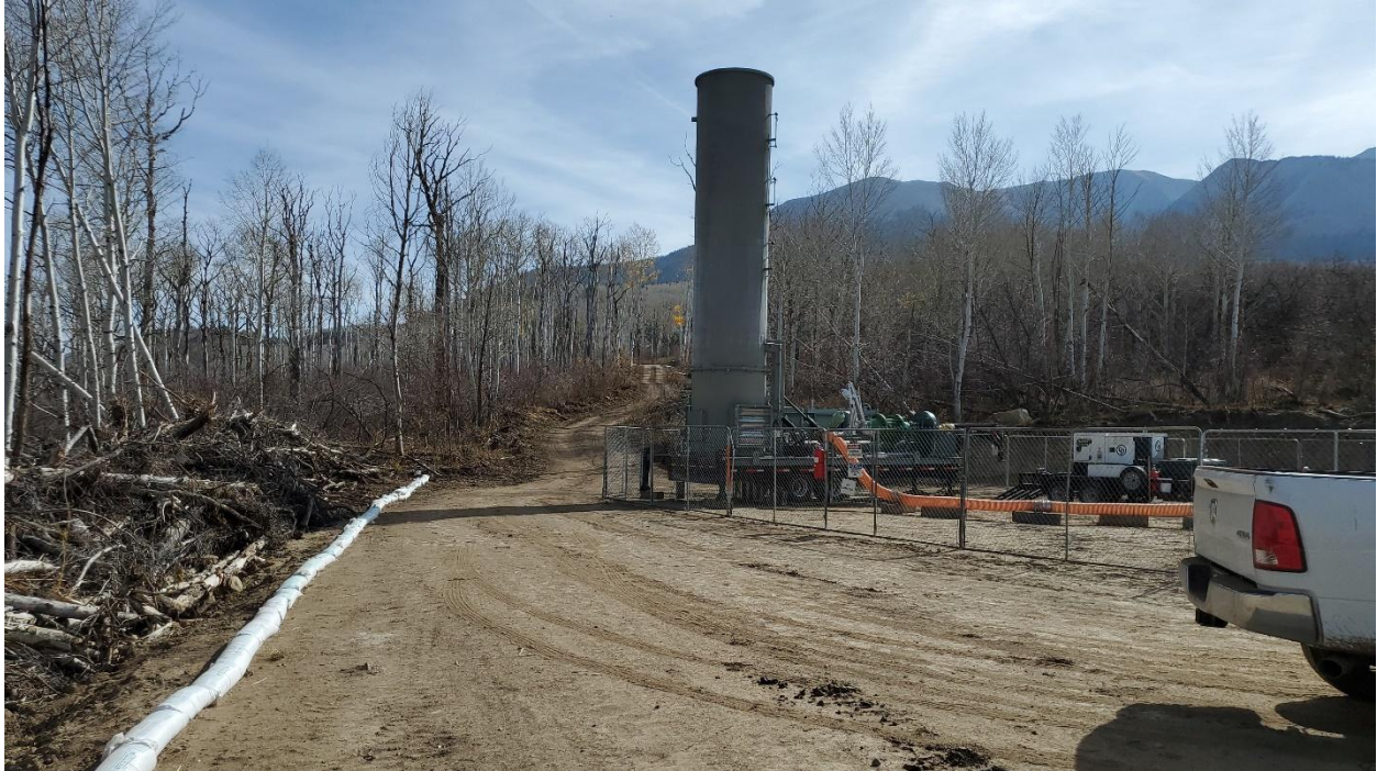
Figure 20: Mobile flare on SS1-5. Sandbags for sediment control shown
