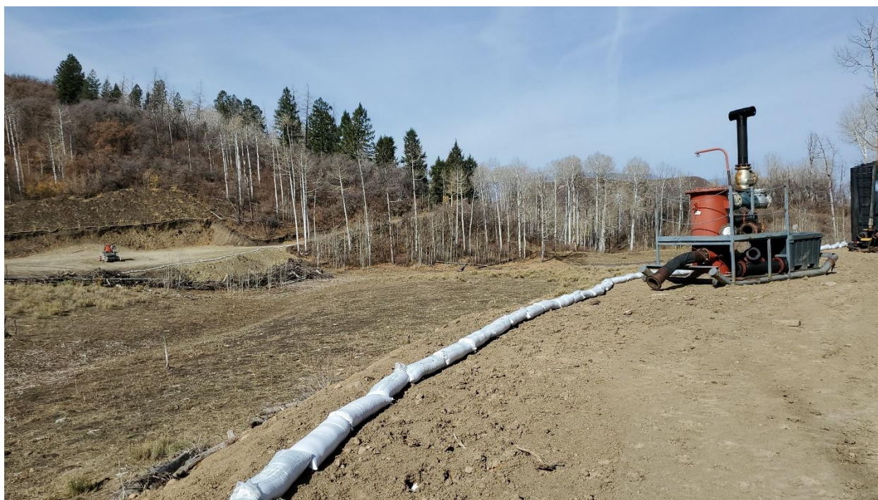
Figure 18: New sandbags for sediment control on SS1-1 pad (2)
