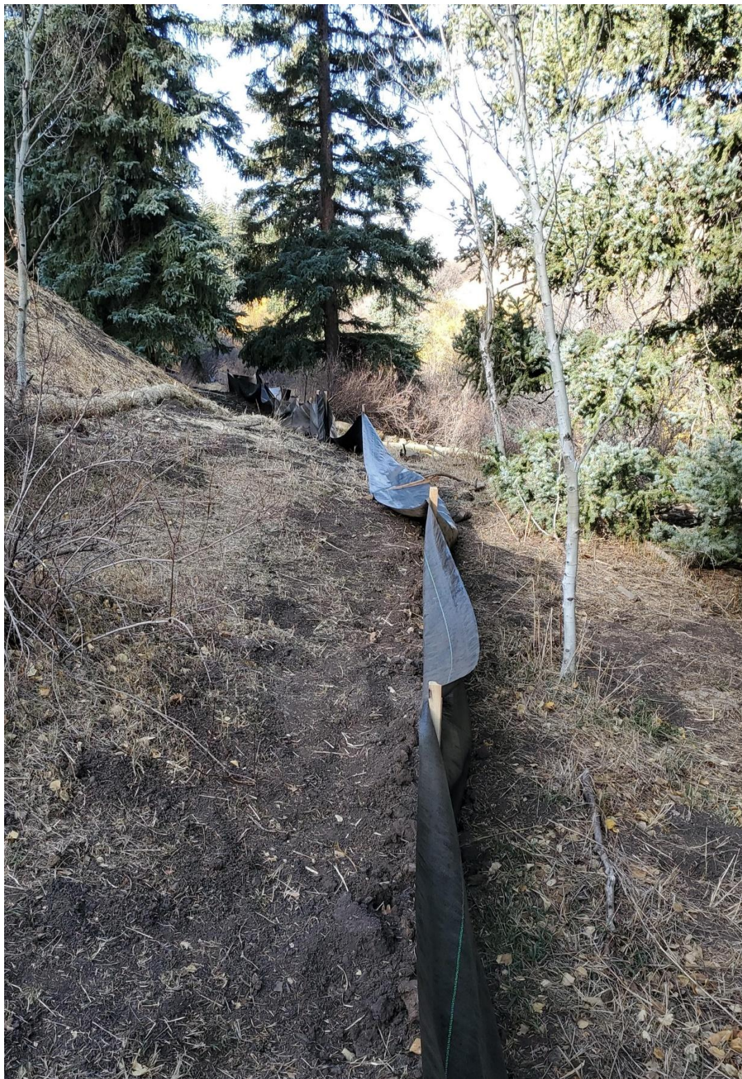
Figure 10: Disturbed area run-off controlled by silt fence (1)
