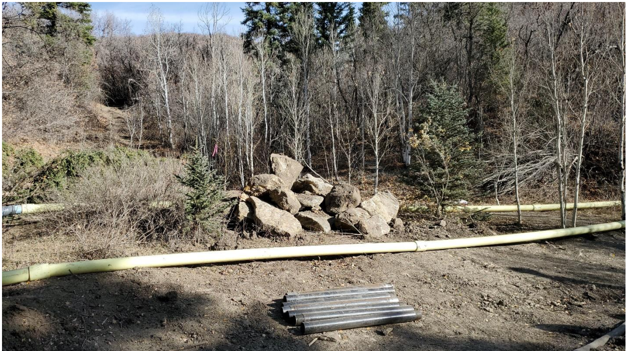
Figure 13: Stockpiled cobble and boulders, with 5' lengths of 5.5" drill casing in foreground
