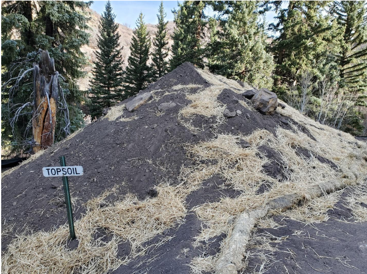
Figure 9: Salvaged topsoil, signposted, mulched, and protected with straw wattle
