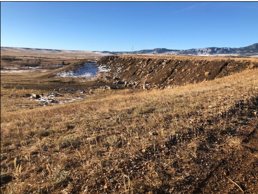
Photo 2. Closer view of eastern edge of lower lift placed inside pit in north mining area. Side slopes of this lift are at ~1.5H:1V.
