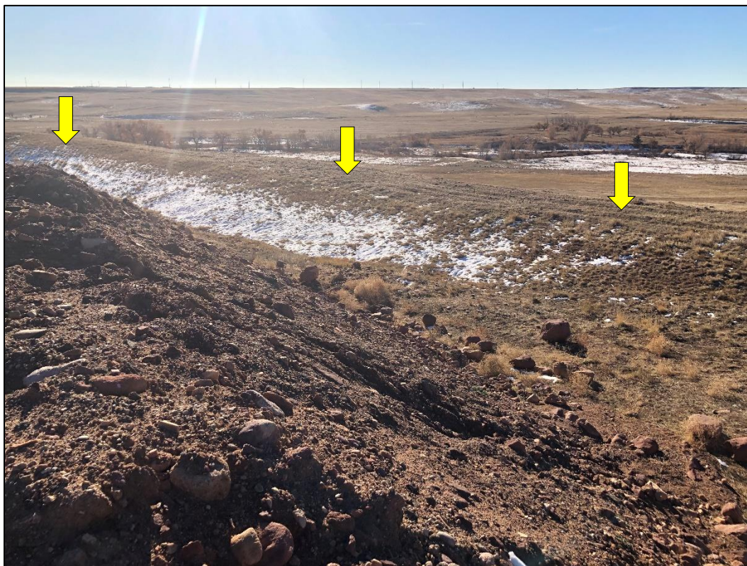
Photo 11. View looking southeast from top of upper lift placed inside pit in north mining area. Note side slope of upper lift (in foreground) at \sim 1.5H:1V . Also note southern rim of pit (indicated in background).
