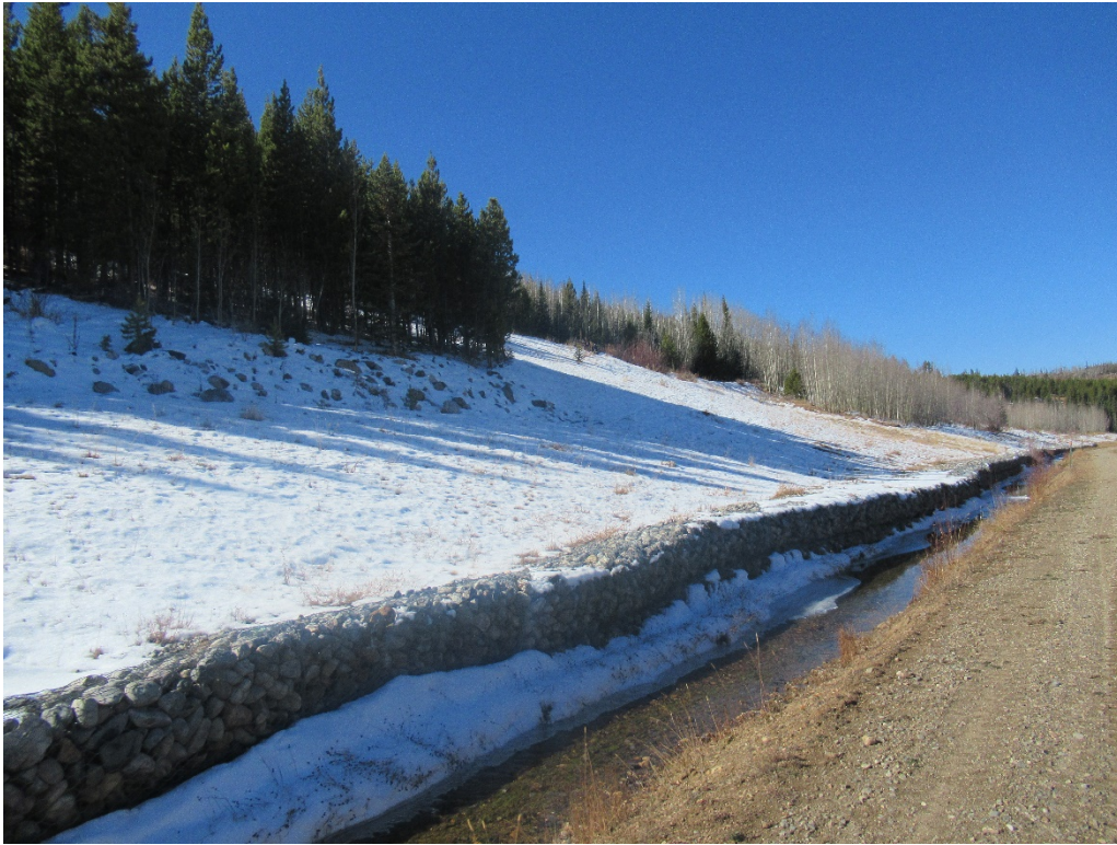
Gabion structure along the Ultimate Canal
