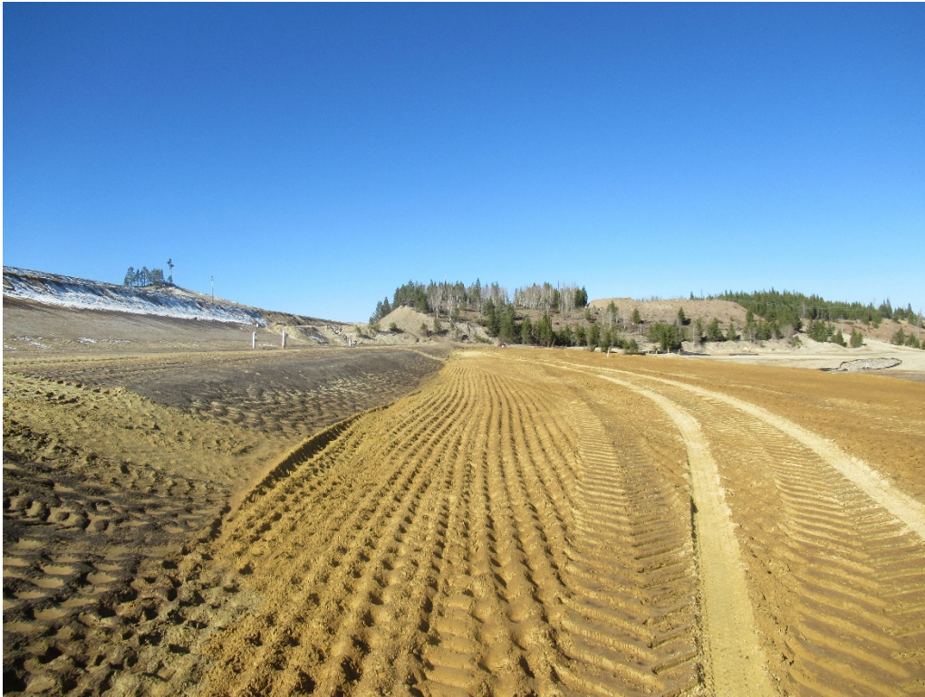
View of the upper bench of the upper face of the 3-Dam north area buttress
