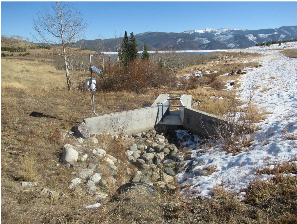
Inlet weir from the Ultimate Canal to the tailings impoundment
