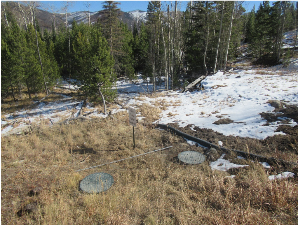
View of the 3-Dam seepwater collection vault covers
