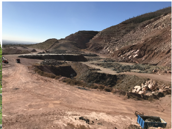
2. FILL STOCKPILED FOR FUTURE PLACEMENT
