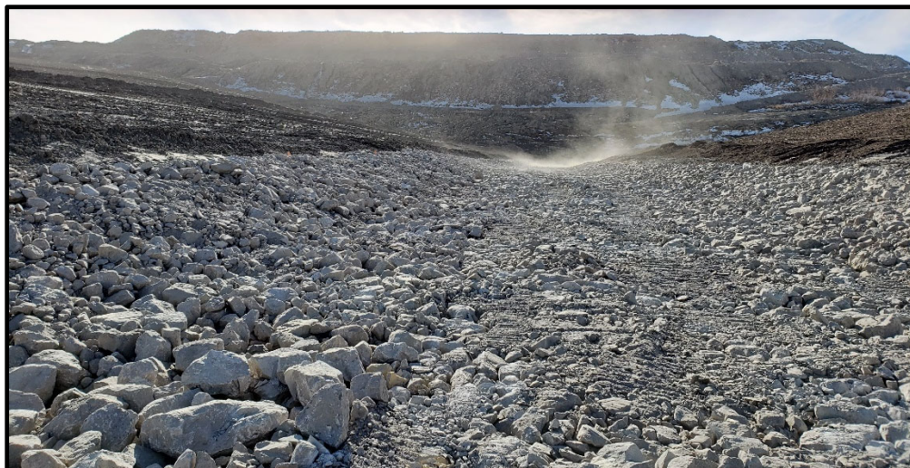
Photo 1 taken 11-11-19. Taylor Tributary Ditch looking south from the center of the inspected section.
