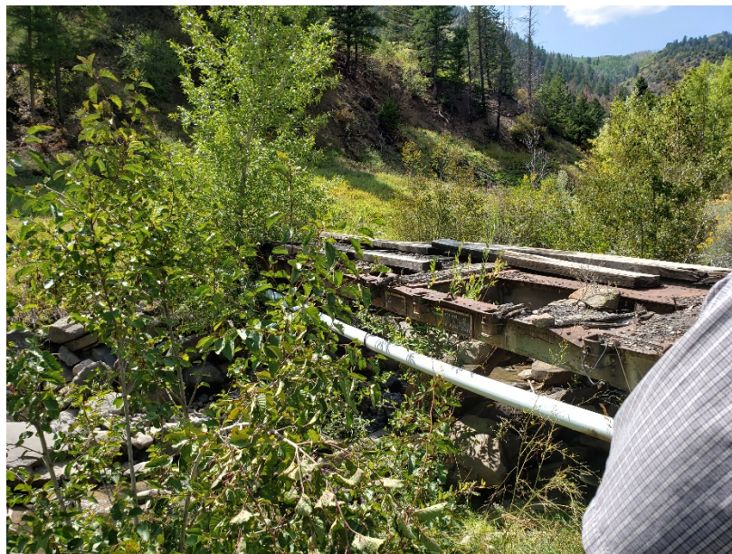
Figure 3 - Although difficult to see in this picture, one support of the portal pipe attaching it to the bridge failed, creating a sag in the pipe. The pipe should be re-supported to eliminate this sag.
