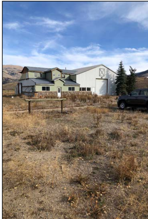
Photo 2 – remaining site structures will be removed during mining.
