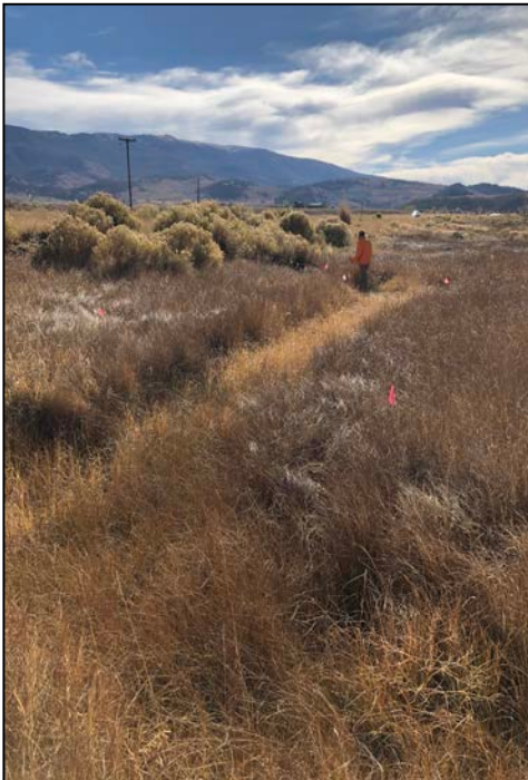
Photo 4 – small channel excavated to guide flow from culverts south toward drainage easement.
