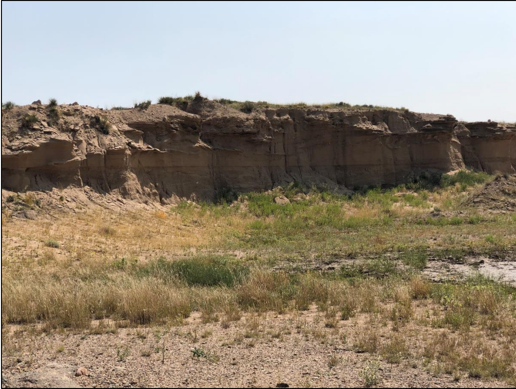
Photo 3. Closer view of eastern pit wall, approximately 15 feet in height with near vertical slopes. Note grasses volunteering across pit floor.
