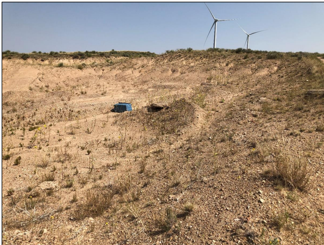
Photo 4. View looking north across eastern pit wall located north of access road which has been graded to 3H:1V or flatter.
