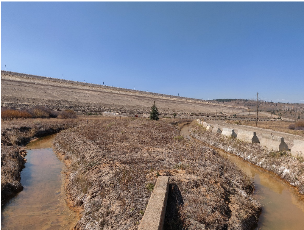
View of the seep collection canals at the Ute Park Pump station looking northwest
