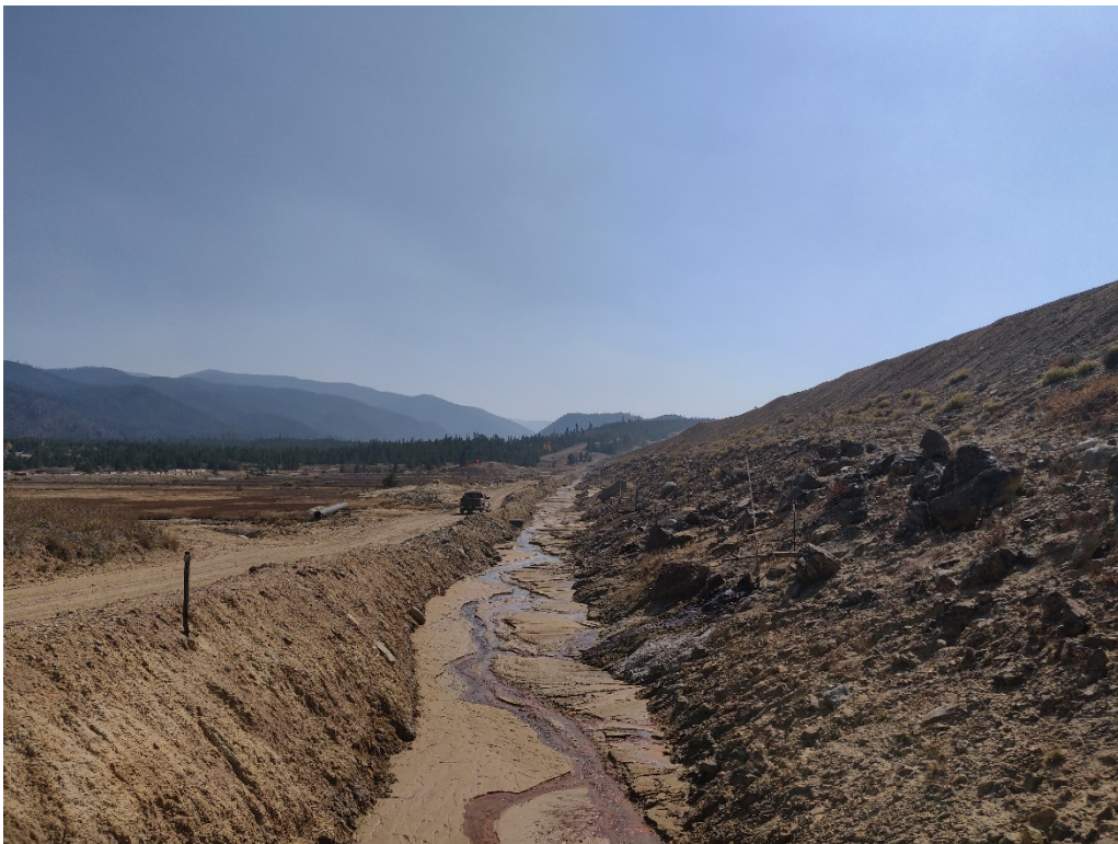
View of the seep collection ditch at the toe of 1-Dam looking south
