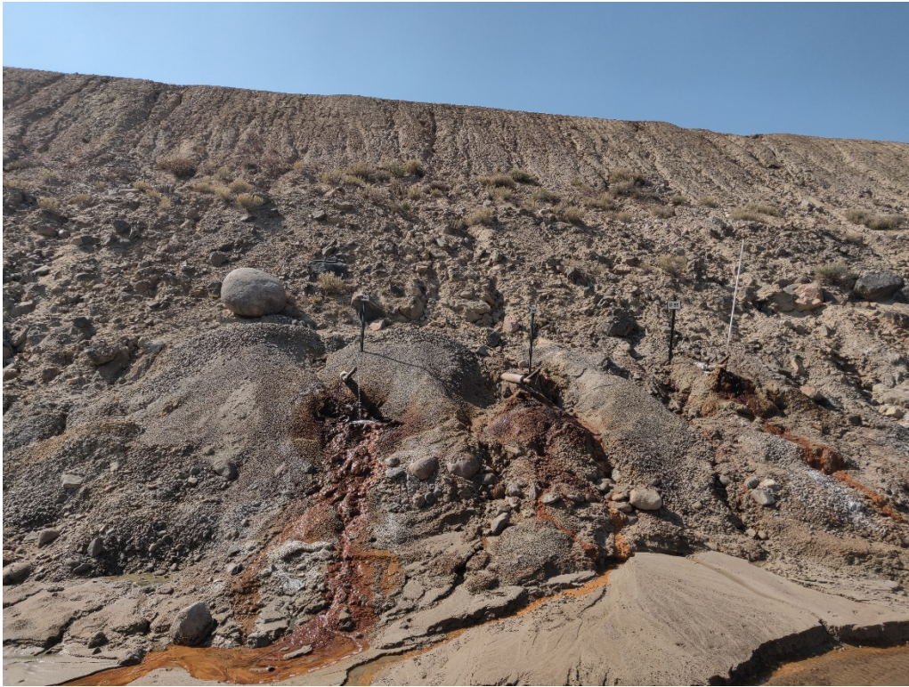
View of typical horizontal drains at the toe of 1-Dam
