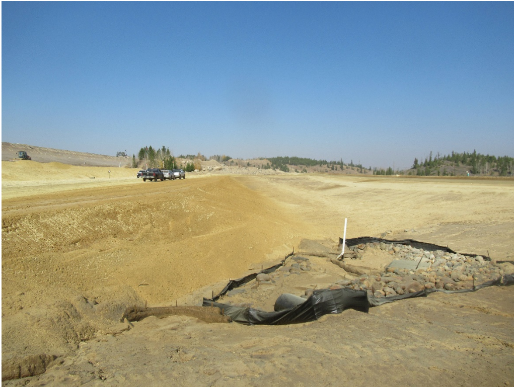
View of the completed middle face of the 3-Dam south area buttress
