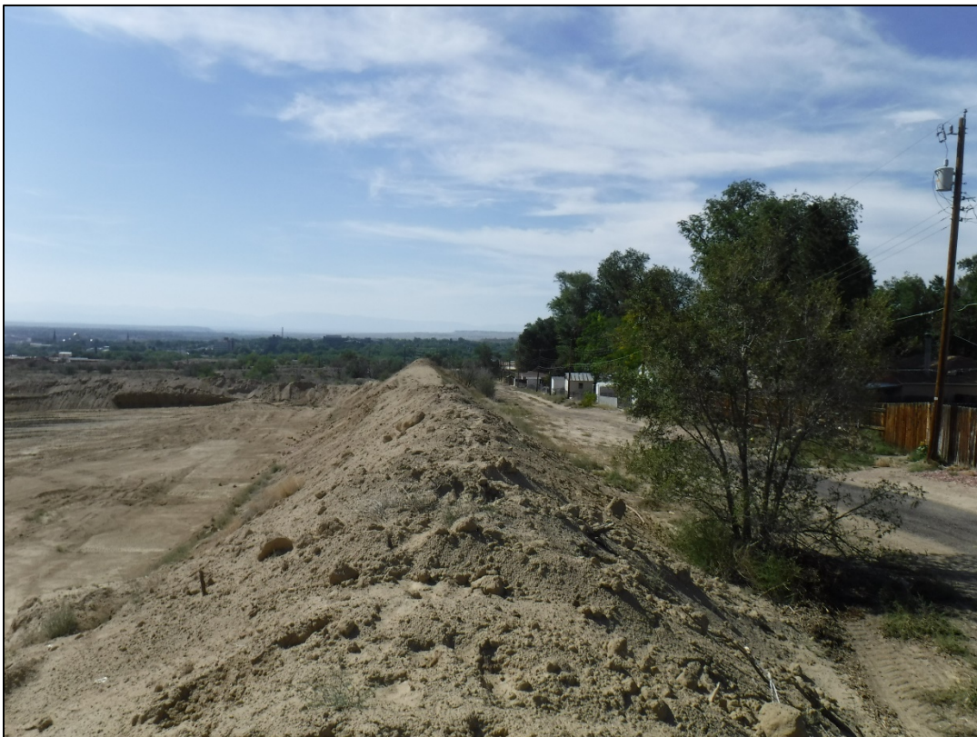
Photo 10: Safety berm adjacent to alley
