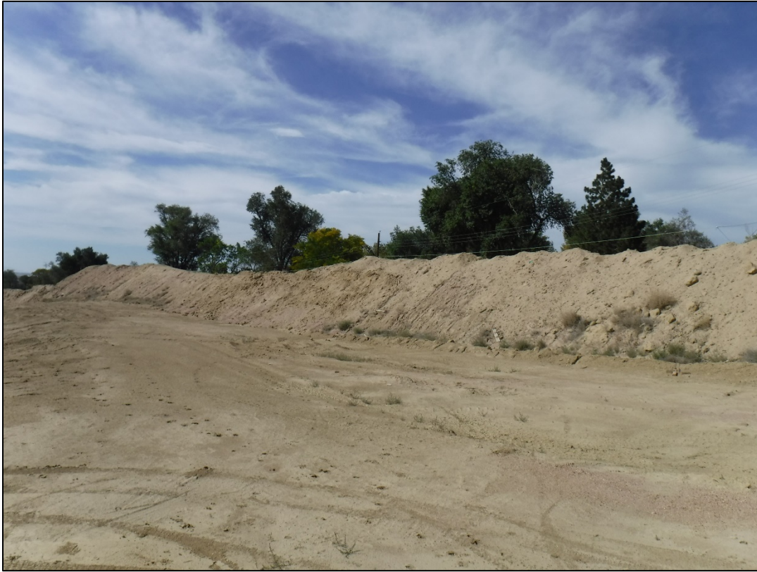
Photo 9: Safety berm adjacent to alley
