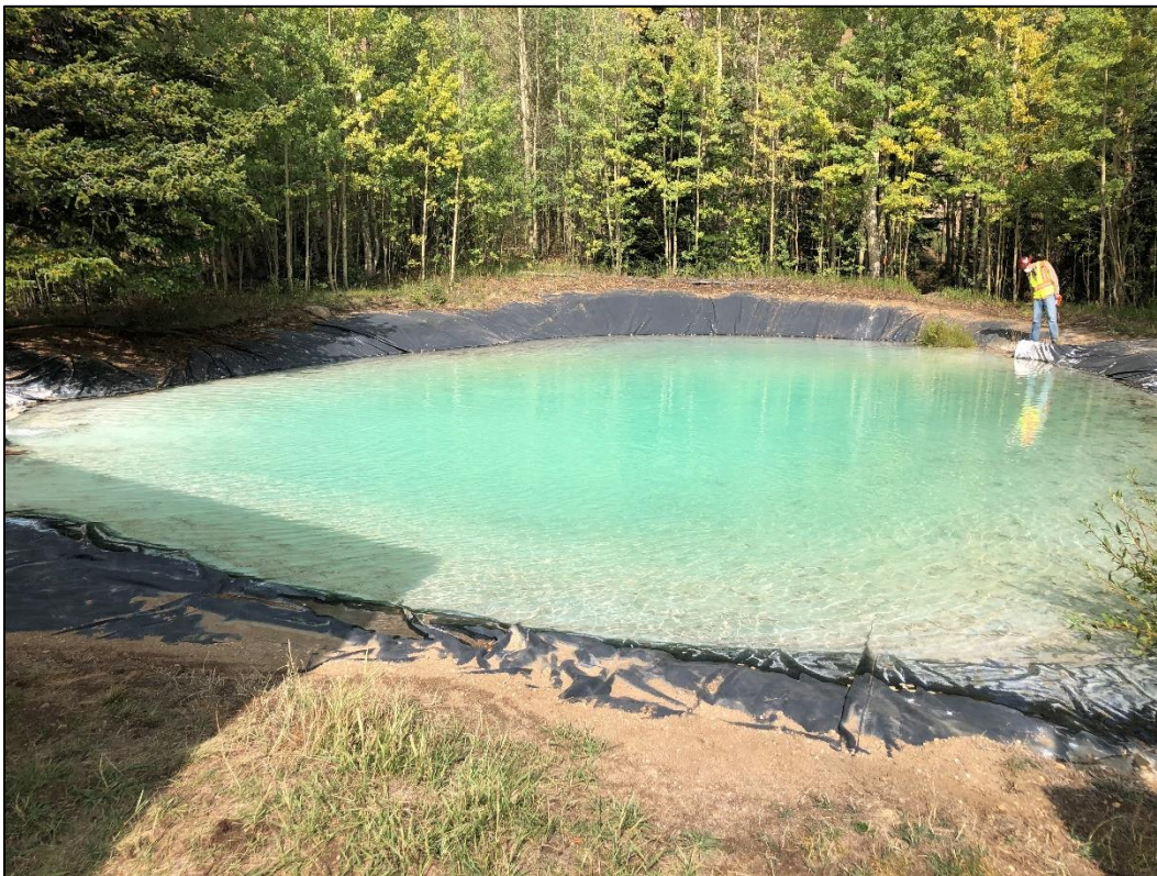
Photo 7. View looking northwest across Pond 1 where Cross Mine water is discharged and treated with 5-15 lbs of lime per day. Water from this pond gravity drains to Pond 2 where it combines with Caribou Mine water prior to being discharged into Coon Track Creek under NPDES permit.
