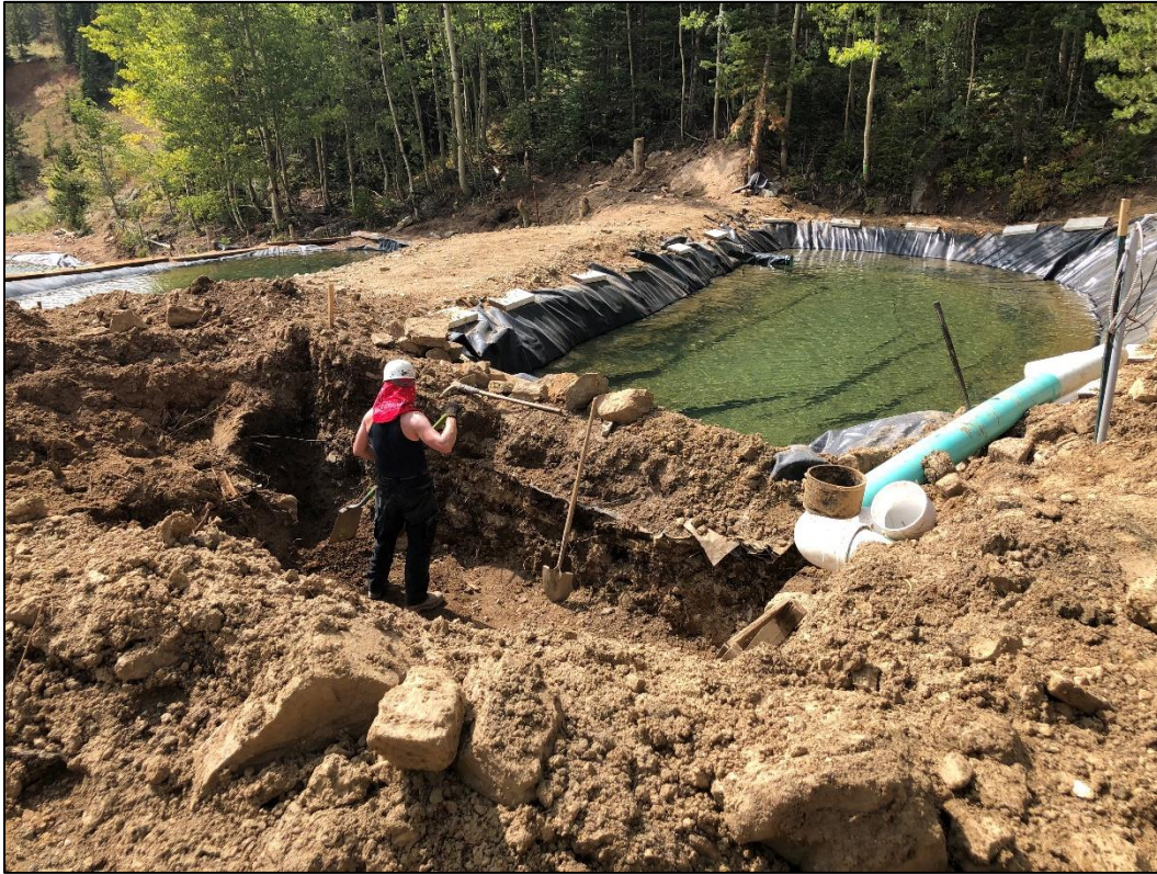
Photo 33. View looking south at settling Pond 3A with new liner installed as proposed in TR-8. Trench was being dug east of Pond 3A (in foreground) for new lime feed and control building.
