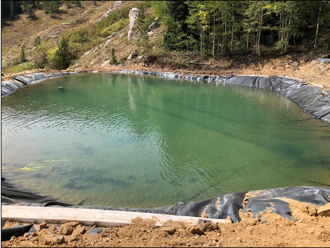
Photo 41. View looking west across settling Pond 3C which was expanded and the liner replaced as proposed in TR-8. This is the largest of the three settling ponds.
