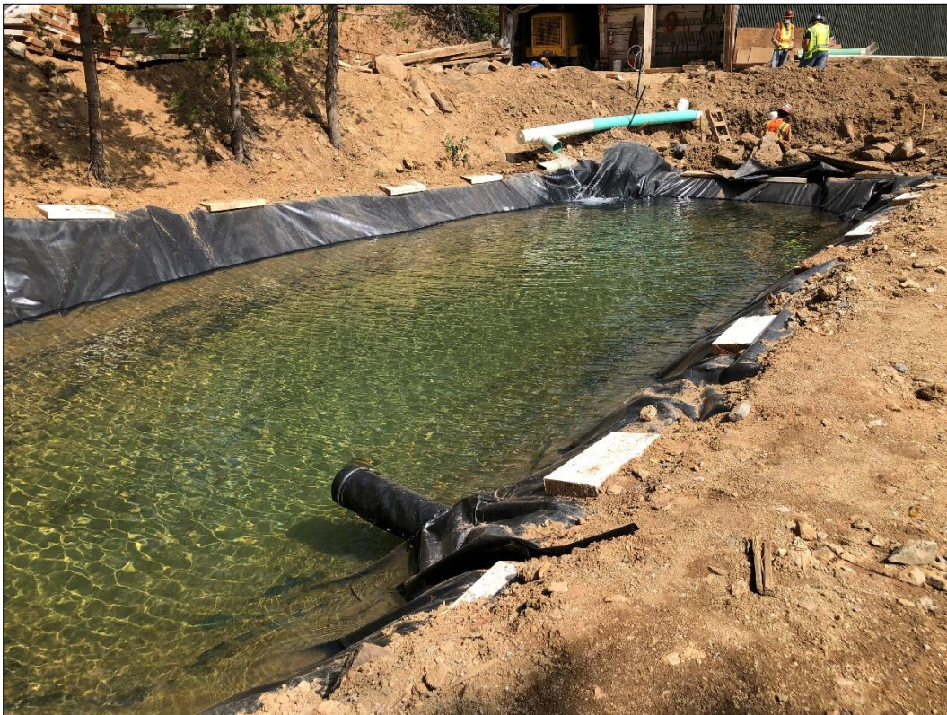
Photo 34. View looking northeast across settling Pond 3A with new liner installed as proposed in TR-8. Note inlet pipe from Caribou Mine at northeastern corner of pond (in background) and outlet pipe to Pond 3B at southwestern corner (in foreground).
