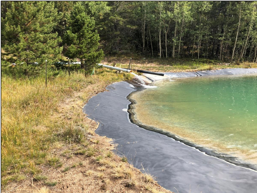
Photo 12. View looking northeast along northwestern edge of Pond 2, showing Cross Mine pipeline (white) and Caribou Mine pipeline (black) discharging into pond.
