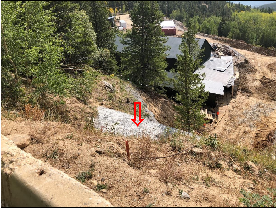
Photo 27. View looking southeast from Caribou Road across slope above Idaho Tunnel portal where small “glory hole” created by tunnel collapse (location indicated) has been stabilized with pervious cellular concrete per TR-5. Majority of new portal area and disturbed slope above is located outside of approved permit boundary.
