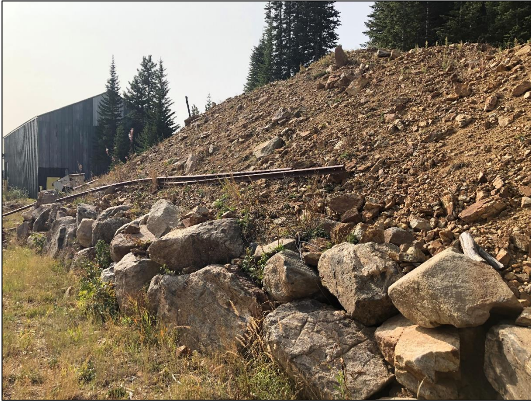
Photo 5. View looking southeast at waste rock from development of new Cross Mine Decline portal temporarily stored near excavation area per AM-1.
