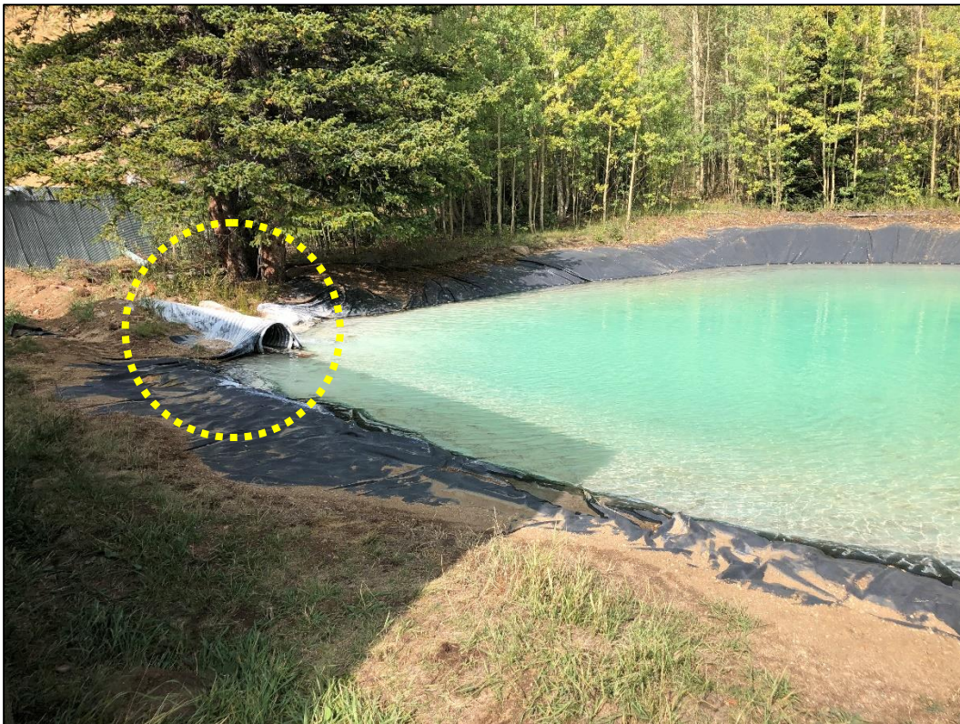
Photo 6. View looking west across southwestern portion of Pond 1 where Cross Mine water is discharged (inlet pipe circled) and treated with 5-15 lbs of lime per day. Operator has plans to add automatic lime feed system in near future.
