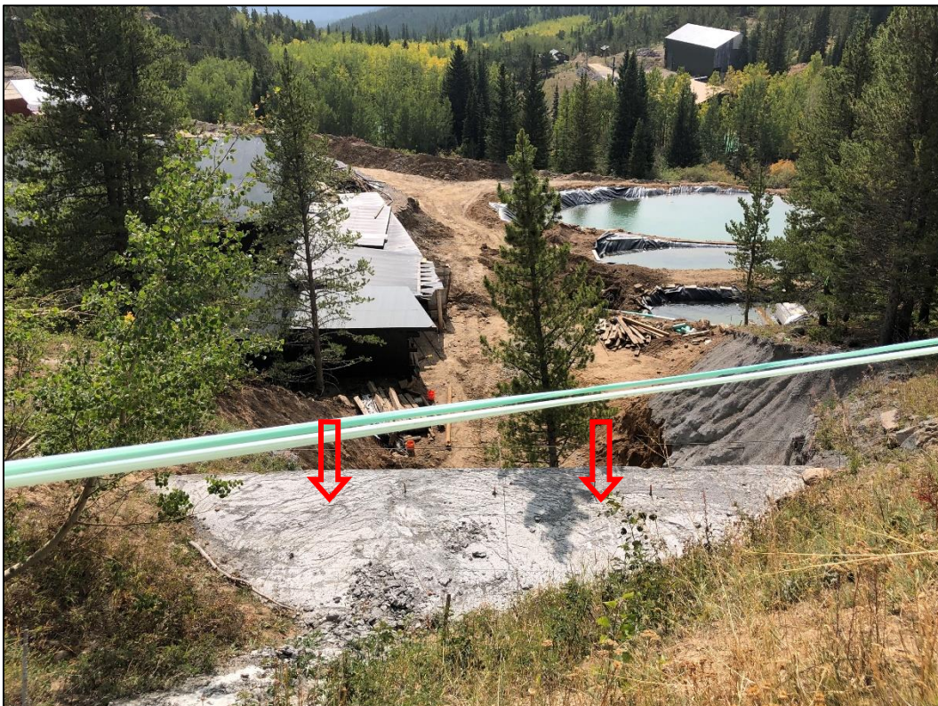
Photo 28. Closer view of slope above Idaho Tunnel portal where small “glory hole” created by tunnel collapse (location indicated) has been stabilized with pervious cellular concrete per TR-5.
