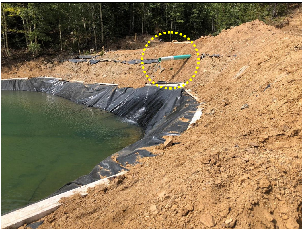
Photo 40. View looking northwest across northeastern corner of settling Pond 3C which was expanded and the liner replaced as proposed in TR-8. Note inlet pipe from Pond 3B (circled) discharging into pond.
