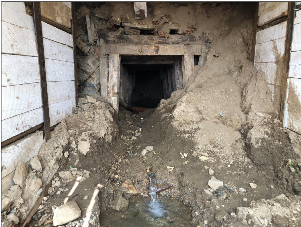
Photo 32. Closer view of Idaho Tunnel portal which requires further rehabilitation for safe entry. Note mine water draining from portal (bottom, center of photo).
