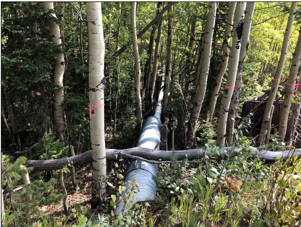
Photo 8. View looking east at drainage pipe which conveys treated Cross Mine water from Pond 1 to Pond 2 where it combines with Caribou Mine water prior to being discharged into Coon Track Creek under NPDES permit.
