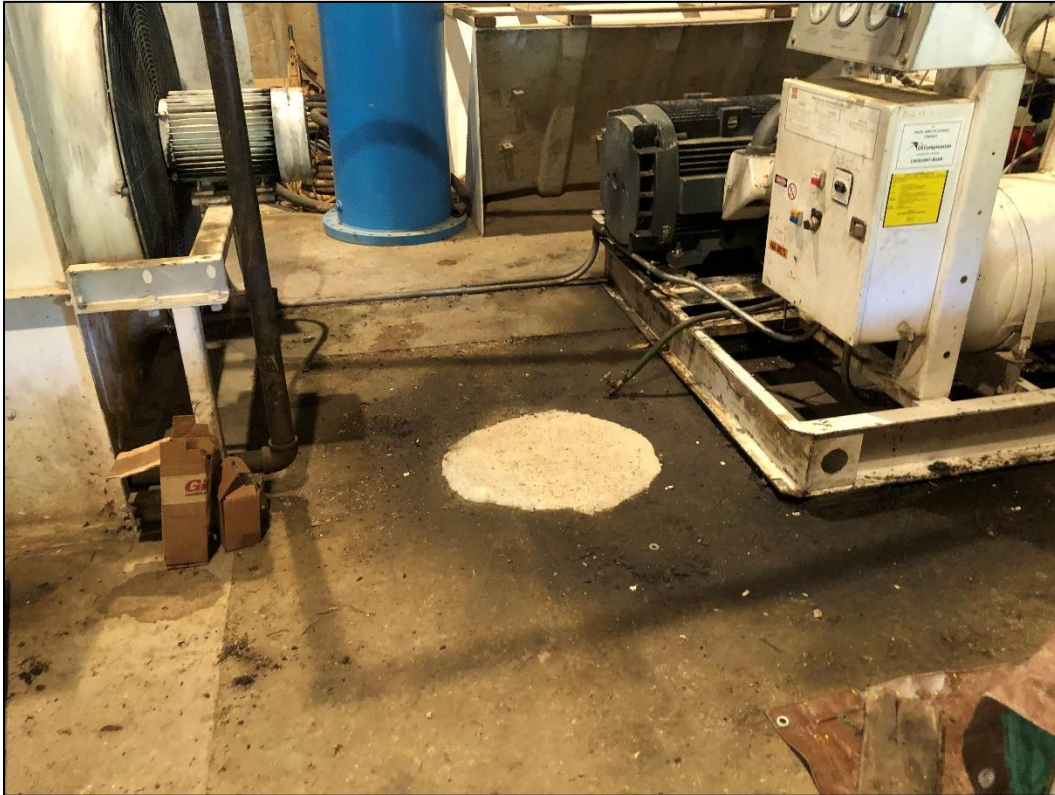
Photo 3. View of floor inside northern end of Cross ore warehouse where operator has permanently sealed floor drain with concrete per TR-6.
