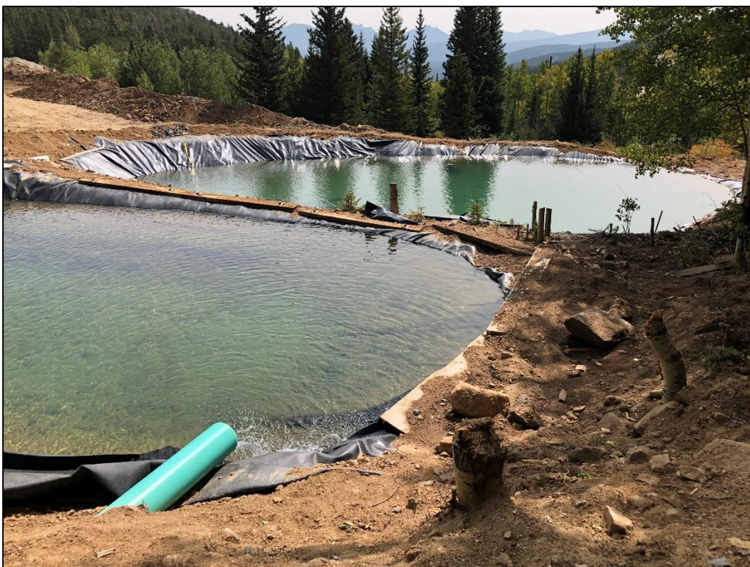
Photo 36. View looking southeast across settling Ponds 3B and 3C with new liners installed as proposed in TR-8. Inlet pipe from Pond 3A located at northwestern corner of Pond 3B (in foreground).
