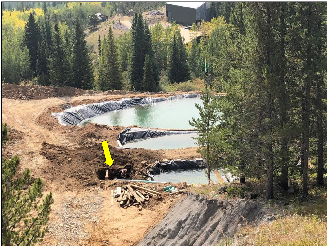
Photo 30. View looking southeast from Caribou Road showing settlings Ponds 3A-C in which Caribou Mine water flows prior to discharging to Pond 2 below. New pond liners have been installed as proposed in TR-8. Trench being dug east of Pond 3A (indicated) is for new lime feed and control building.
