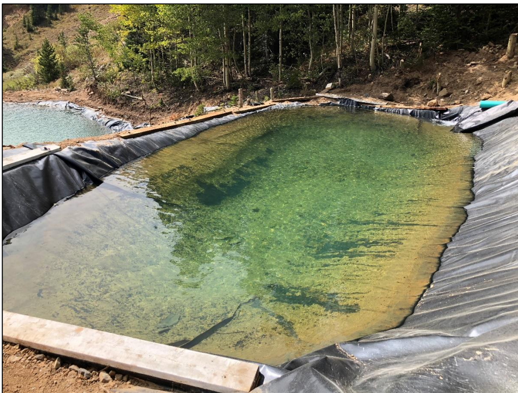
Photo 39. View looking southwest across settling Pond 3B with new liner installed as proposed in TR-8. Note inlet pipe from Pond 3A at northwestern corner of pond (in background, right). Outlet pipe at southeastern corner of pond (not visible in photo).
