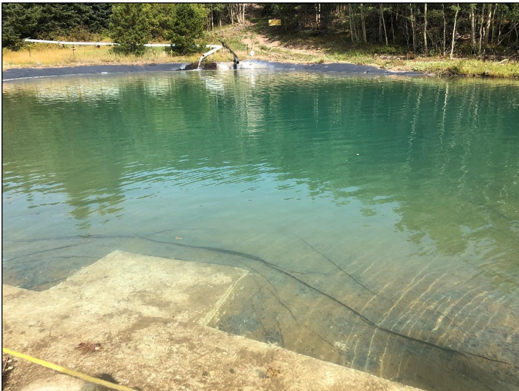
Photo 16. View looking northwest across Pond 2 in which treated Cross Mine water and untreated Caribou Mine water is combined prior to being discharged to Coon Track Creek under NPDES permit.
