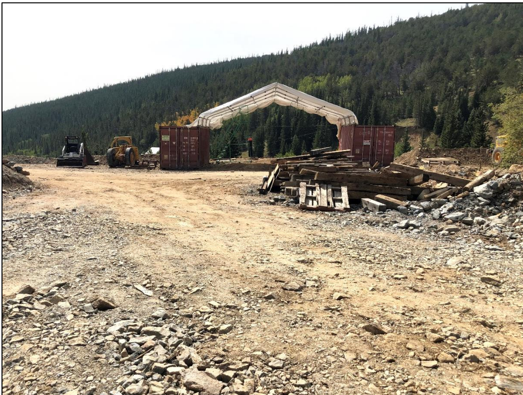
Photo 44. View looking west showing new storage facility constructed in Caribou Mine area with fabric roof installed across two conex containers. This is not considered a permanent structure.
