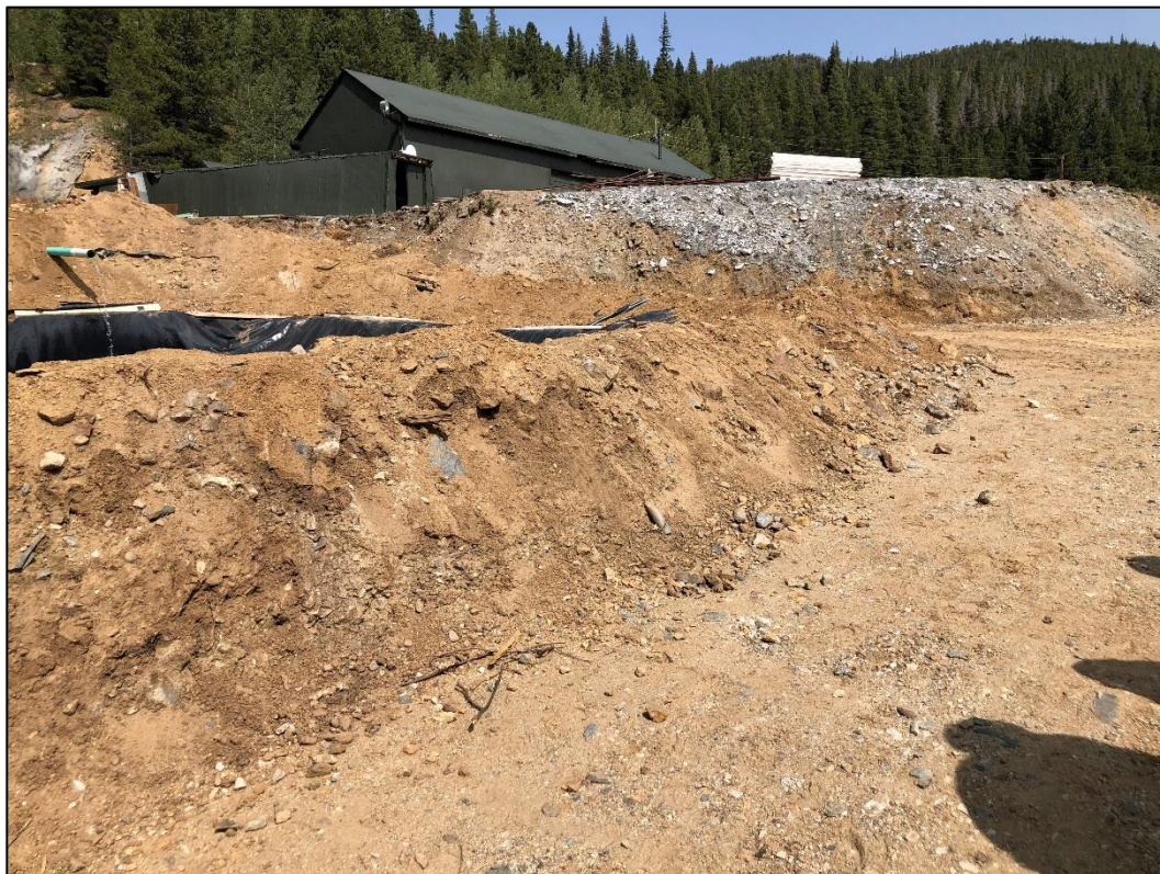
Photo 42. View looking northeast at earthen embankment constructed below settling Pond 3C (at left).
