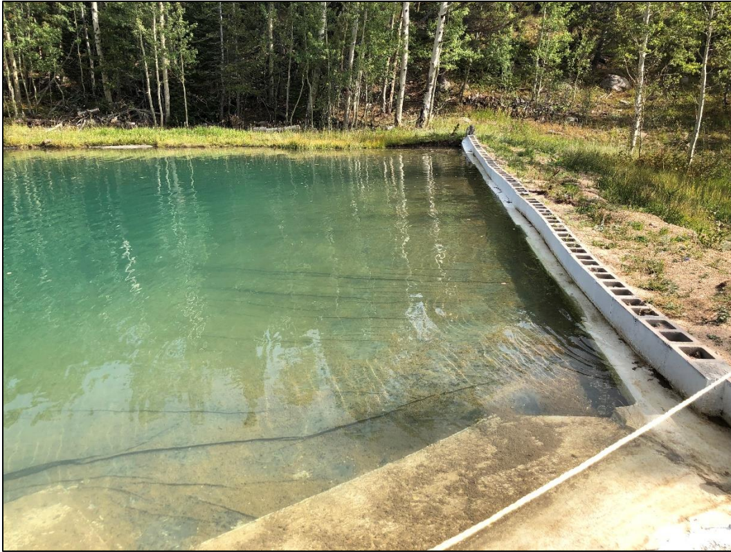
Photo 15. View looking northeast across southeastern edge of Pond 2 in which treated Cross Mine water and untreated Caribou Mine water is combined prior to being discharged to Coon Track Creek under NPDES permit.
