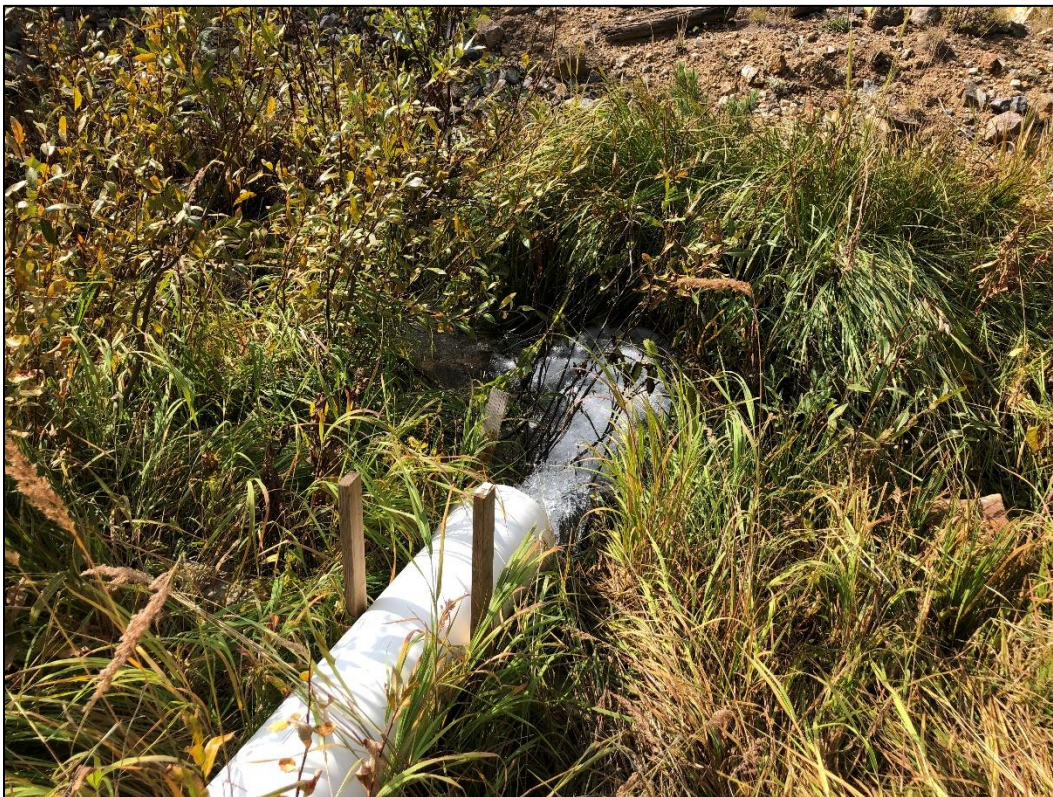
Photo 21. View of discharge point where Pond 2 water is discharged into Coon Track Creek under NPDES permit. Pond 2 discharge rate was 106.5 gal/min during inspection.
