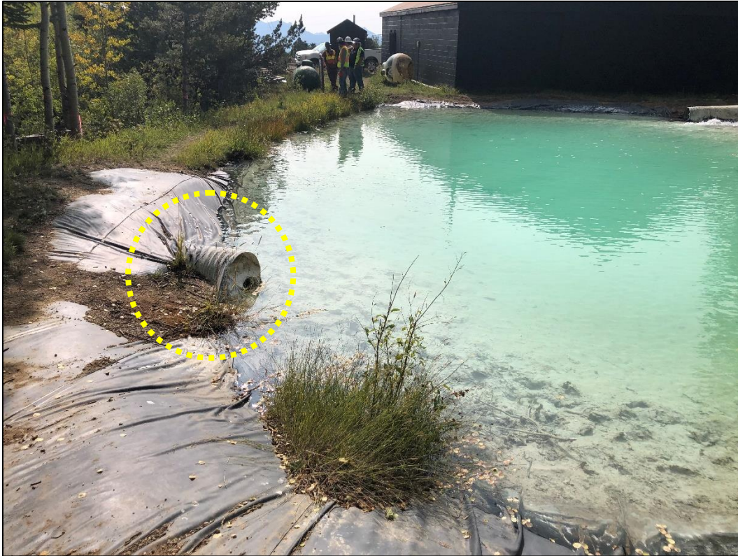
Photo 9. View looking southeast across northeastern corner of Pond 1, showing outlet pipe at left (circled). Operator should remove any sediment and vegetation from pond liner to maintain freeboard and protect liner integrity.
