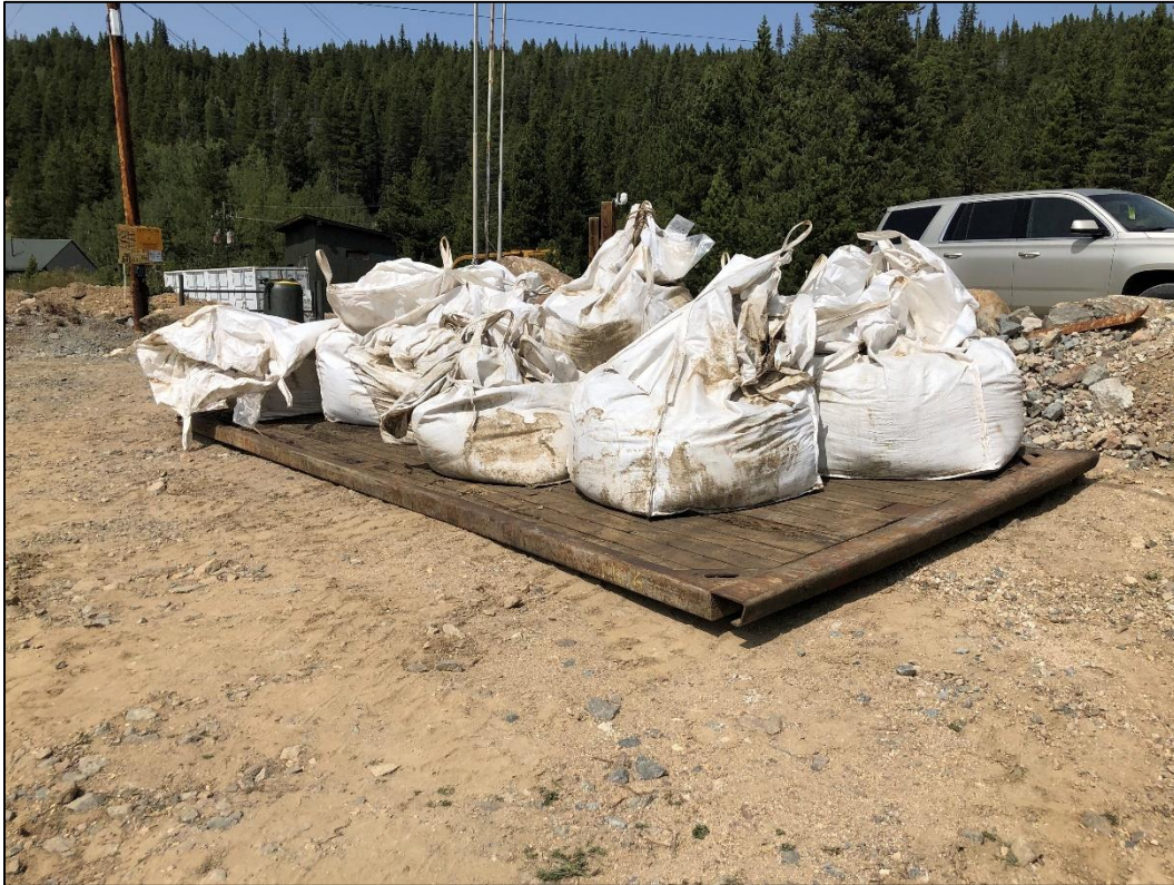
Photo 47. View looking north at nine super sacks filled with sludge removed from settling ponds, currently stored on top of existing waste rock pile in Caribou Mine area. Operator will need to perform additional lab testing on this material to determine an appropriate disposal location.
