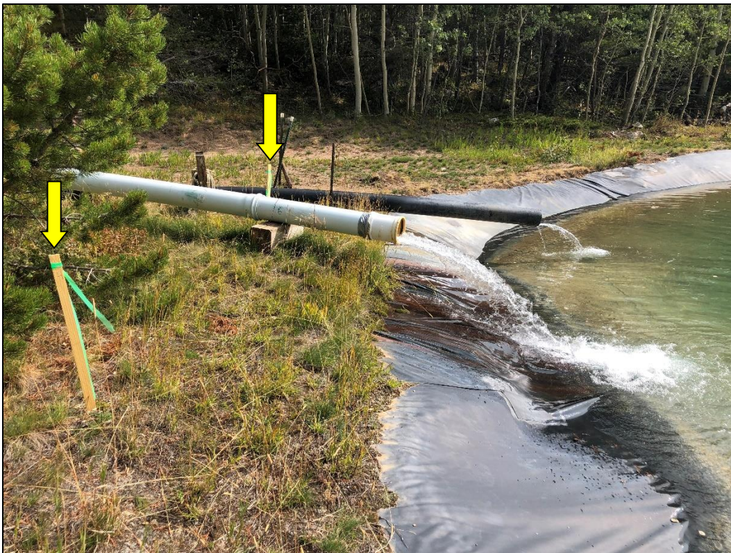
Photo 13. Closer view of northern corner of Pond 2 where Cross Mine pipeline (white) and Caribou Mine pipeline (black) discharge into pond. Laths with green flagging (indicated) mark approved permit boundary. Recent surveying shows portions of Caribou pipeline and northwestern corner of pond are located outside approved boundary.
