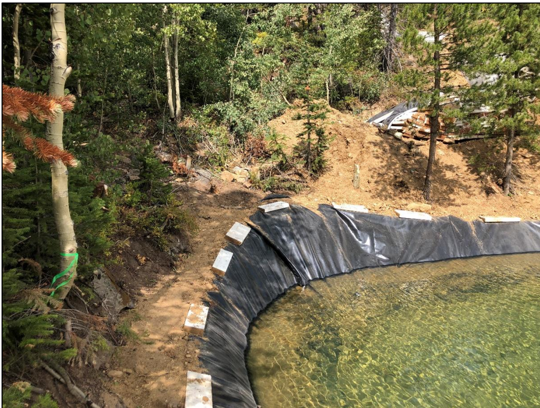
Photo 35. View looking northwest along western edge of settling Pond 3A where vegetation was removed to allow room to install new pond liner. Recent surveying shows a portion of this pond is located outside of approved permit boundary.
