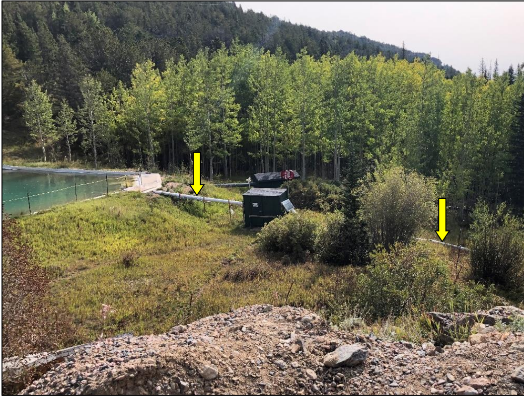
Photo 11. View looking southeast showing discharge pipeline (indicated) from southern corner of Pond 2 to Coon Track Creek where combined mine water is discharged under NPDES permit. Note two discharge sheds located south of pond, newer shed in front.
