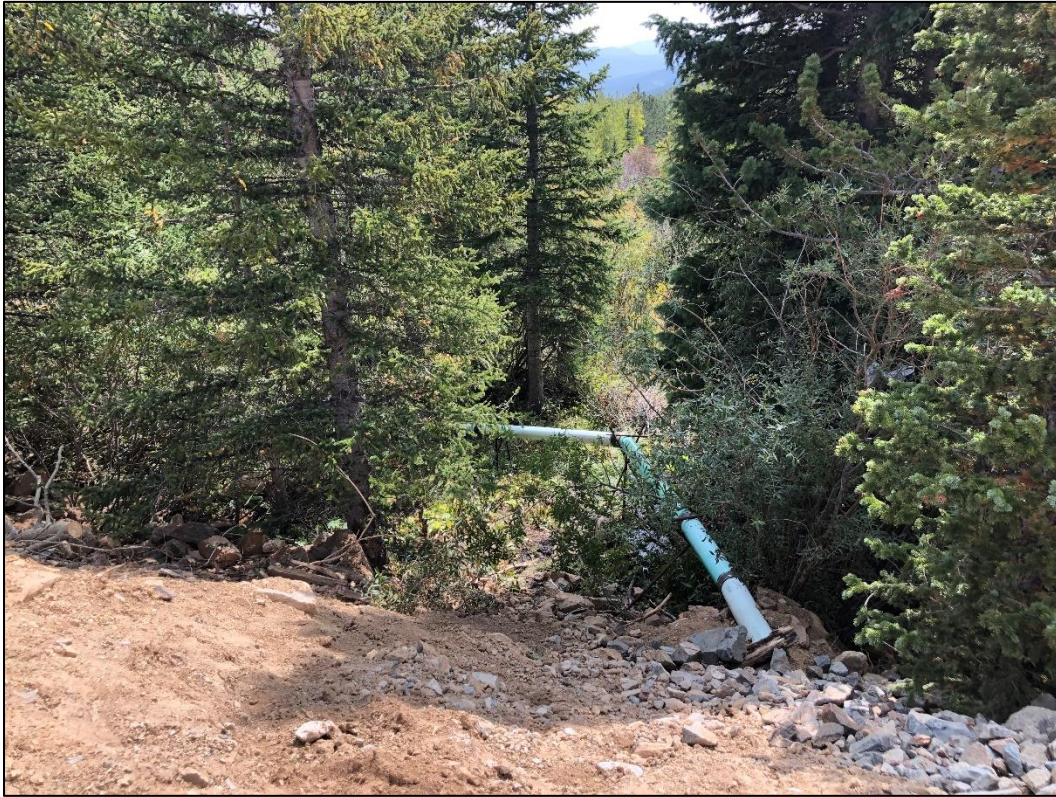
Photo 43. View looking southeast at outlet pipe from settling Pond 3C which conveys Caribou Mine water from settling ponds to Pond 2 below, where water is mixed with treated Cross Mine water prior to being discharged to Coon Track Creek under the NPDES permit.
