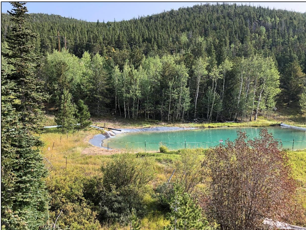
Photo 10. View looking northeast at Pond 2 where treated Cross Mine water and untreated Caribou Mine water is combined prior to being discharged into Coon Track Creek under NPDES permit.
