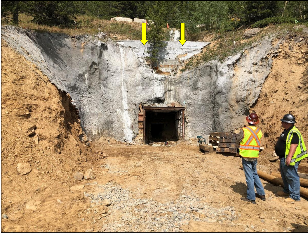
Photo 31. View looking northwest at Idaho Tunnel portal, showing surrounding slope face stabilized with shotcrete and small “glory hole” created by tunnel collapse (location indicated) stabilized with pervious cellular concrete per TR-5. Majority of portal area and disturbed slope above is located outside of approved permit boundary.
