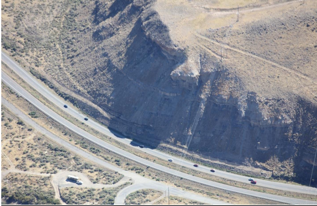
Photo 3: The cliffs at the north end of the Tract 70 Mesa. The photo was taken looking to the east.
