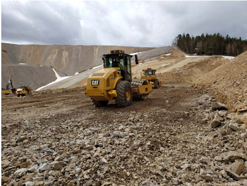
Photo 3: Compaction with 12-ton Vibratory Sheepsfoot Drum Compactor
