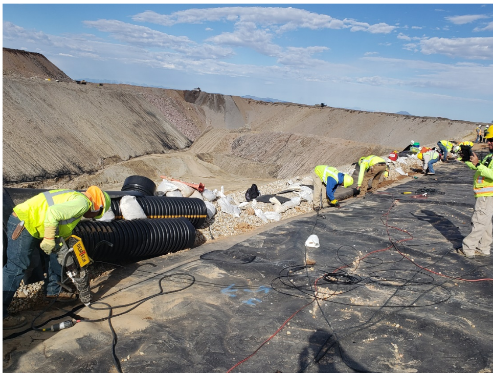
Photo 10 – Extrusion welding of geomembrane (July 7, 2020)
