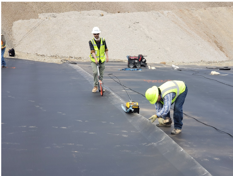
Photo 8 – Fusion welding of geomembrane (June 22, 2020)
