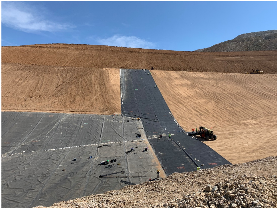
Photo 5 – Deployment of geomembrane (June 15, 2020)
