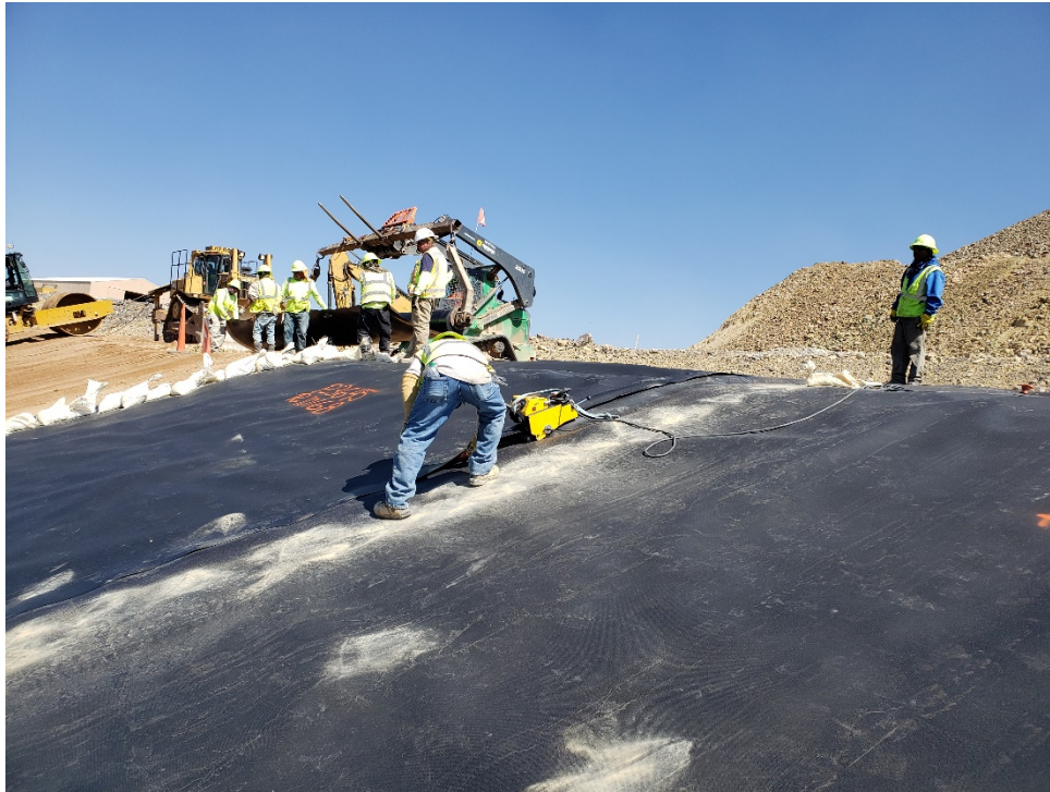
Photo 27 – Fusion welding of geomembrane (August 14, 2020)
