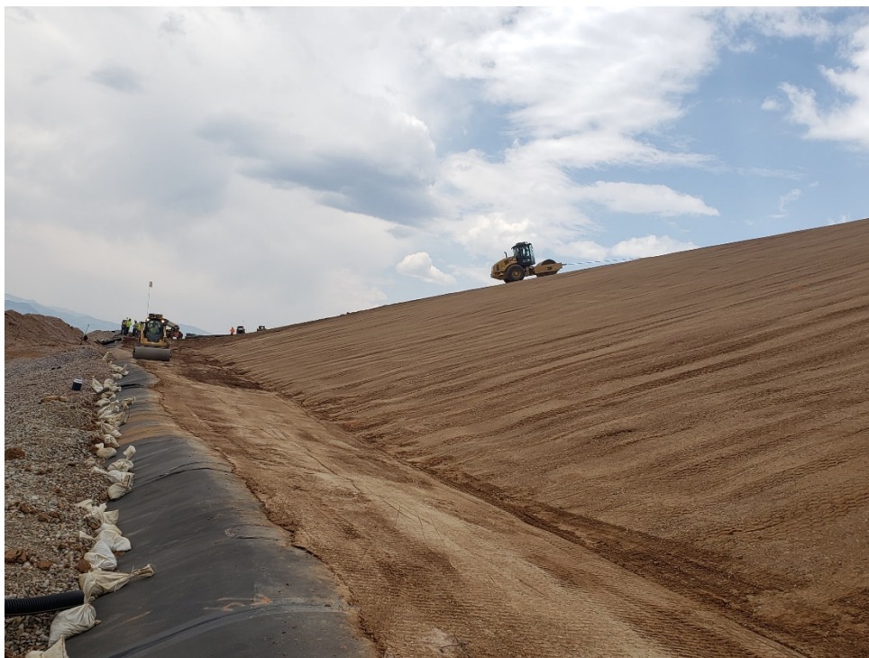
Photo 22 – Compaction of SLF (August 4, 2020)
