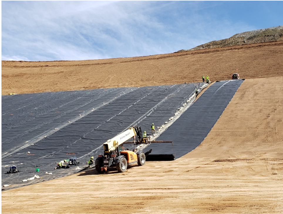
Photo 7 – Deployment of geomembrane (June 20, 2020)
