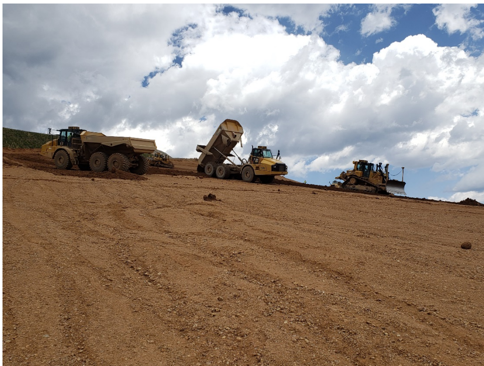
Photo 20 – Placement of SLF (August 1, 2020)
