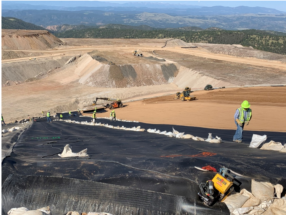
Photo 23 – Deployment of geomembrane (August 6, 2020)
