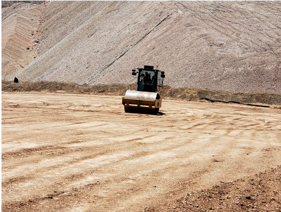
Photo 13 – Compaction of SLF (July 10, 2020)
