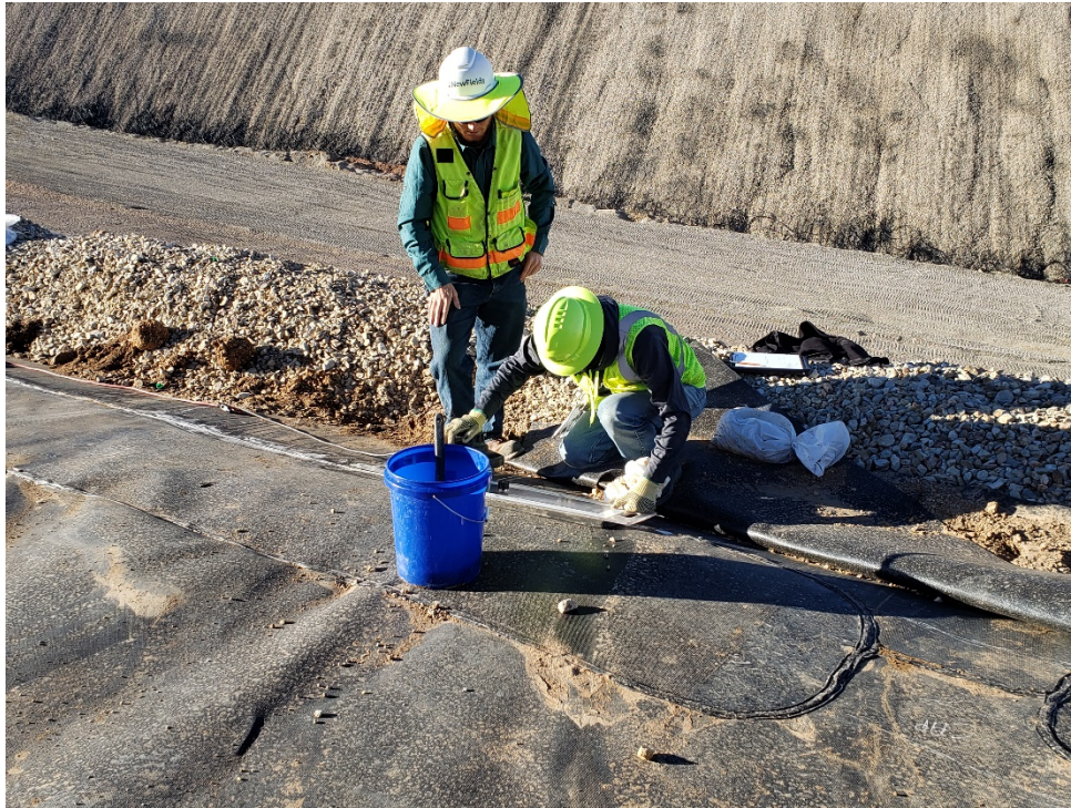
Photo 11 – Vacuum testing an extrusion weld (July 9, 2020)
