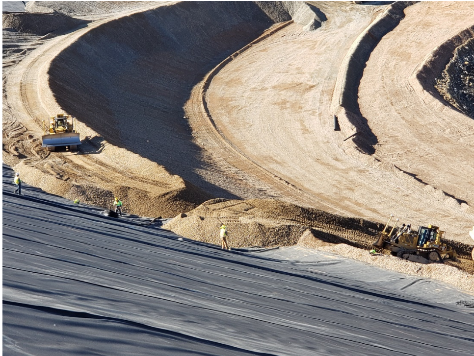
Photo 19 – Building 4' thick DCF haul road (July 31, 2020)
