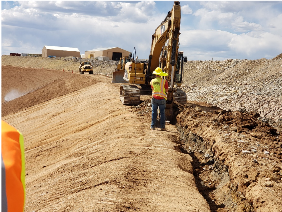
Photo 25 – Anchor trench excavation (August 10, 2020)
