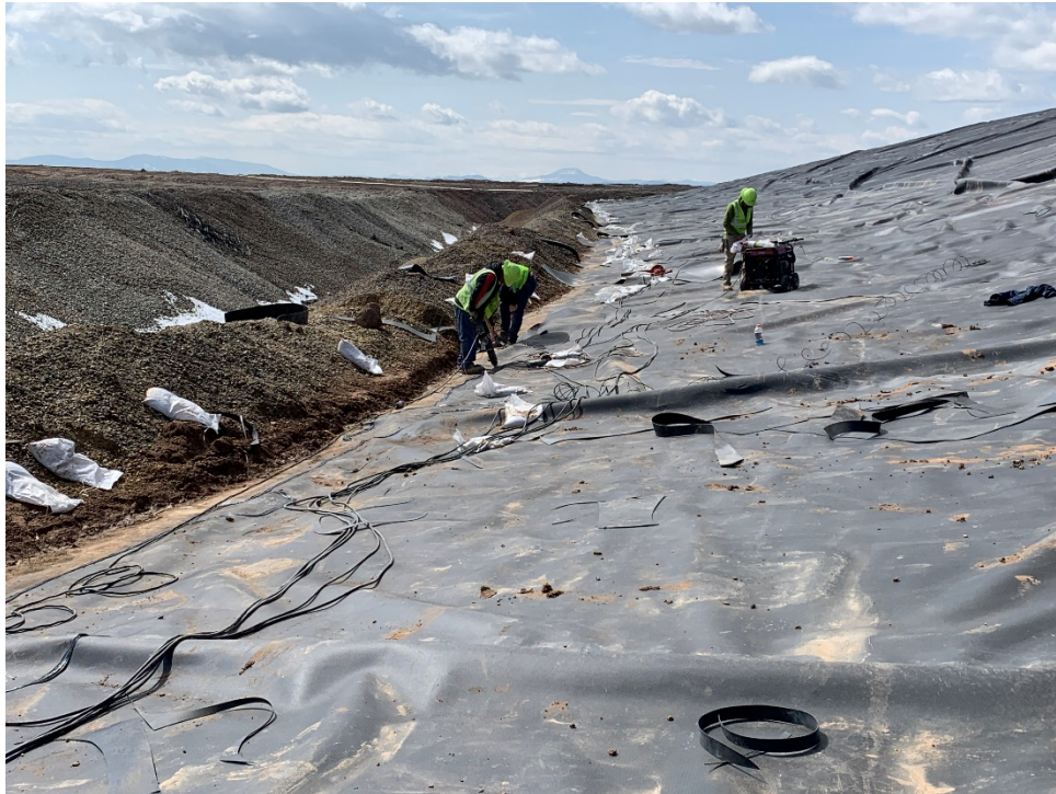
Photo 36 – Extrusion welding of geomembrane (September 11, 2020)
