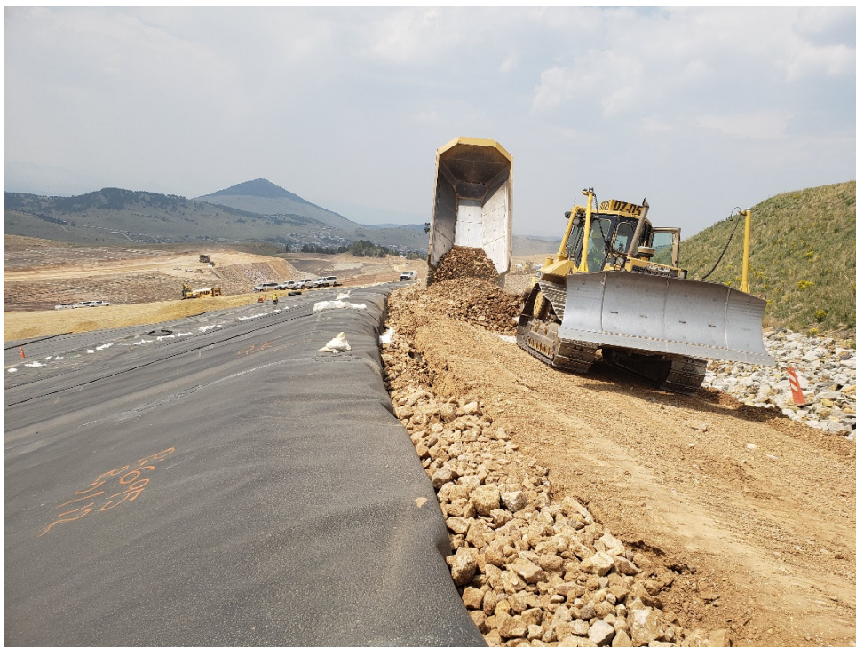
Photo 30 – Backfilling permanent anchor trench (August 24, 2020)
