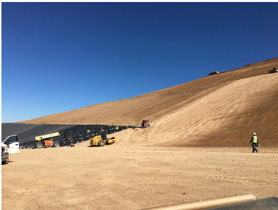
Photo 4 – SLF compaction (June 12, 2020)
