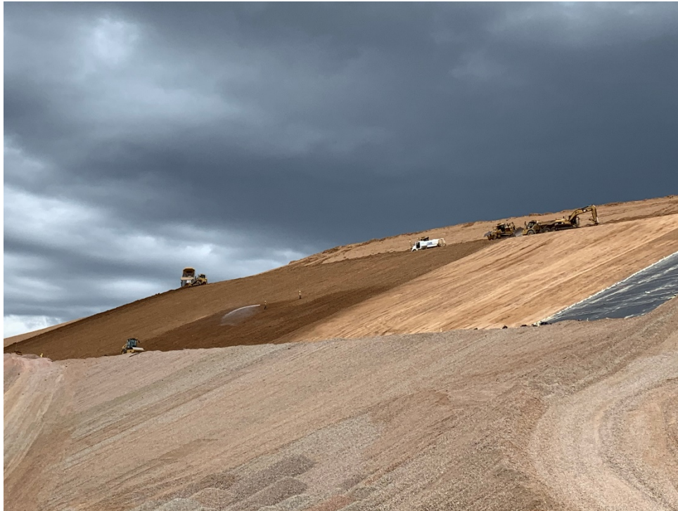
Photo 17 – Moisture conditioning SLF (July 24, 2020)
