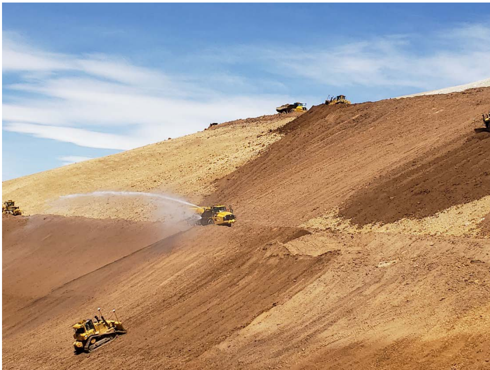
Photo 2 –Spreading and moisture conditioning SLF (May 18, 2020)
