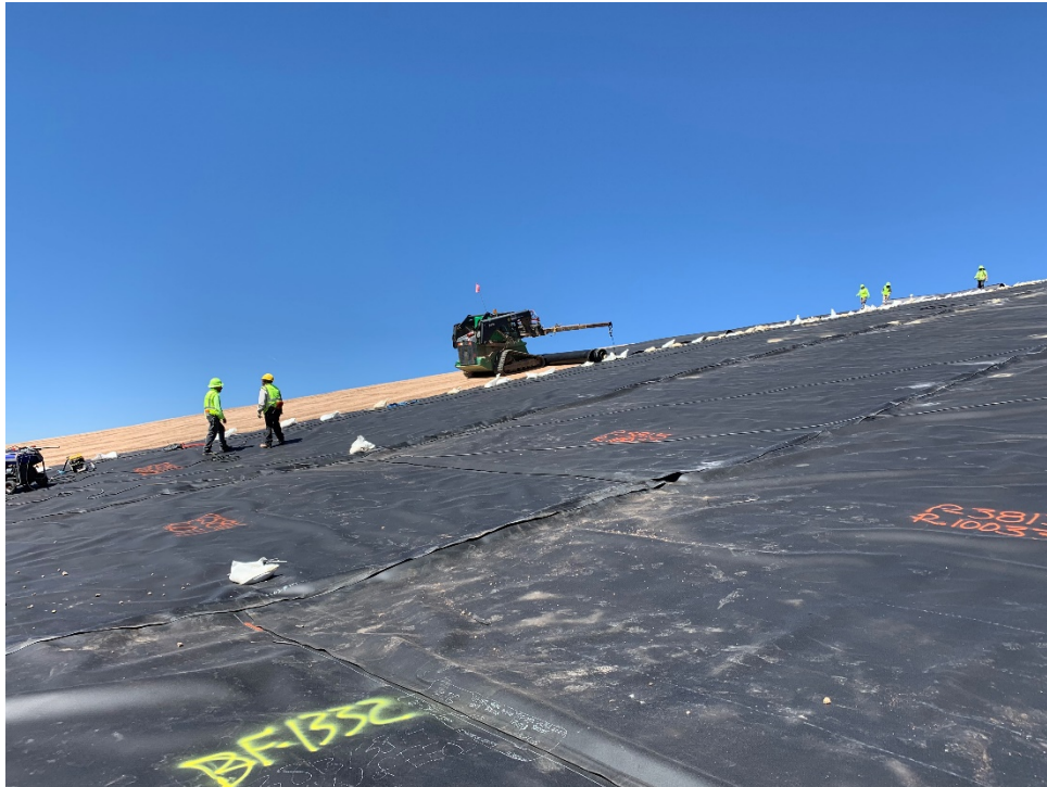
Photo 34 – Deployment of geomembrane (September 3, 2020)
