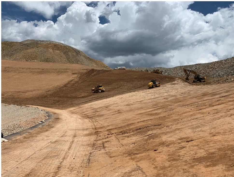
Photo 14 – Spreading of SLF (July 14, 2020)
