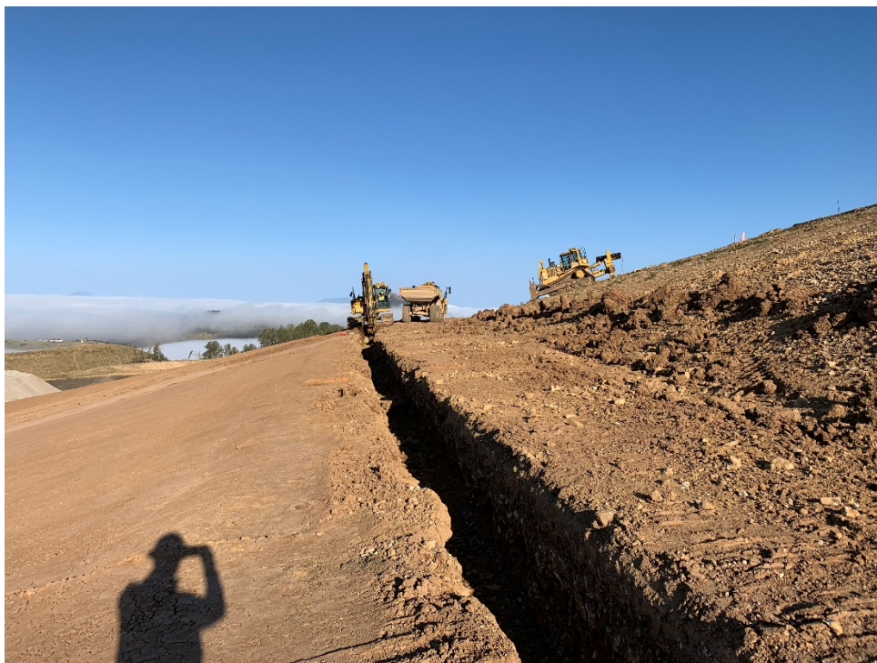
Photo 32 – Anchor trench excavation (August 31, 2020)
