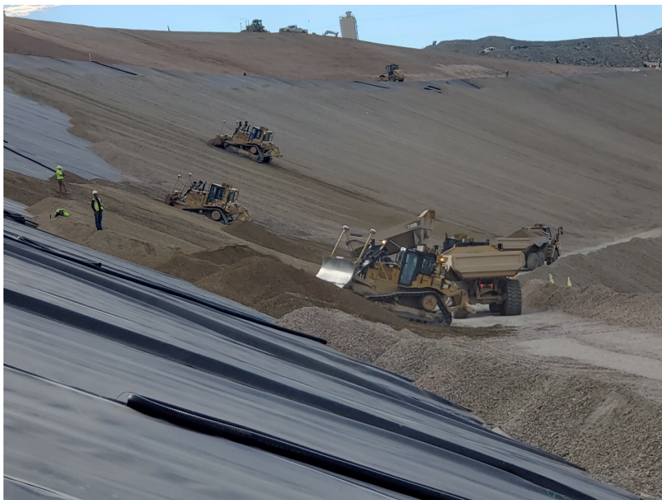
Photo 26 – Spreading of DCF (August 11, 2020)
