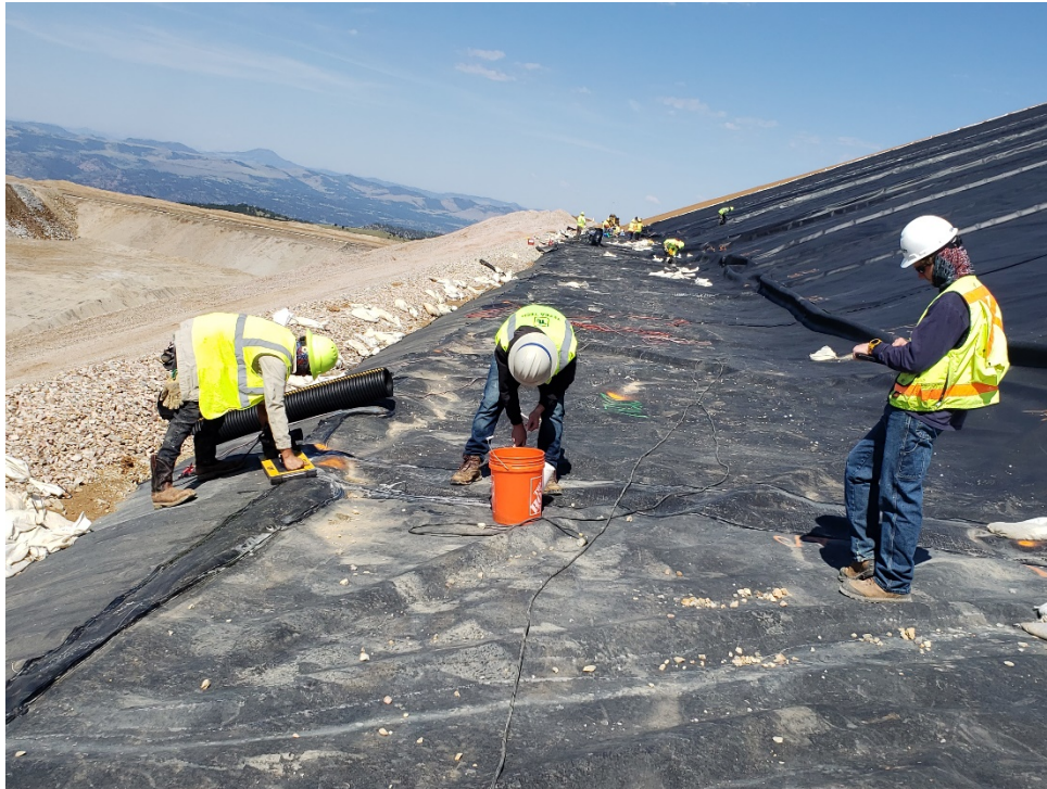
Photo 21 – Vacuum testing an extrusion weld (August 3, 2020)
