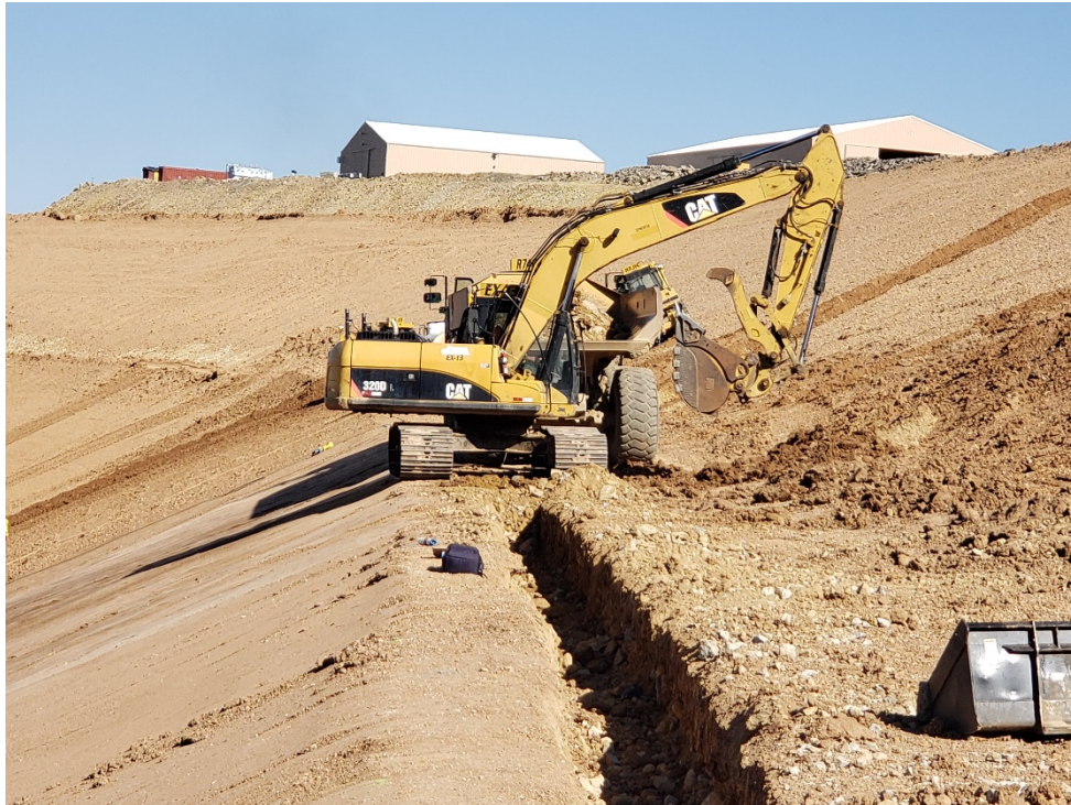
Photo 15 – Anchor trench excavation (July 17, 2020)
