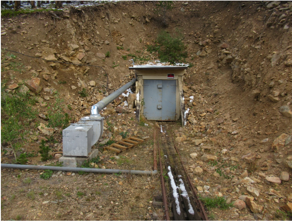
View of the secured portal and mine fan
