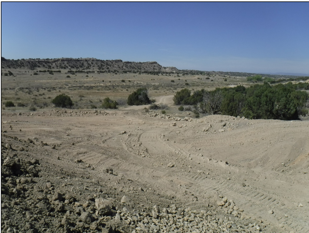
Photo 6: Recently mined area that has been reclaimed to a 3H:1V slope or shallower, looking southwest
