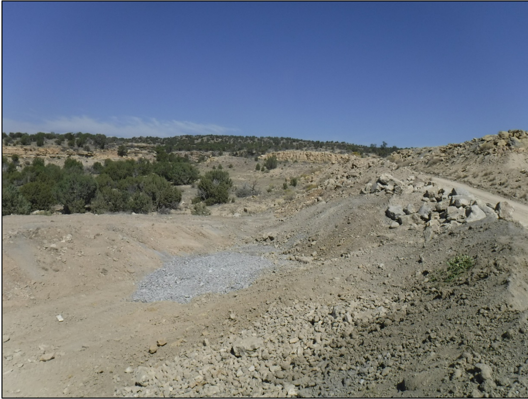
Photo 5: Recently mined area that has been reclaimed to a 3H:1V slope or shallower, looking northeast
