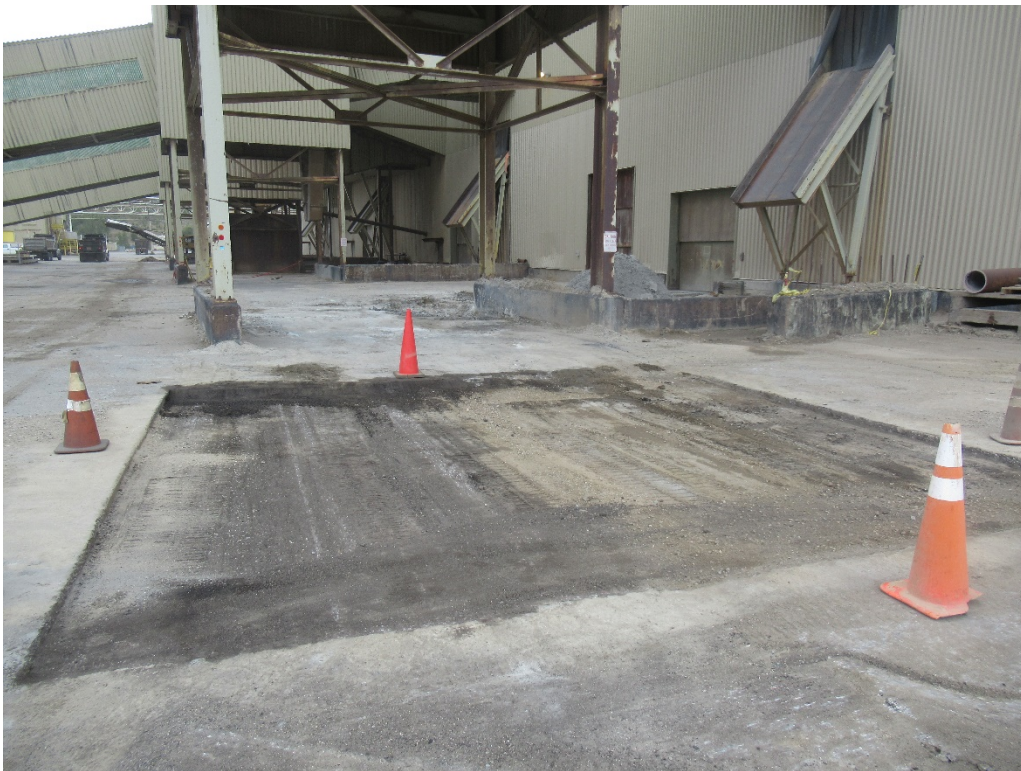
View of fire water repair area located east of hydrant #6
