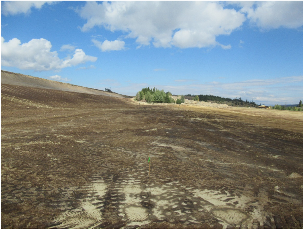
View of the upper face on the south area of 3-Dam, stakes indicate toe of buttress material placement for Phase 2
