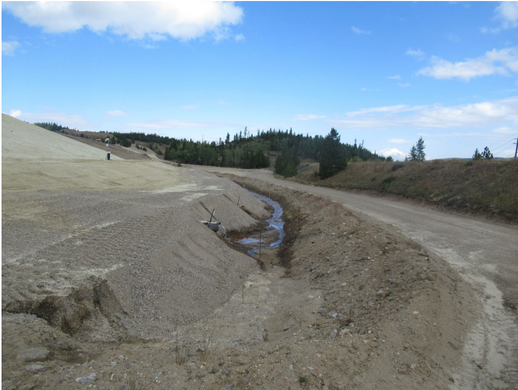
View of the rock fill at the toe of the south area of 3-Dam from the south end looking north
