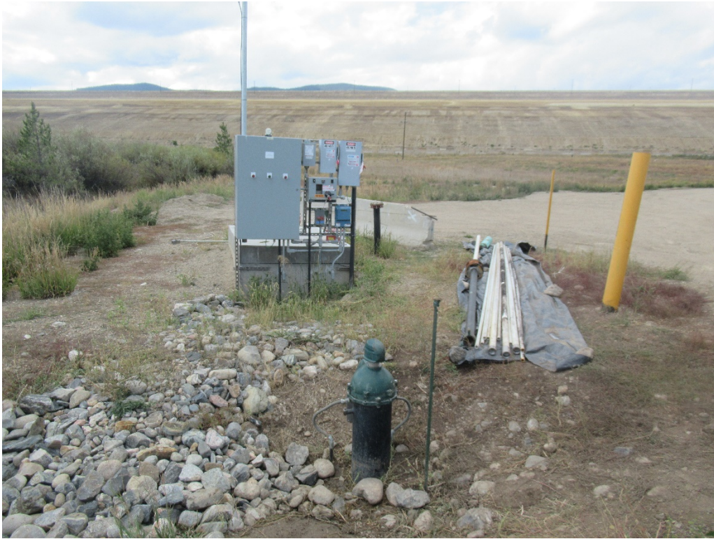
View of MLEX-4 during rehabilitation
