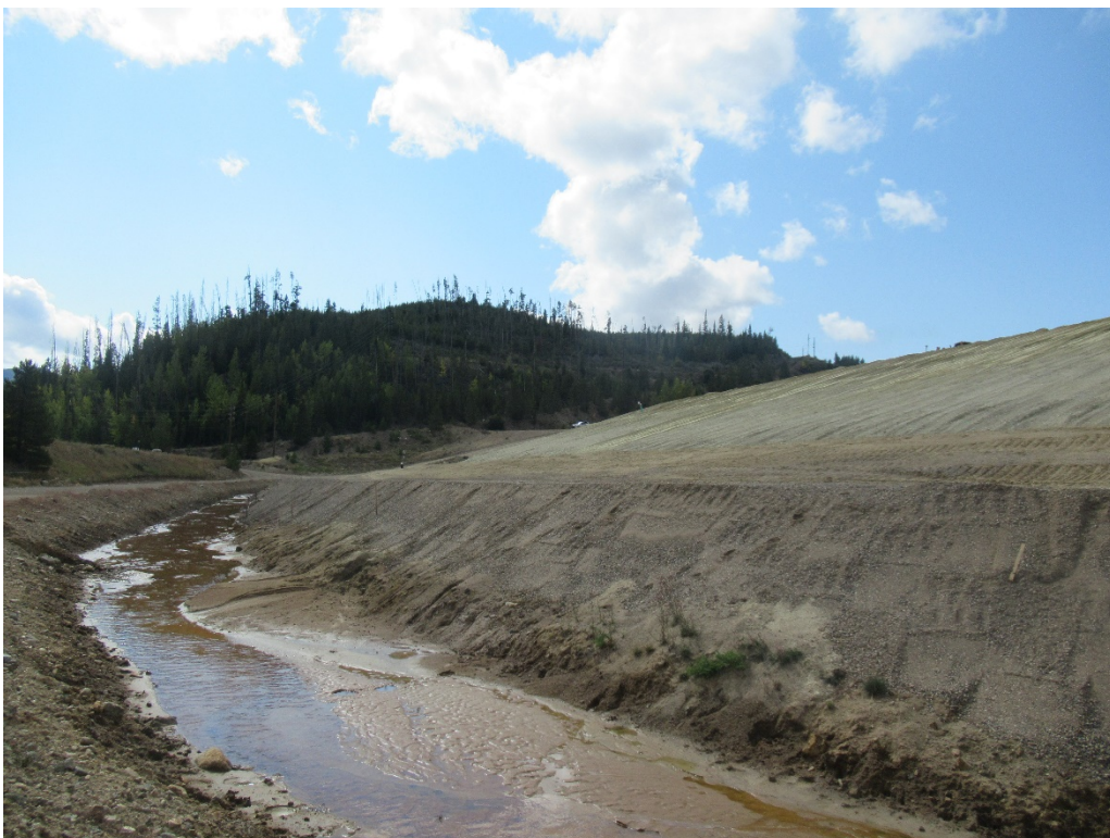
View of the rock fill at the toe of the south area of 3-Dam from the north end looking south
