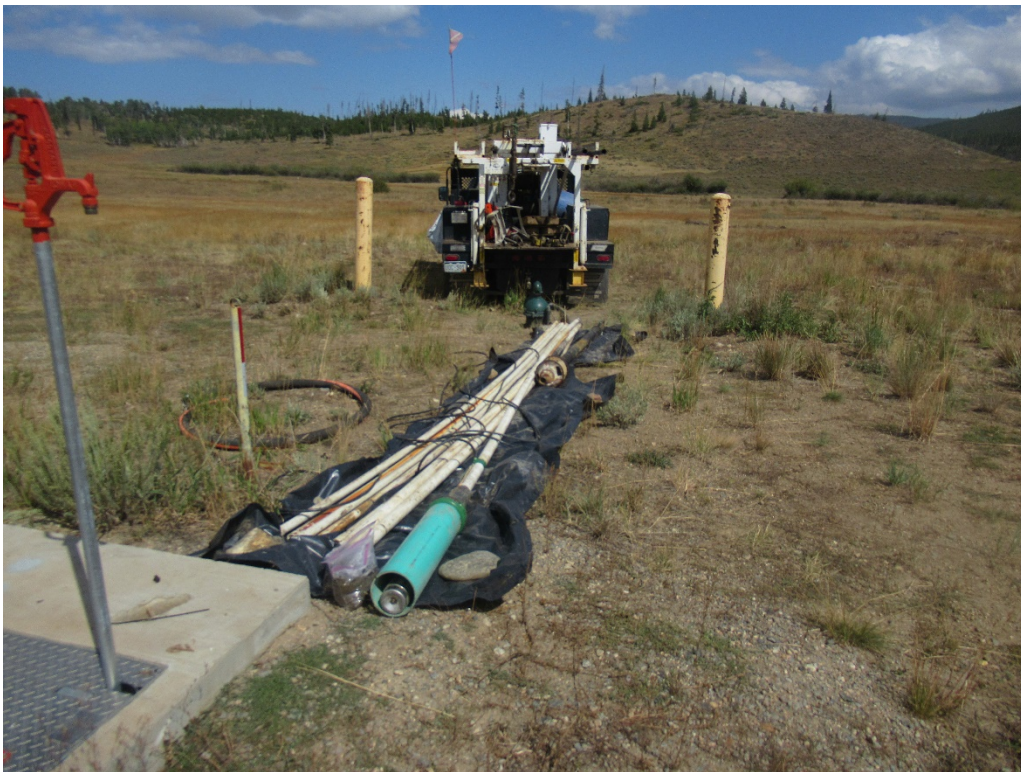
View of MLEX-1 during rehabilitation
