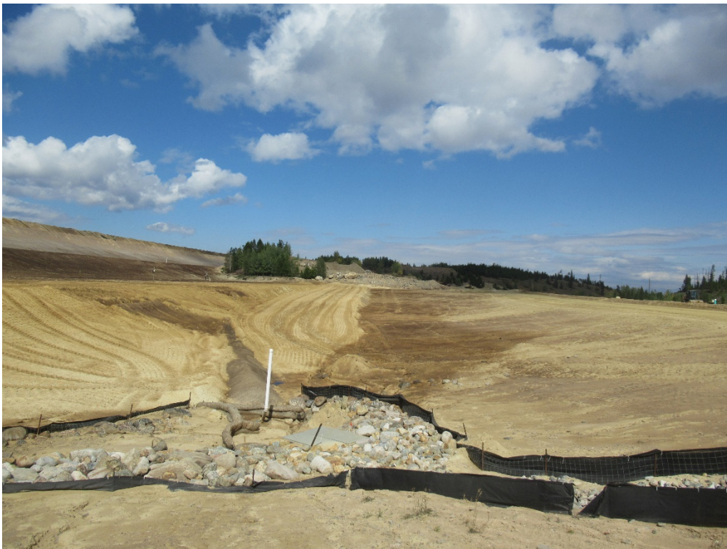
View of the stepback bench on the south area of 3-Dam, filter material placed and covered with buttress material
