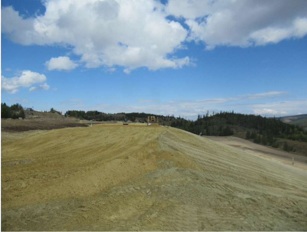
View of the placement and compaction of buttress material on the lower face of the south area of 3-Dam
