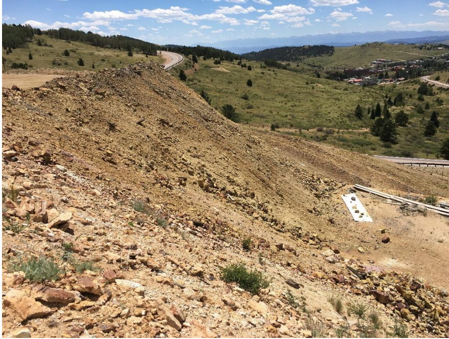
Photo 1: Stormwater controls are adequate, very little erosion from side slope
