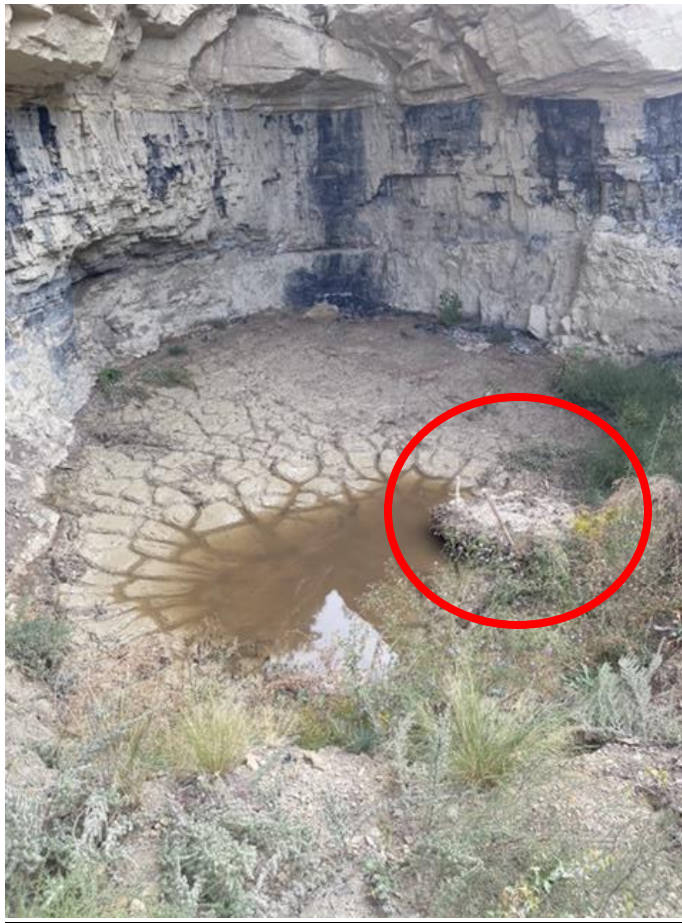
Photo 4: The sump east of the portals bench. The red circle outlines the trash rack that requires cleaning.
