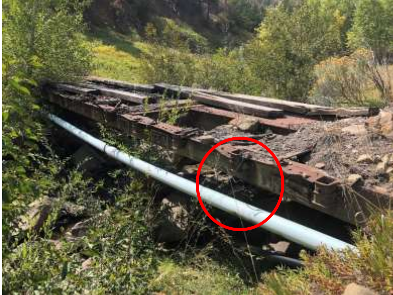
Pipe on bridge across creek (circle around disconnected support)
