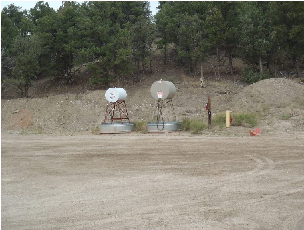
Photo 1. Fuel storage secondary containment. (near shop area).
