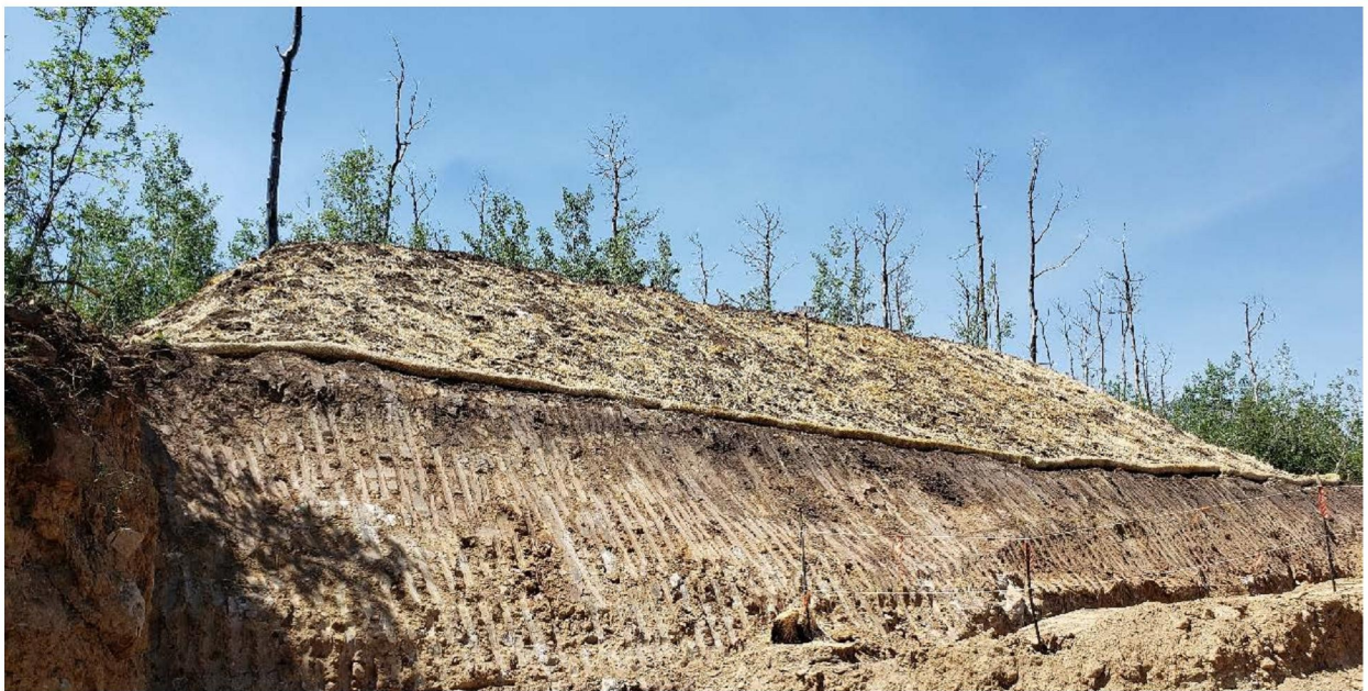
Figure 6: Topsoil stockpiled on SS2-5 pad
