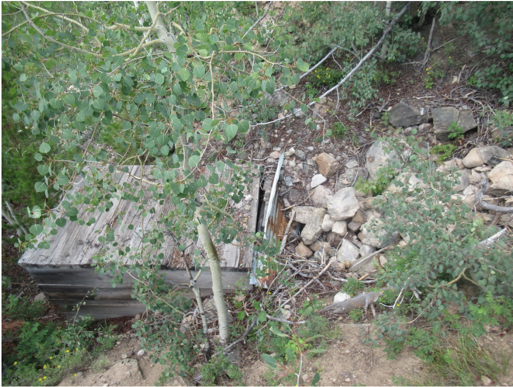
View of collapsed tunnel behind the adit
