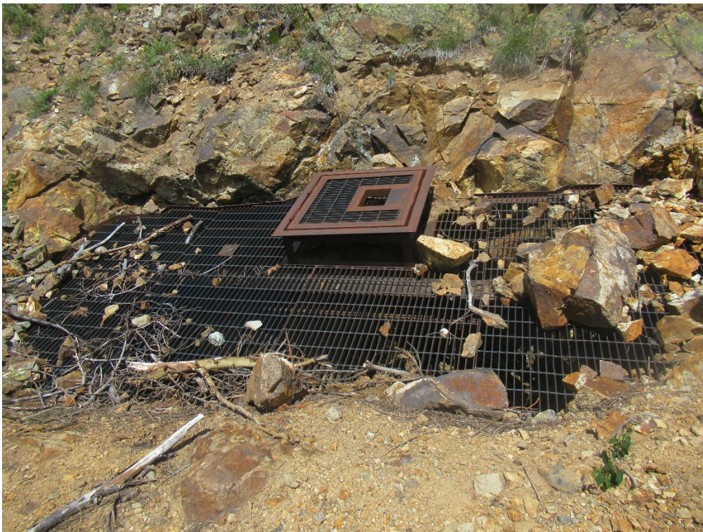
View of AML shaft closure grate
