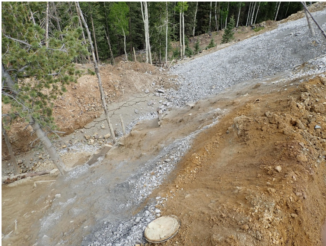
Photo 8. Fine grain material (flotation mill tailings) on out-slope of waste rock dump; looking north.
