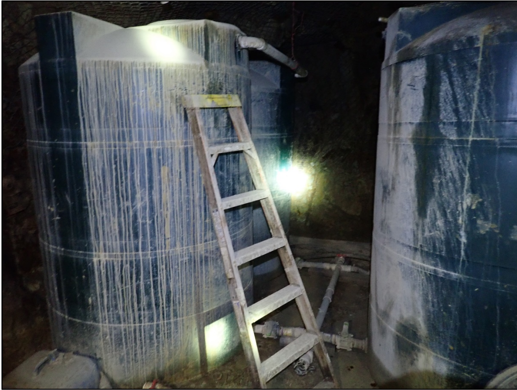
Photo 9. 5,000 gallon fresh water storage are on lower level of mill.
