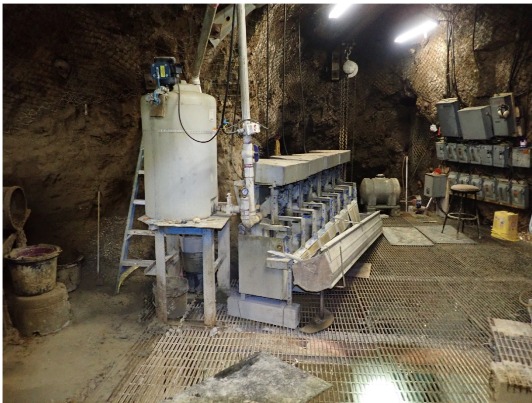
Photo 6. The second of two flotation machines on upper level of mill.
