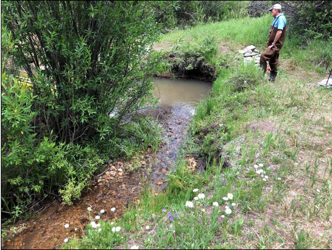
Photo 7. View looking downstream on Beaver Creek directly upstream of larger hole. Operator has backfilled holes in this section of the creek with tailings material.
