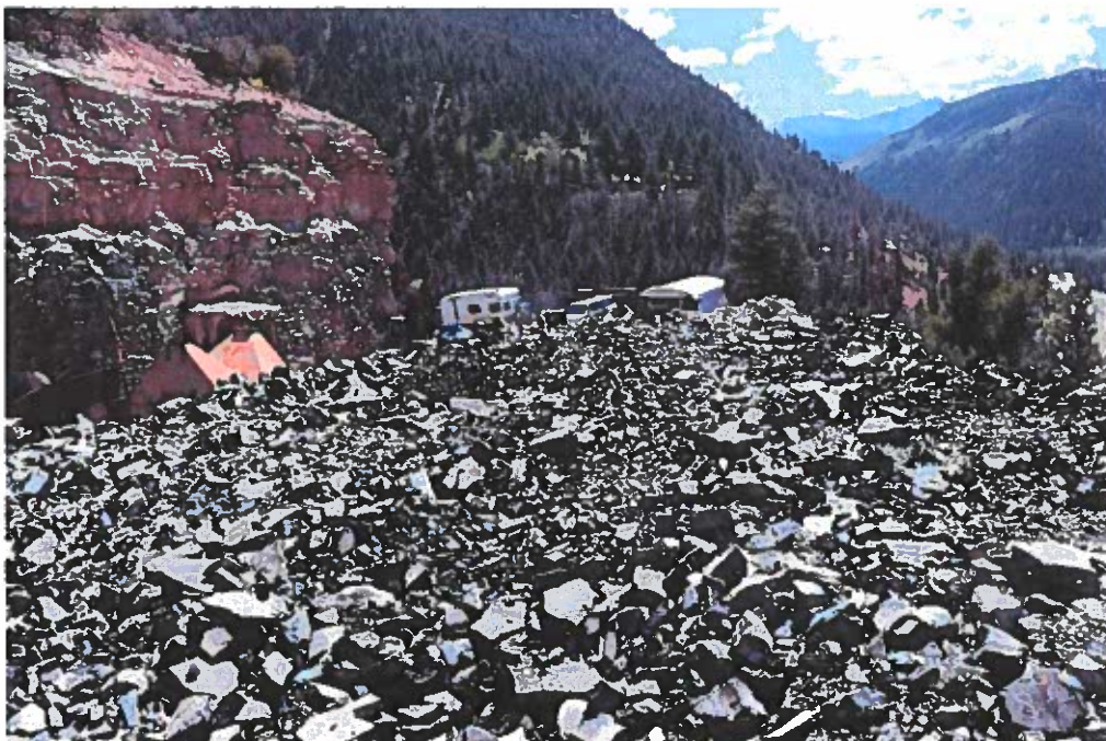
Unstable rock fin removed. In its place is a "berm" approximately 100 feet long.
