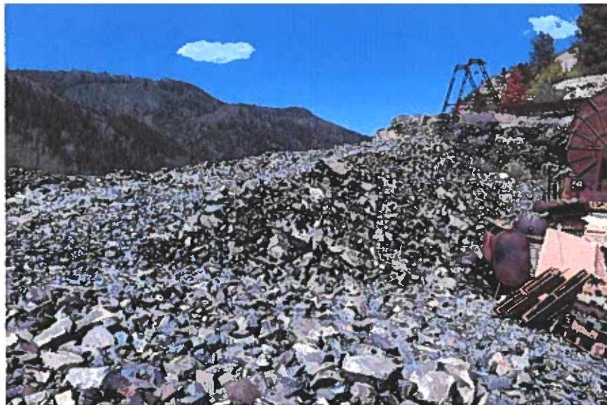
View of new berm looking West (formerly unstable limestone fin)
