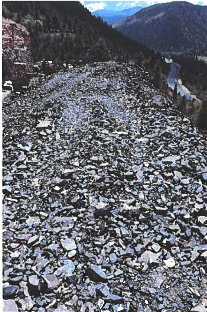
Photo 10. View looking East (note Colorado Hwy 145 in upper right). This is the resulting berm from the demolition of unstable limestone fins left by former mining operations.
