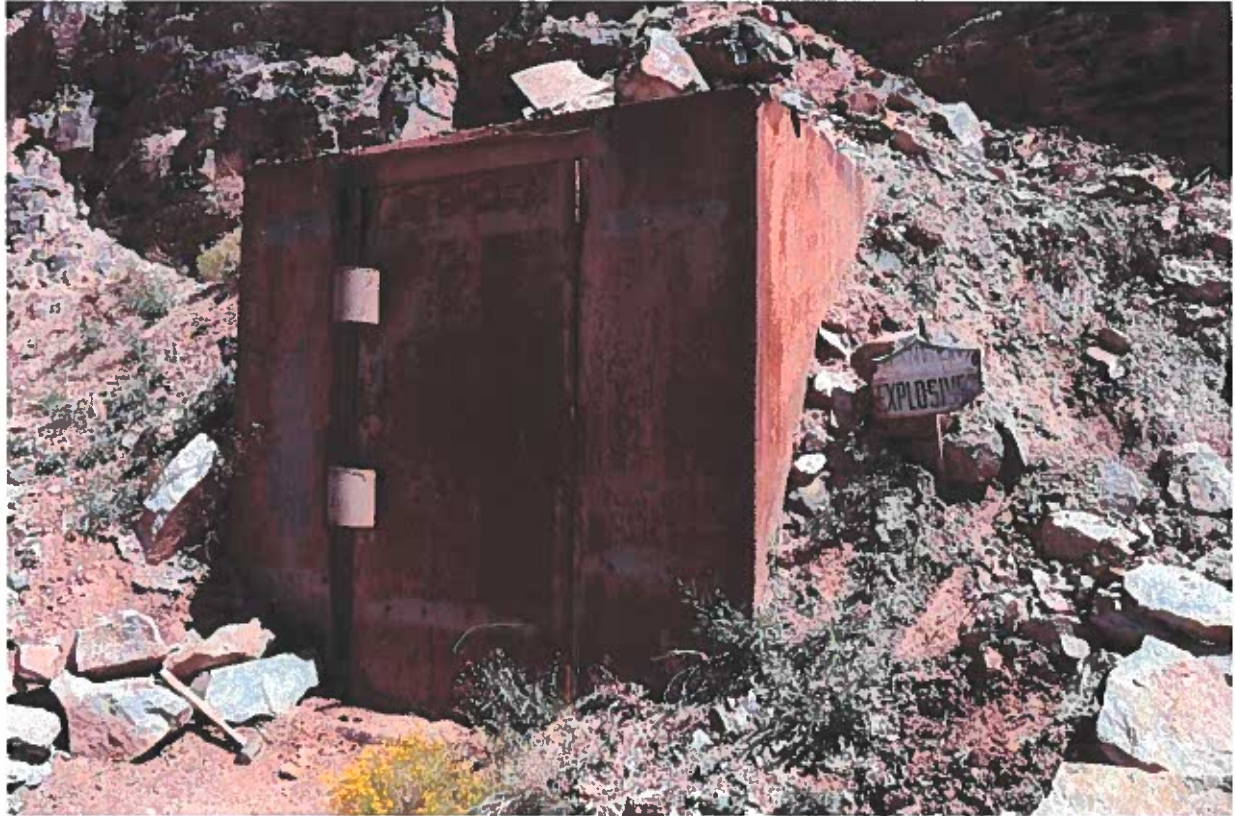
Photo 9. Door hinge repaired on Explosives magazine such that door can now be secured. Note: This steel structure only used for fuels, not explosives.
