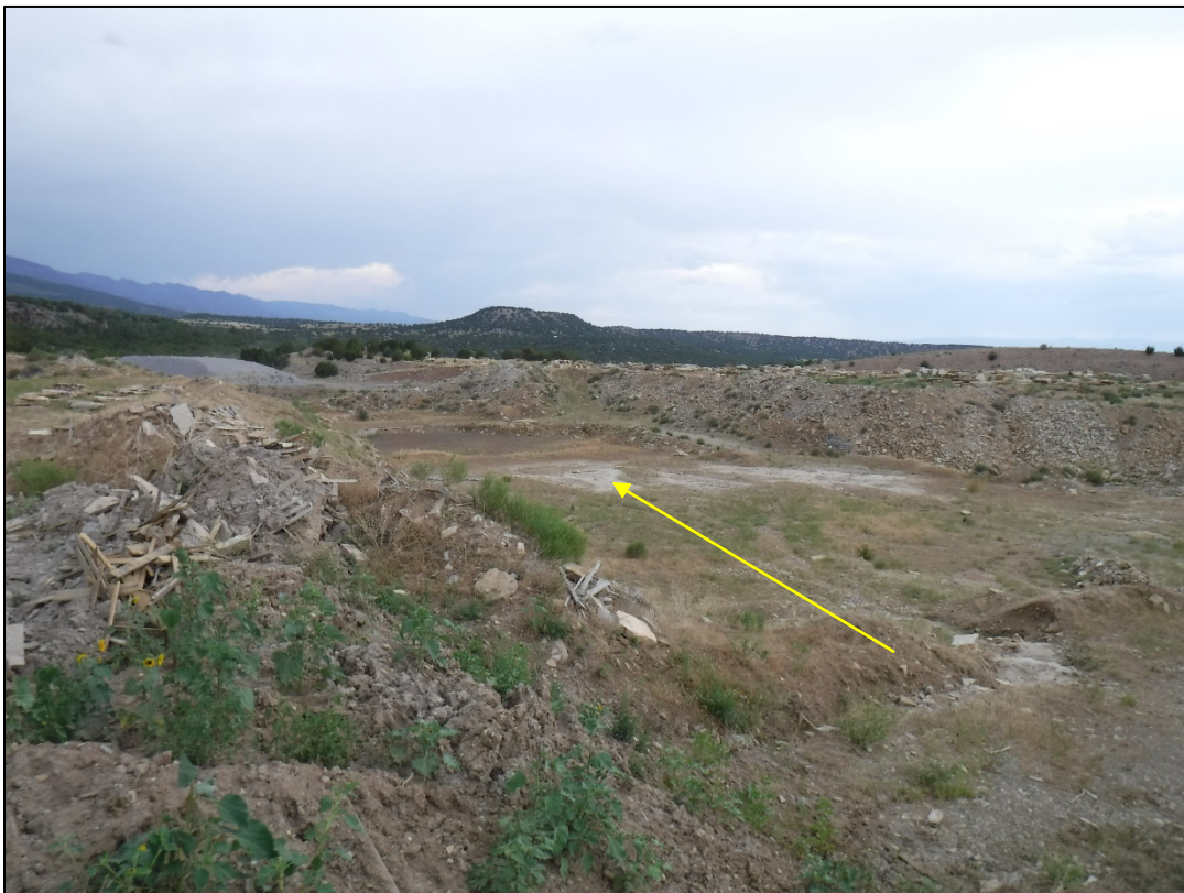
Photo 6: Area of potential pond (arrow) that should be graded to prevent ponding
