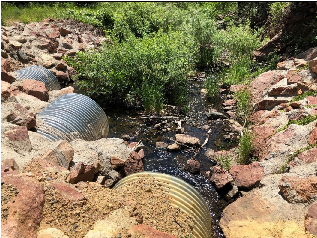
Photo 34. View looking downstream on Ralston Creek at surface water monitoring location SW-FBRG located downstream of mine site (outside permit area), below SW-BPL.
