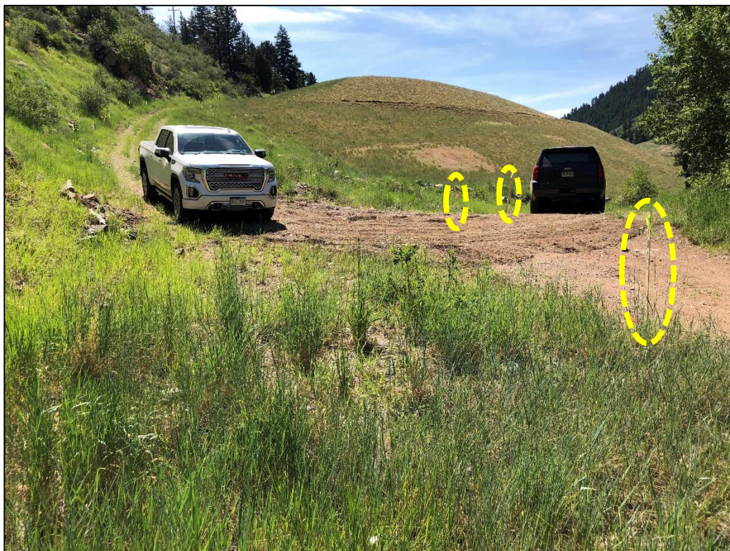
Photo 30. View looking east across area located north of NWRP where stormwater diversion channel dissipation basin (approved in TR-28) will be installed. Stakes (circled) mark alignment of this structure.
