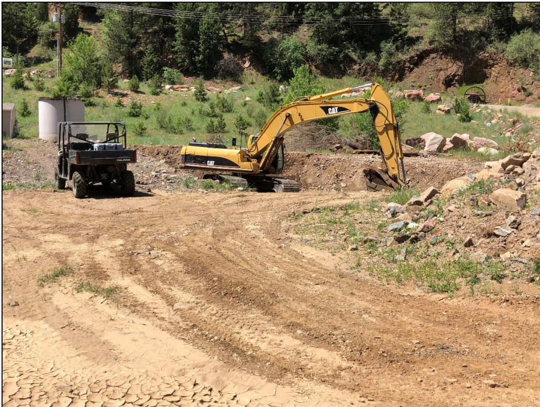
Photo 14. View looking south across southern portion of northern excavation area located near new water treatment plant area.
