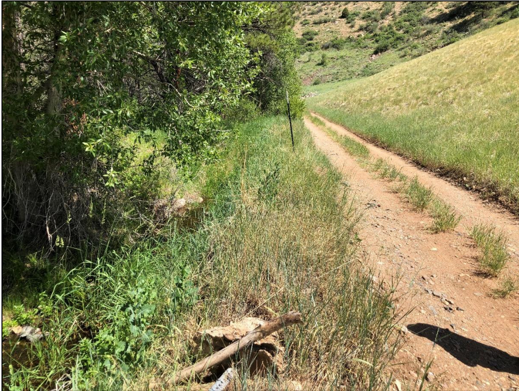
Photo 17. View looking north along Glencoe Valley Road at toe of NWRP, showing roadside ditch (at left) in which slightly green-colored water was ponded during inspection. This water is believed to be “seep water” from the NWRP.
