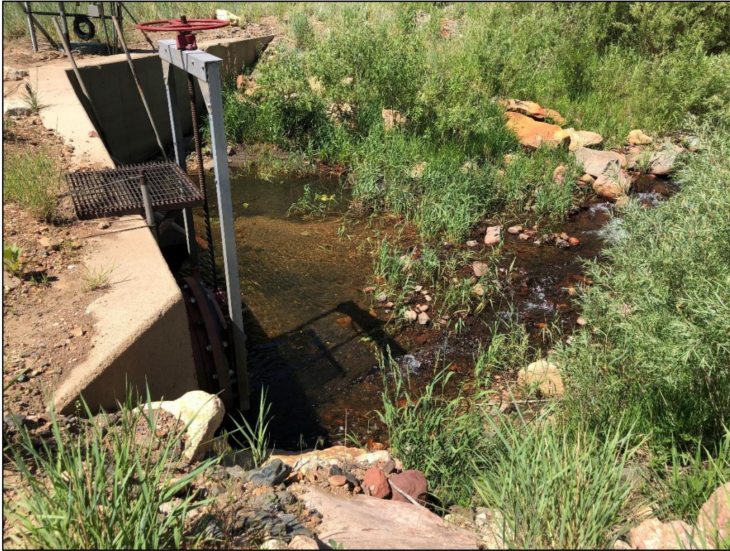
Photo 15. View looking at upgradient cutoff wall/headgate in Ralston Creek, showing creek flowing upstream of cutoff wall during inspection.
