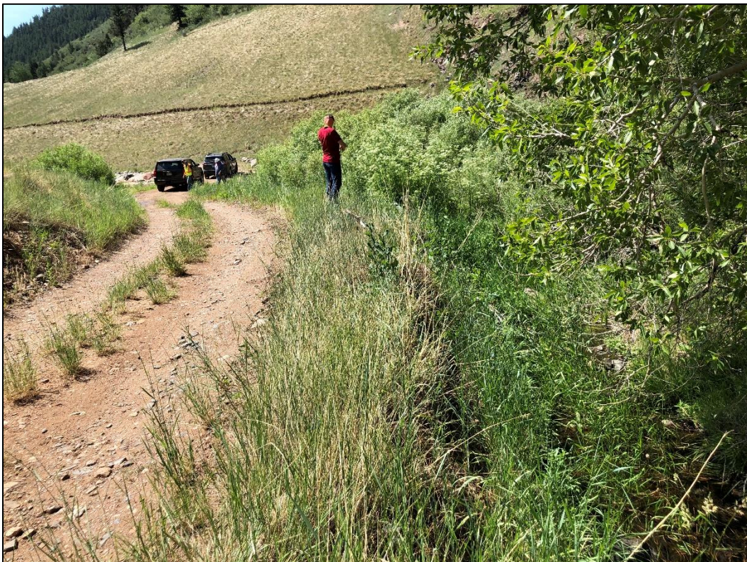
Photo 18. View looking south along Glencoe Valley Road at toe of NWRP, showing roadside ditch (at right) in which slightly green-colored water was ponded during inspection. This water is believed to be “seep water” from the NWRP.
