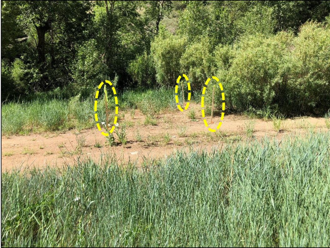
Photo 31. View looking west across Glencoe Valley Road from north of NWRP showing area where stormwater diversion channel dissipation basin roadway crossing (approved in TR-28) will be installed. Stakes (circled) mark alignment of this structure.
