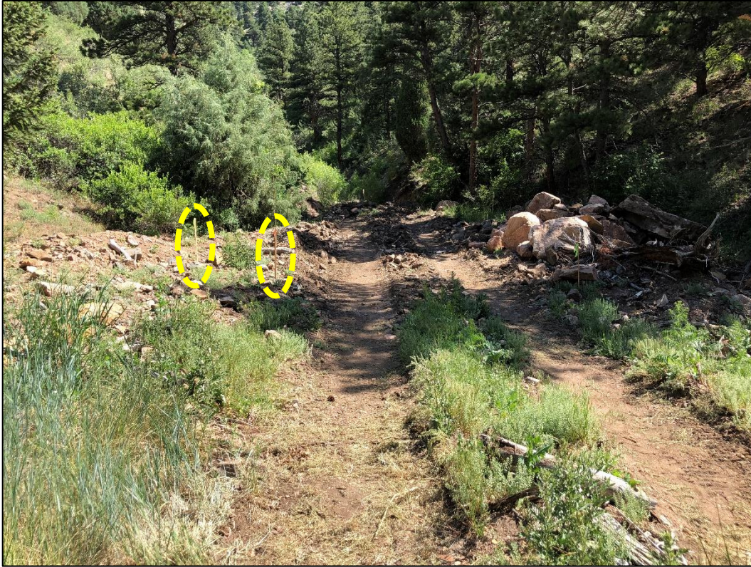
Photo 23. View looking northeast across top of NWRP toward ephemeral drainage above the pile (in background). Note alignment of stormwater diversion channel (approved in TR-28) has been staked out (stakes circled).
