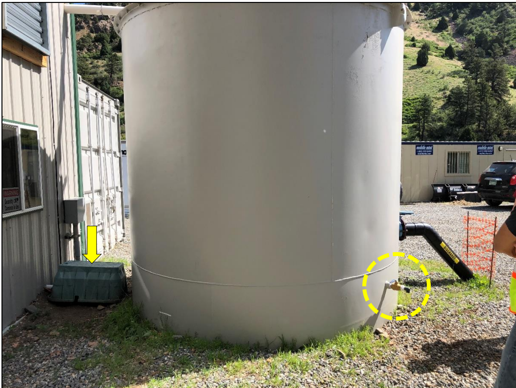
Photo 6. Side view of discharge tank shown in Photo 5. This tank was deep cleaned recently and a new sampling port was installed (circled). The old sampling port is located at the back of the tank (under green bucket; location indicated with arrow).
