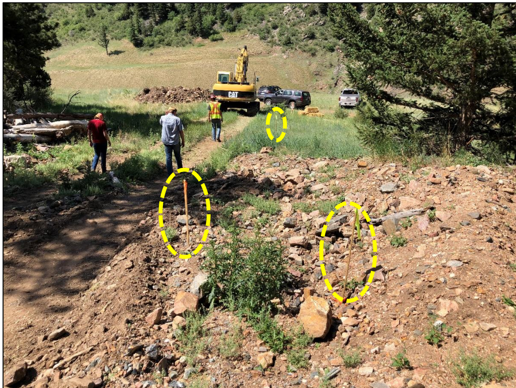
Photo 22. View looking southwest across northern edge of NWRP where alignment of stormwater diversion channel (approved in TR-28) has been staked out (stakes circled).
