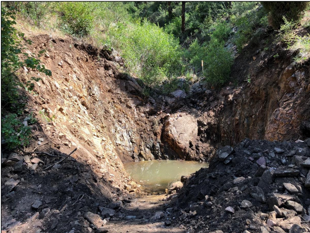
Photo 24. View looking northeast across excavated area at top of NWRP where concrete seal wall will be installed in accordance with TR-28.
