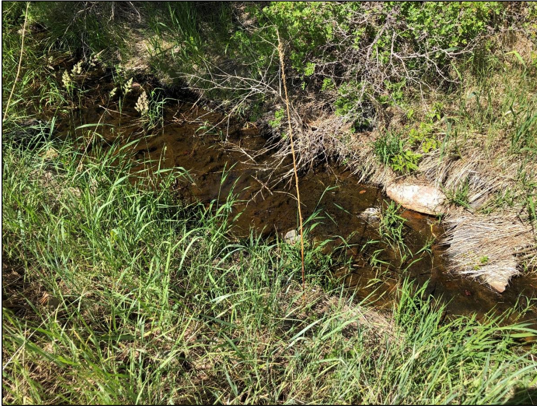
Photo 19. View of slightly green-colored water ponded in roadside ditch near toe of NWRP during inspection. This water is believed to be “seep water” from the NWRP.
