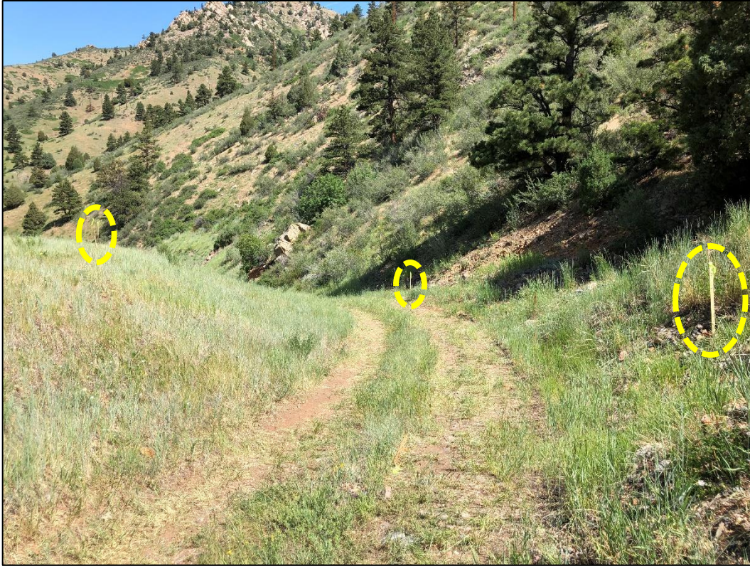
Photo 21. View looking northwest across northern edge of NWRP where alignment of stormwater diversion channel (approved in TR-28) has been staked out (stakes circled).
