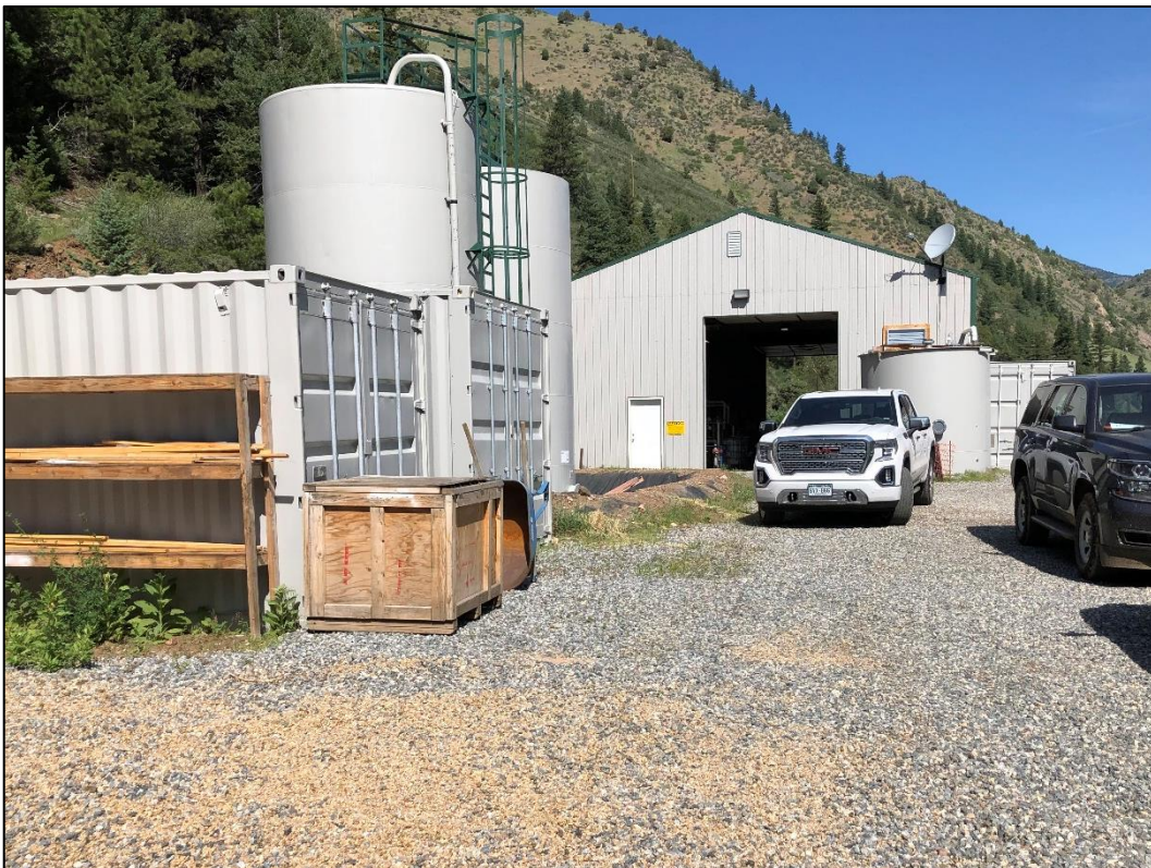
Photo 4. View looking northwest at new water treatment plant constructed on top of mesa south of Ralston Creek.
