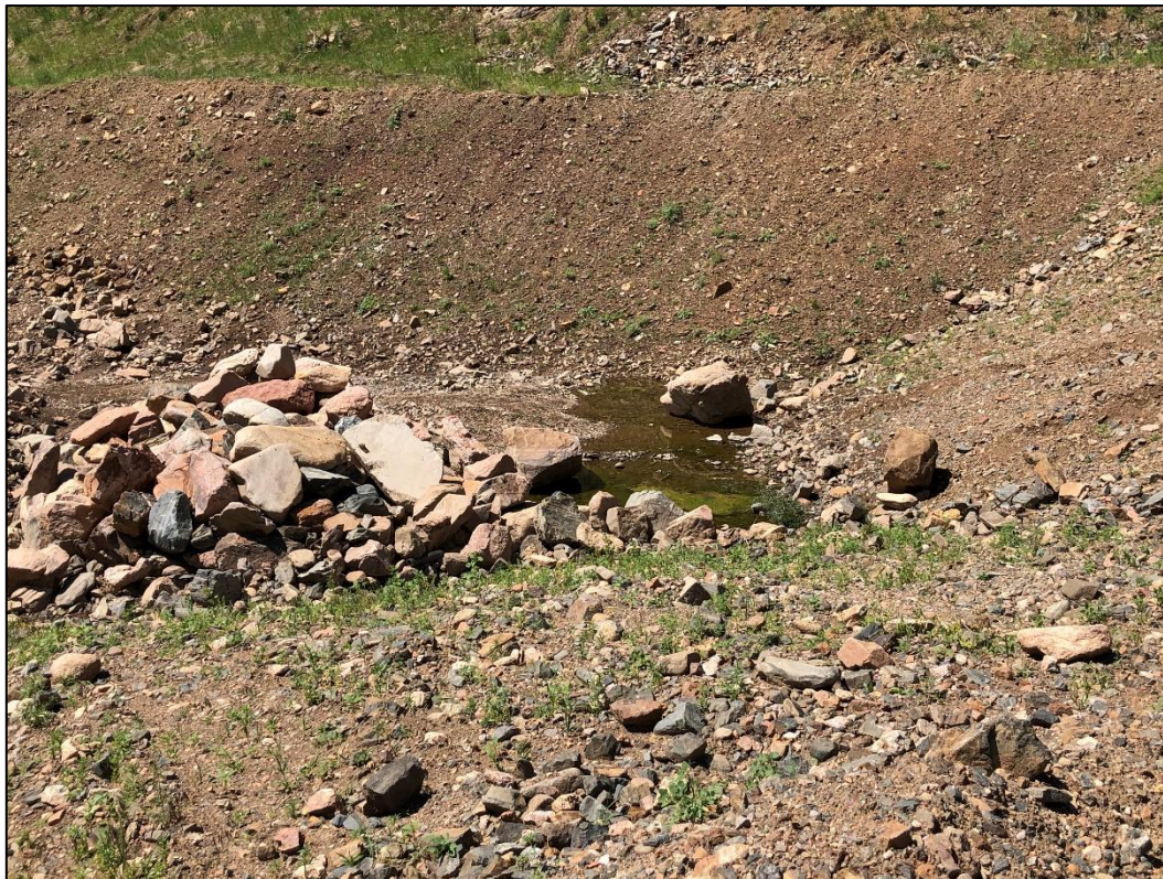
Photo 12. View looking west across central portion of northern excavation area.
