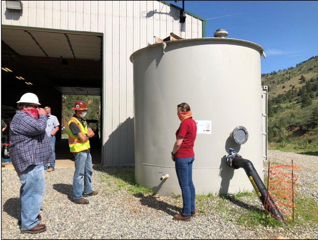
Photo 5. View looking northwest at discharge tank located at southeastern corner of water treatment plant, from which treated water is discharged (through pipeline shown at bottom right) to Ralston Creek at SW-BPL.
