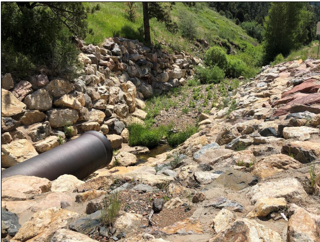
Photo 16. View looking downstream from upgradient cutoff wall in Ralston Creek, showing creek channel dry downstream of cutoff wall during inspection.
