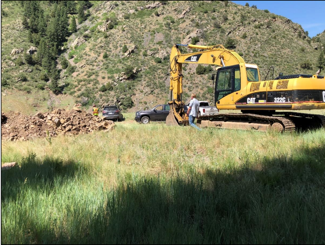
Photo 25. View looking southwest across top of NWRP showing excavator and stockpiled material excavated from drainage area temporarily stored on top of pile.
