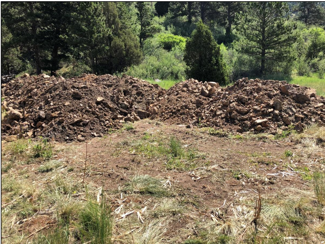
Photo 26. Closer view of stockpiled material excavated from drainage area temporarily stored on top of NWRP. Radiation testing will be performed on this material to determine whether it will require disposal in the Minnesota Mine.
