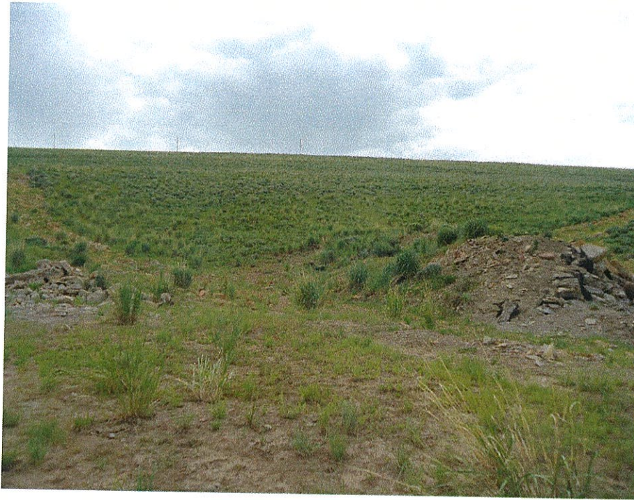
Photograph 6: West Side Fill 3H: 1V Face Looking East (6/25/2020)
