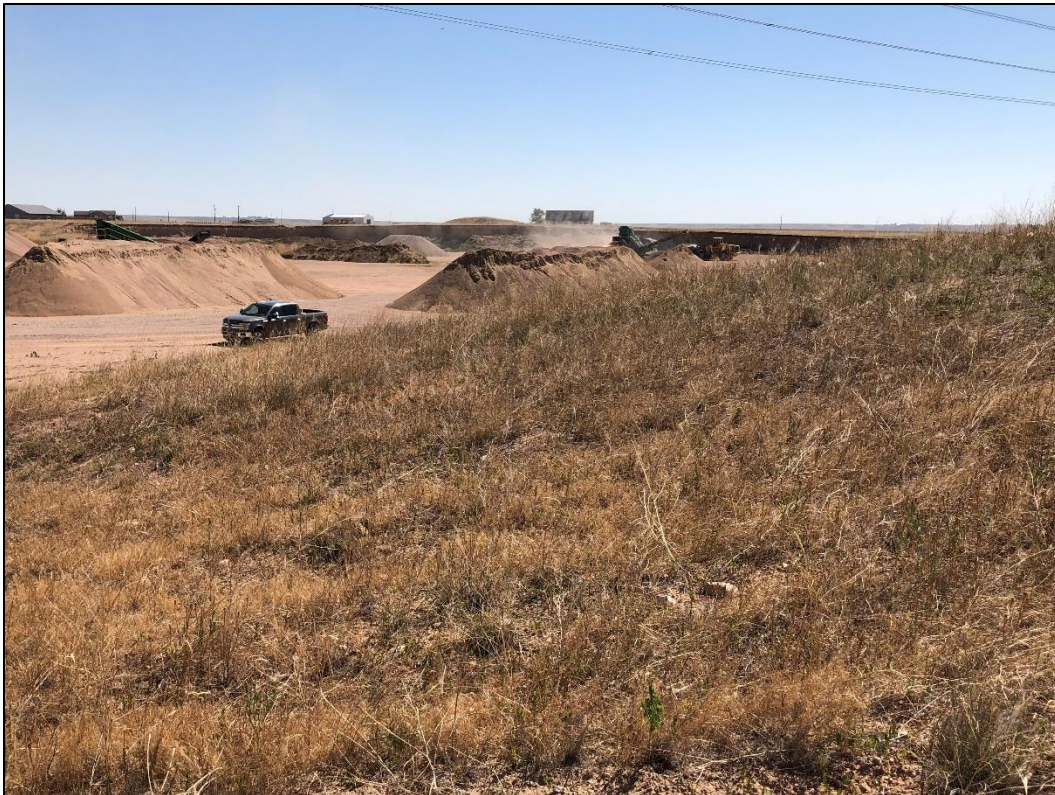
Photo 16. View looking east across reclaimed southwestern pit wall with slopes of 3H:1V or flatter and established grass cover.
