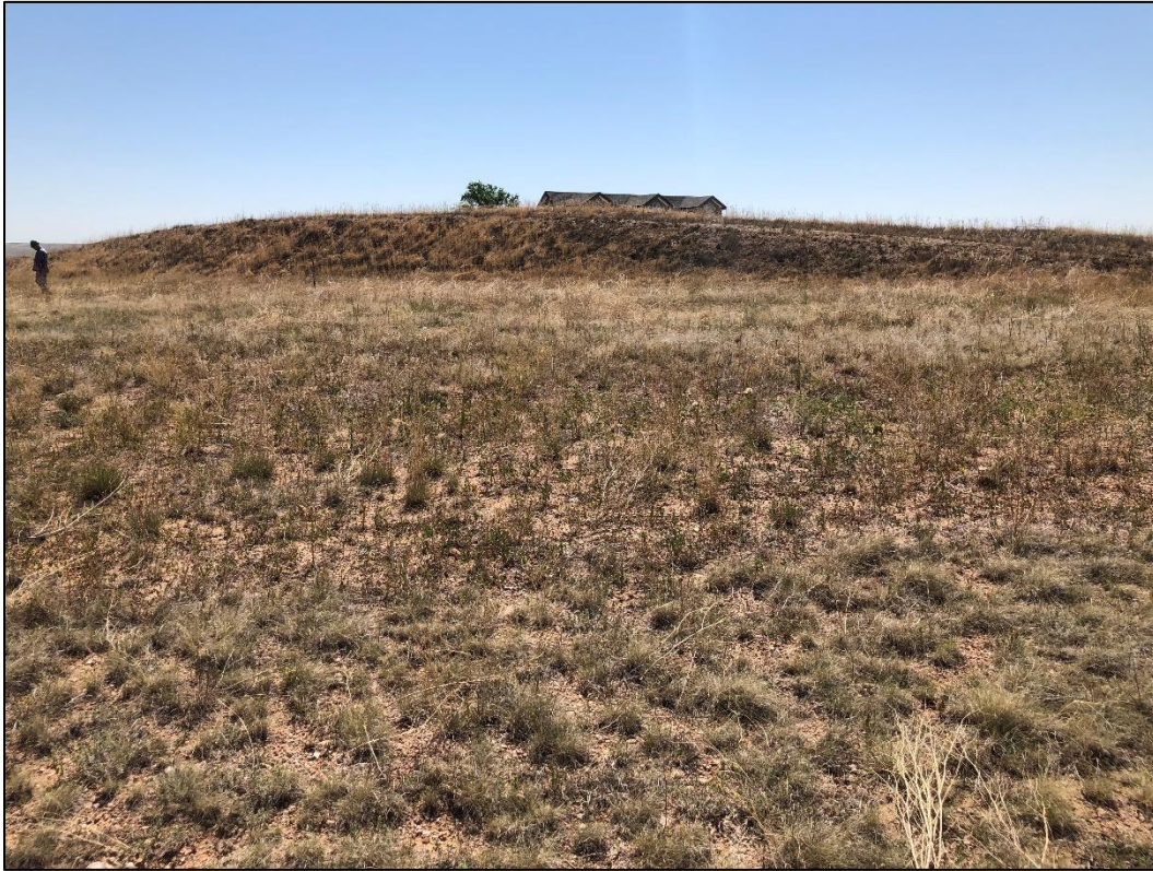
Photo 19. View looking southeast at large topsoil stockpile stored at eastern edge of site. Areas north of this stockpile which were disturbed by previous stockpiling activities are reclaimed with established grass cover.
