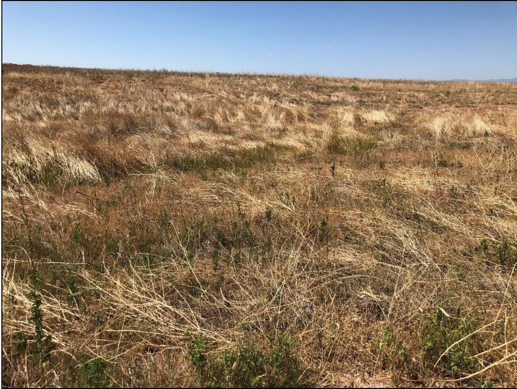
Photo 15. View looking southwest across reclaimed southwestern portion of pit with slopes of 3H:1V or flatter and established grass cover.
