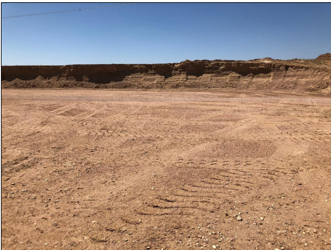
Photo 6. View looking south at southeastern pit wall approximately 15-18 feet in height with near vertical slopes.
