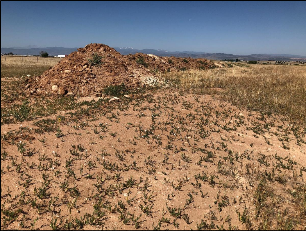
Photo 9. View looking west at topsoil stockpile stored along top of reclaimed southwestern pit wall.
