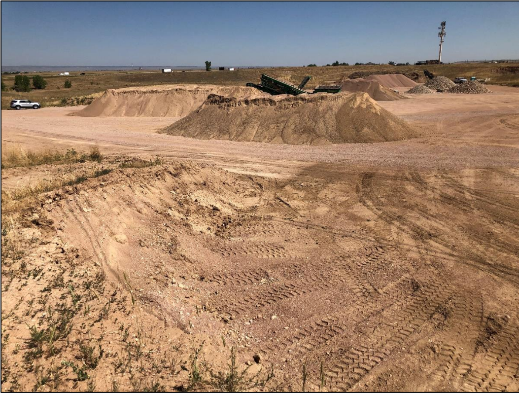
Photo 3. View looking north across pit from its southern edge. Note several material stockpiles and processing equipment stored on pit floor (in background).
