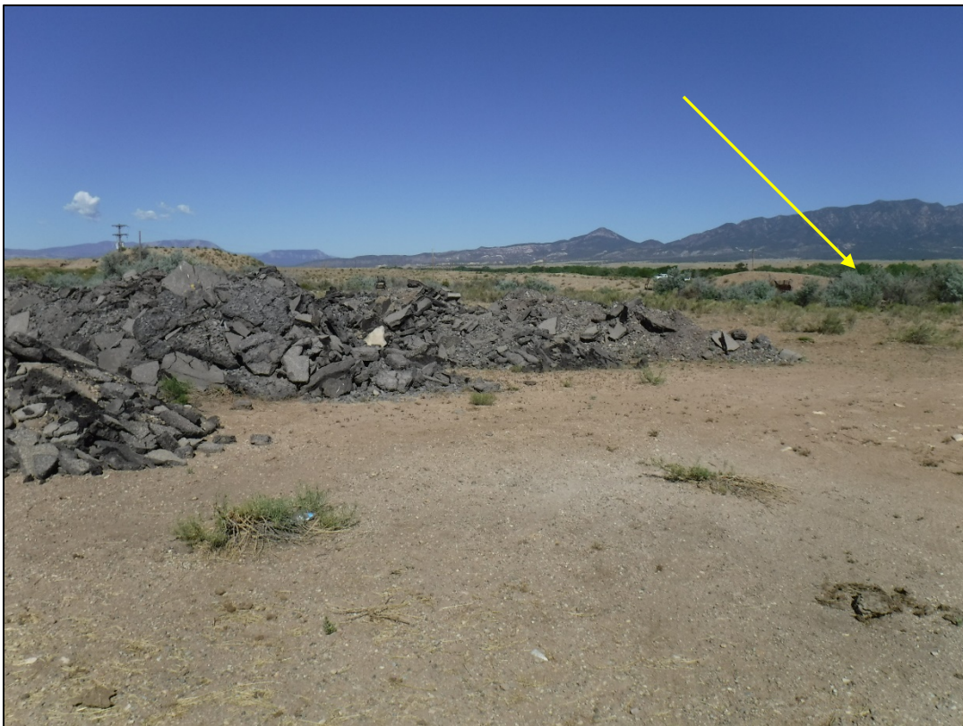
Photo 6: Asphalt debris in the foreground and the depressed area requiring re-contouring yellow arrow
