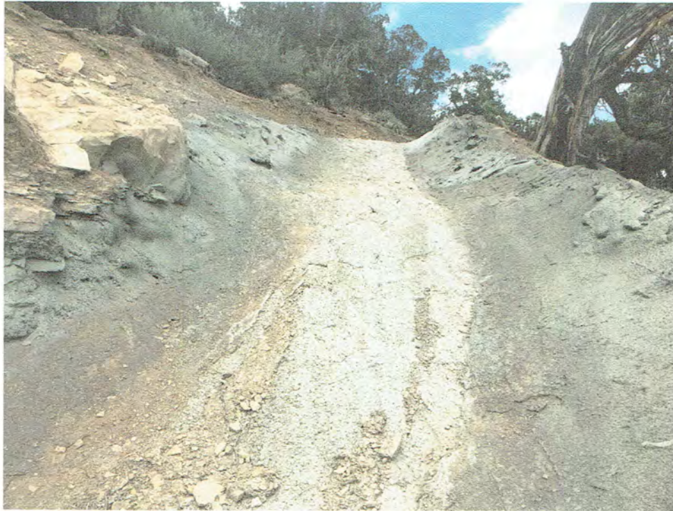
Pic. 1 –Reach 1, additional grouting along sides of upper section, grouted channel.
