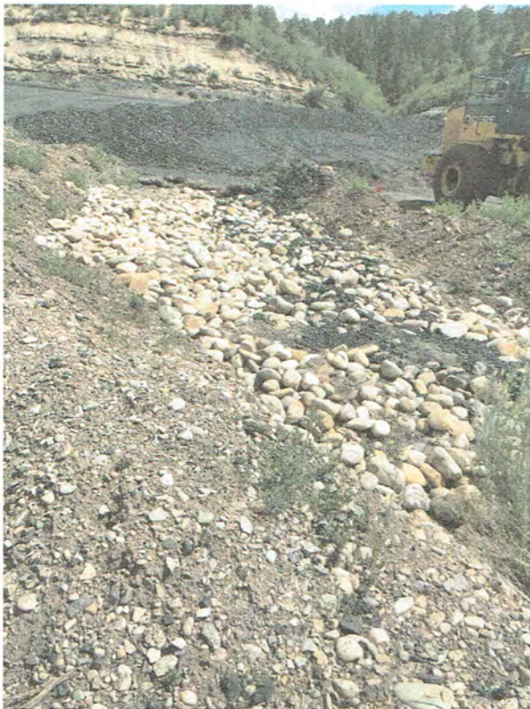
Pic. 6 – Improvements preventing excess sedimentation at Reach 7/foundation drain.
