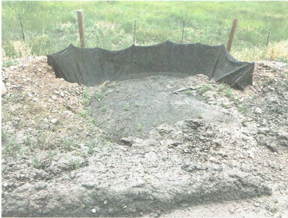
Pic. 3 – Sediment trap at driveway.
