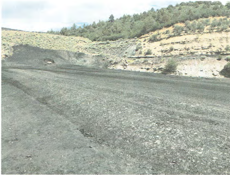
Pic. 5 – Placement of waste material at base of existing embankment pile.
