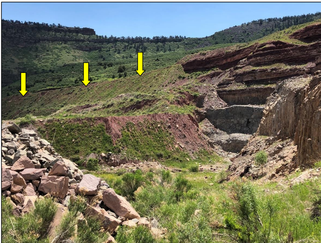
Photo 10. View looking east/southeast across pit floor of larger eastern portion of quarry. Note backfilled portion of highwall in background (indicated). Edge of backfill visible on pit floor.
