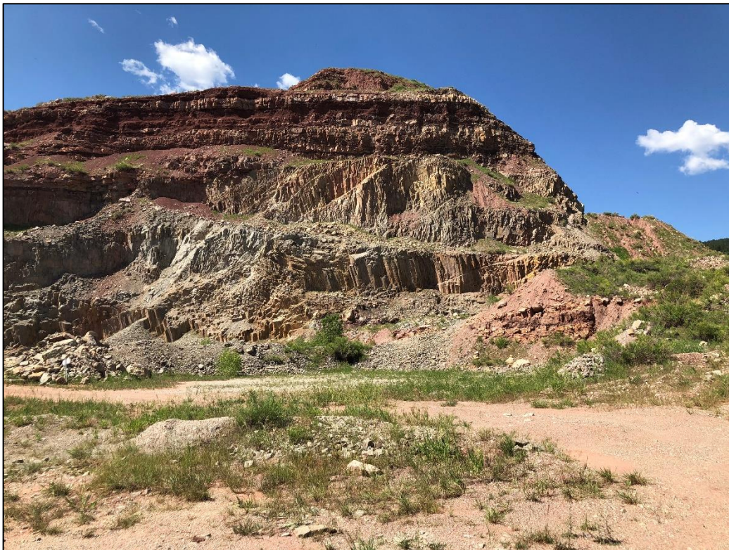
Photo 4. View looking southwest across central portion of quarry, showing highwall in background up to approximately 150 feet in height with near vertical slopes.
