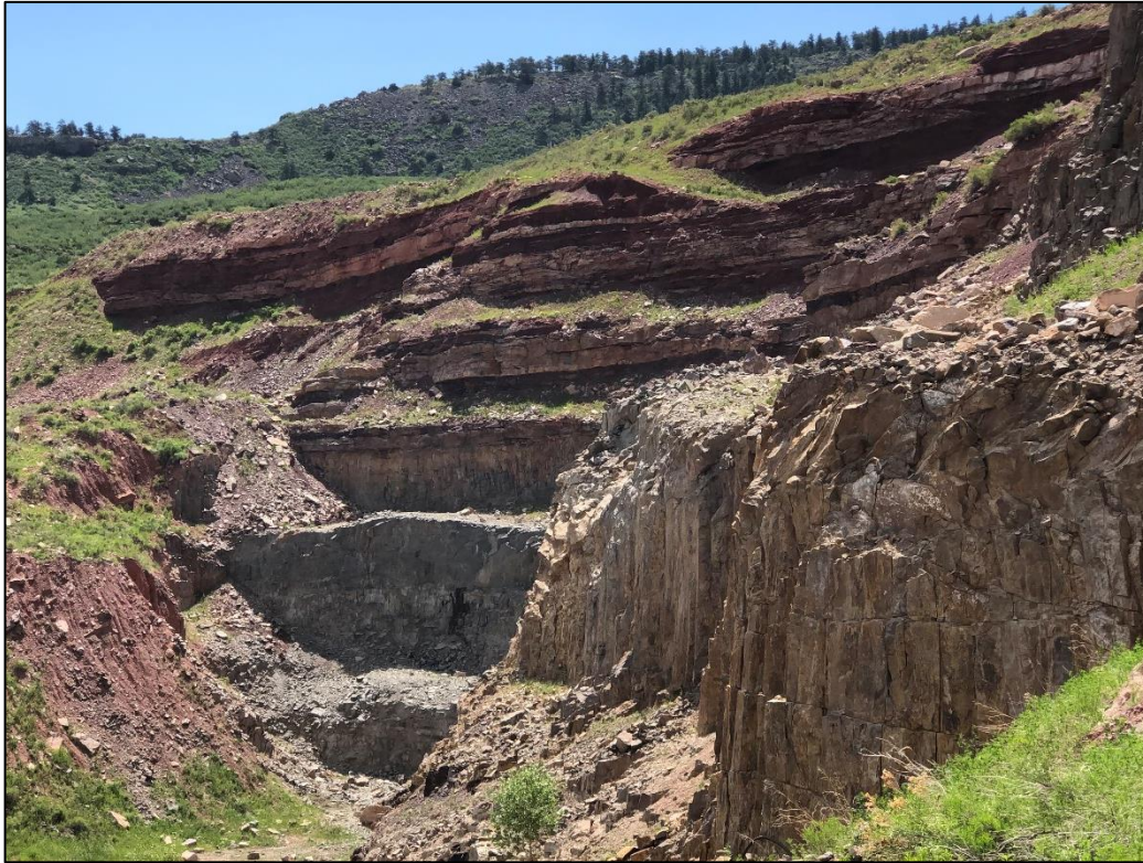
Photo 11. Closer view of unbackfilled eastern portion of highwall (shown in Photo 10), benched with near vertical slopes.
