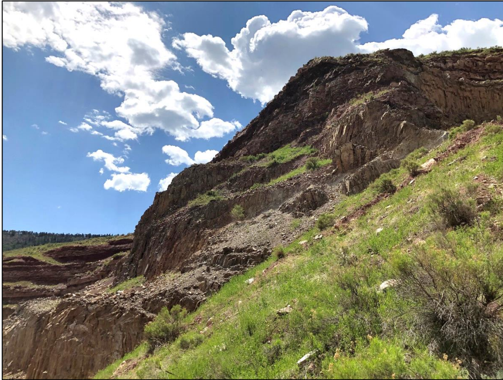
Photo 9. View looking southeast across central portion of highwall which has some irregular benching with near vertical slopes.
