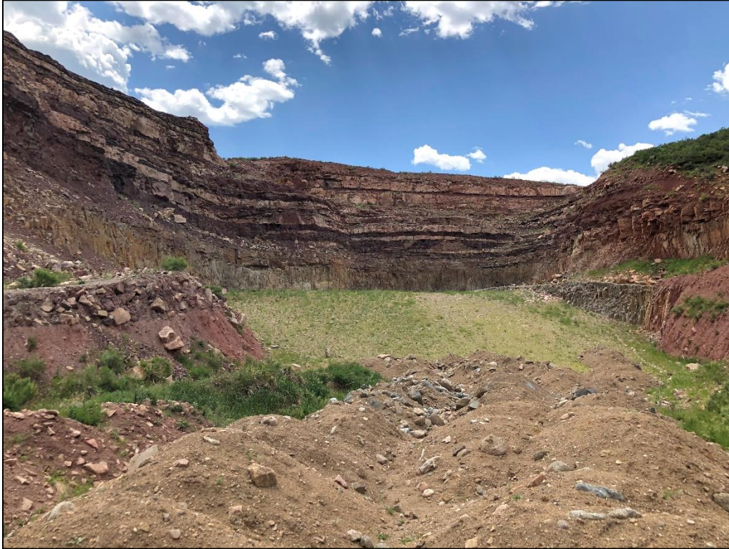
Photo 15. View looking south across western portion of quarry where county has placed imported inert backfill material in accordance with TR-3. Approximately 80-100 feet of near vertical highwall remains above current backfill surface.
