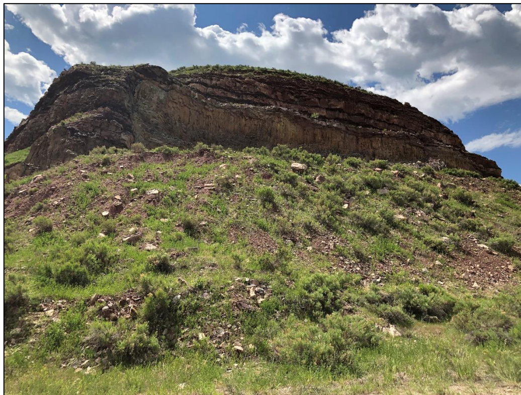
Photo 12. View looking southeast at highwall along edge of ridge which extends into quarry, separating larger eastern pit from smaller western pit. Large overburden/waste rock stockpile visible in foreground.
