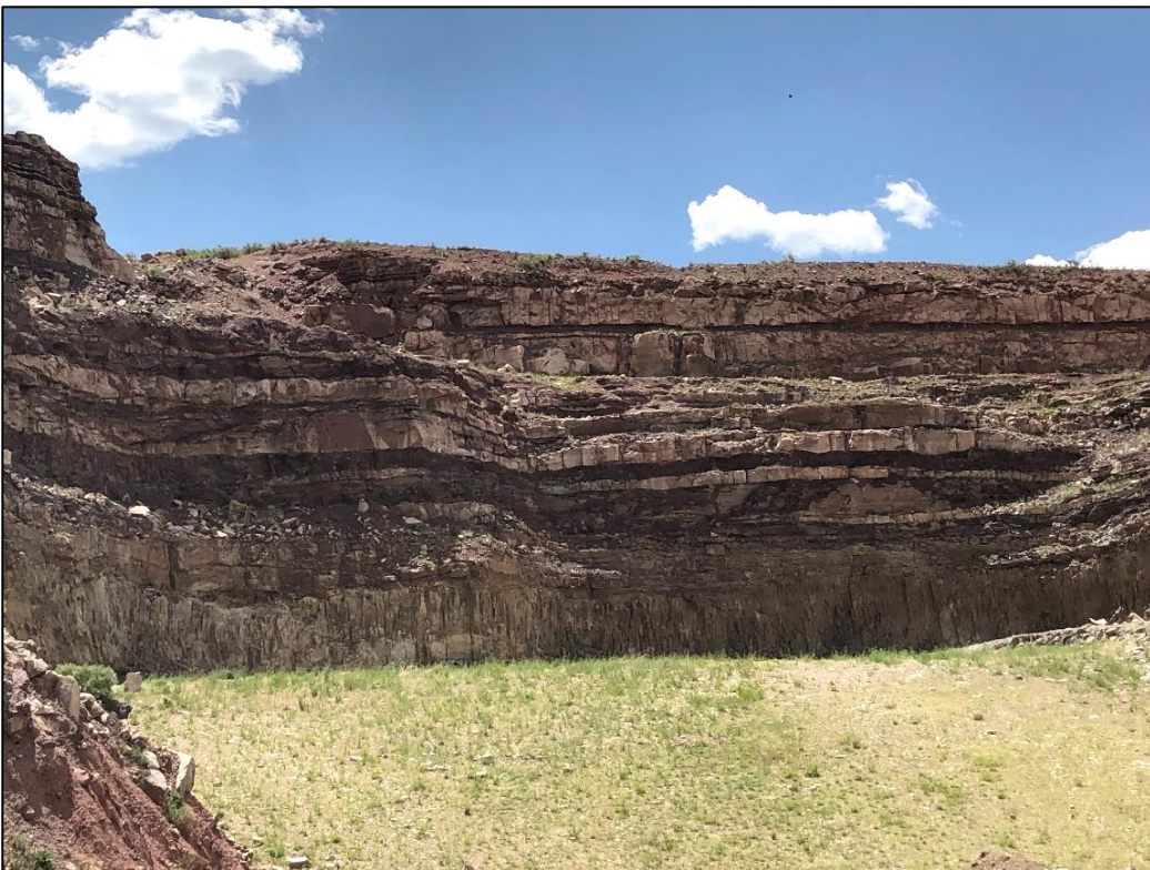
Photo 16. Closer view of near vertical highwall in western portion of quarry (shown in Photo 15). Current backfill surface is shown at bottom.
