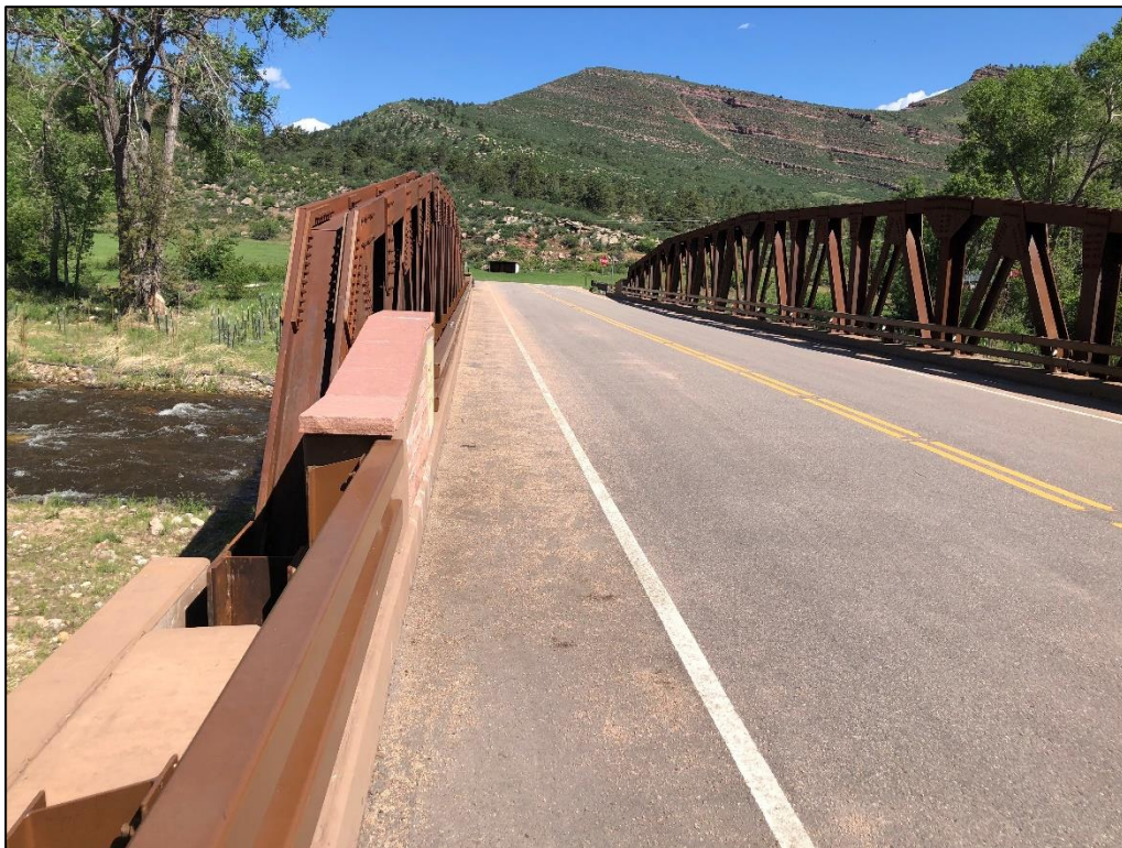
Photo 2. View looking northwest across new steel truss bridge constructed by county connecting Hwy 7 to Old St Vrain Rd. Construction of this bridge restored access to the Lyons Quarry.
