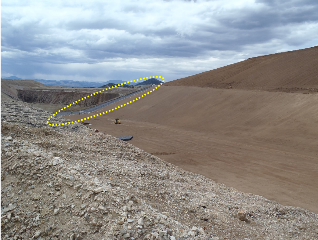
Photo 8. VLF 2 Phase 2 beginning of geomembrane installation.
