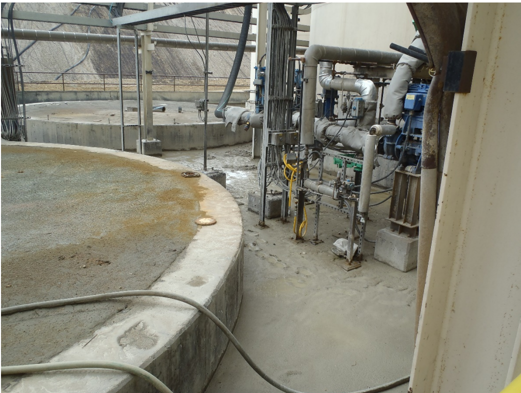
Photo 7. Sludge in HGM vat leach area.
