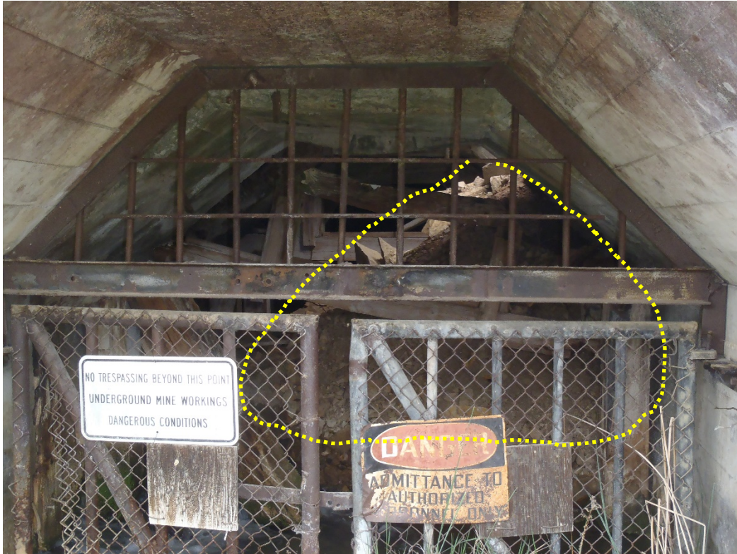
Photo 2. Carlton Tunnel outlet view of failure material (outlined).
