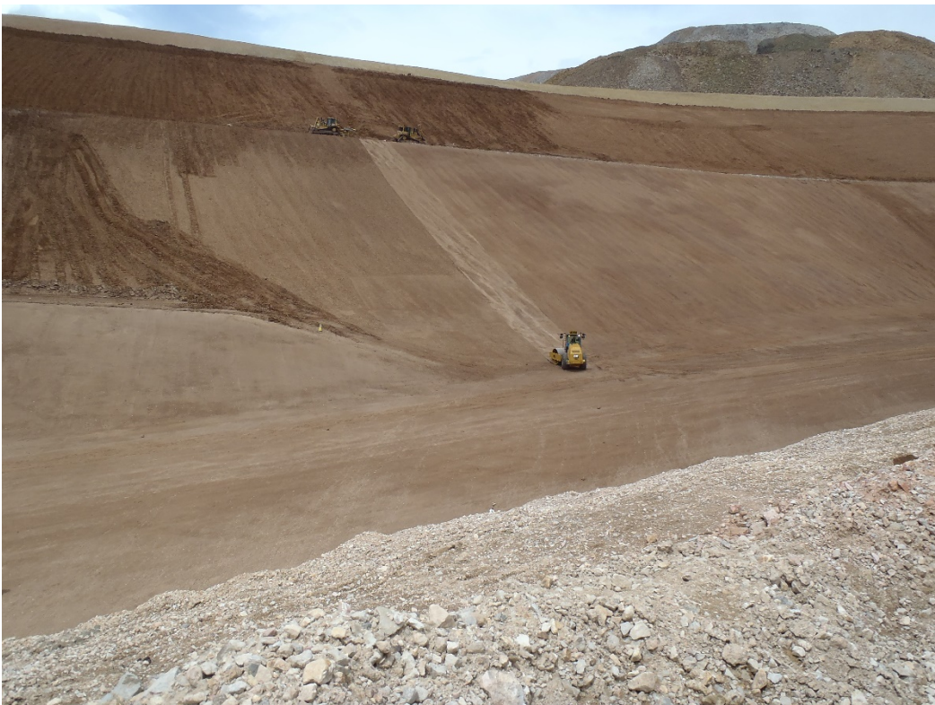
Photo 9. VLF 2 Phase 2 SLF compaction effort.
