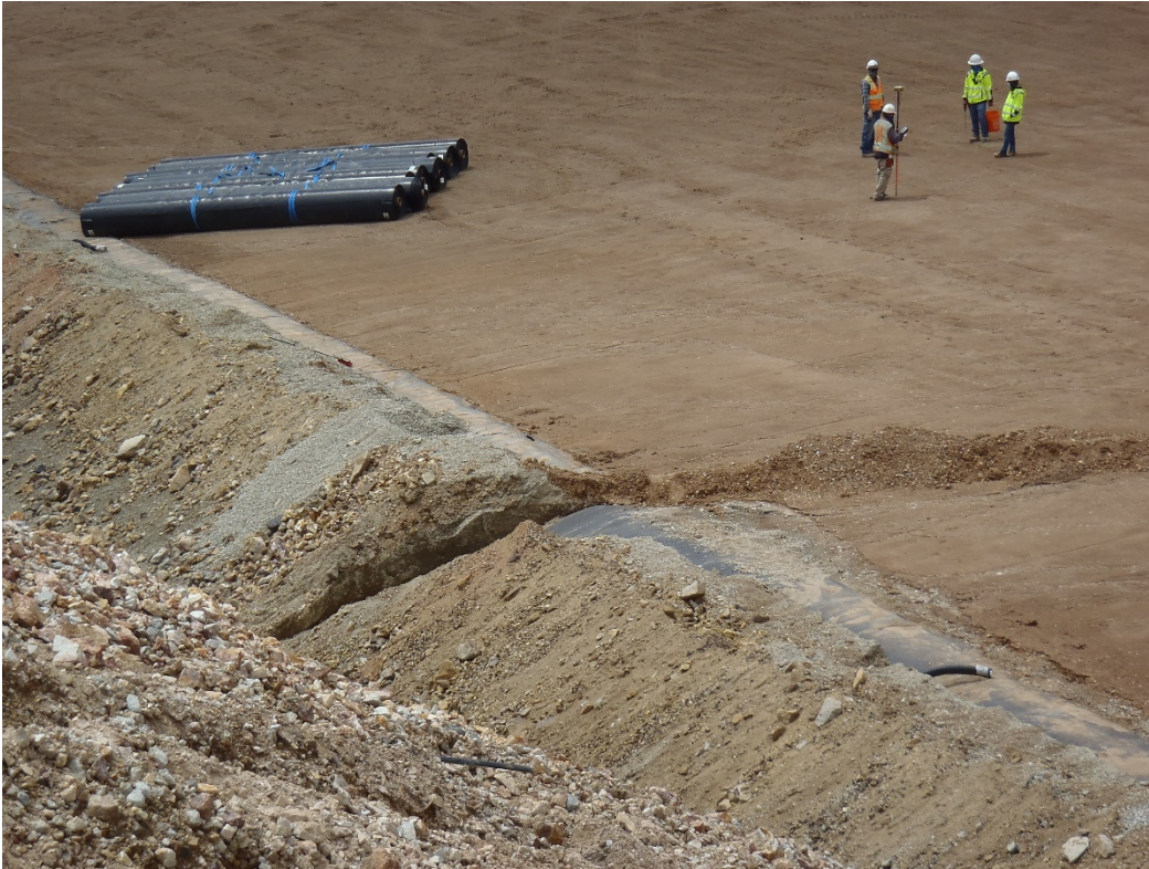
Photo 10. Crew verifying SLF required thickness.
