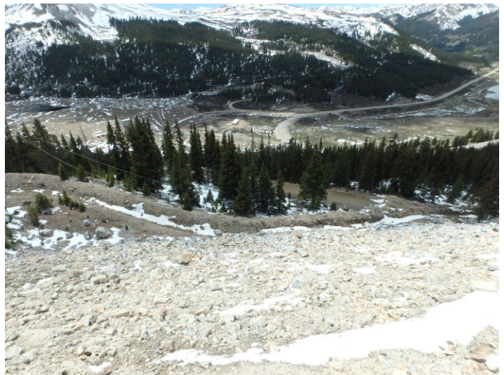
Ceresco Seepage Collection Ditch
