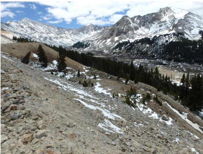
Ceresco Seepage Collection Ditch
