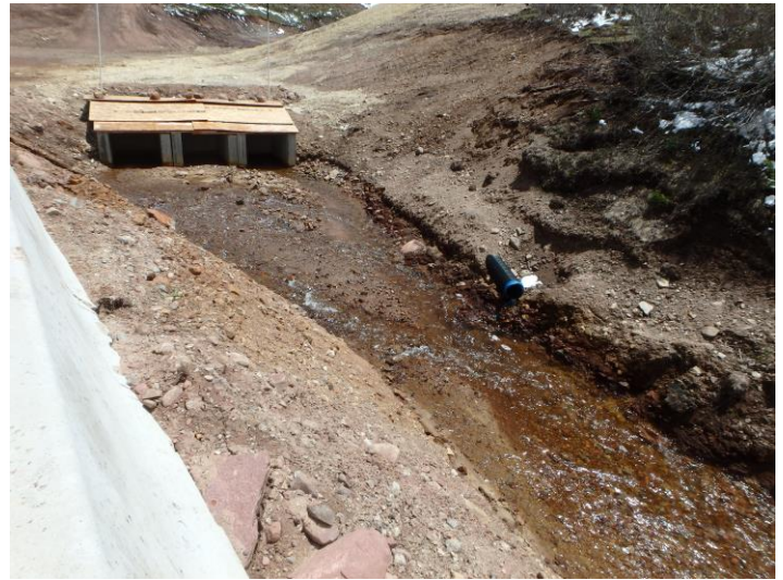
Surface water bypassing underdrain redirected into McNulty Ditch
