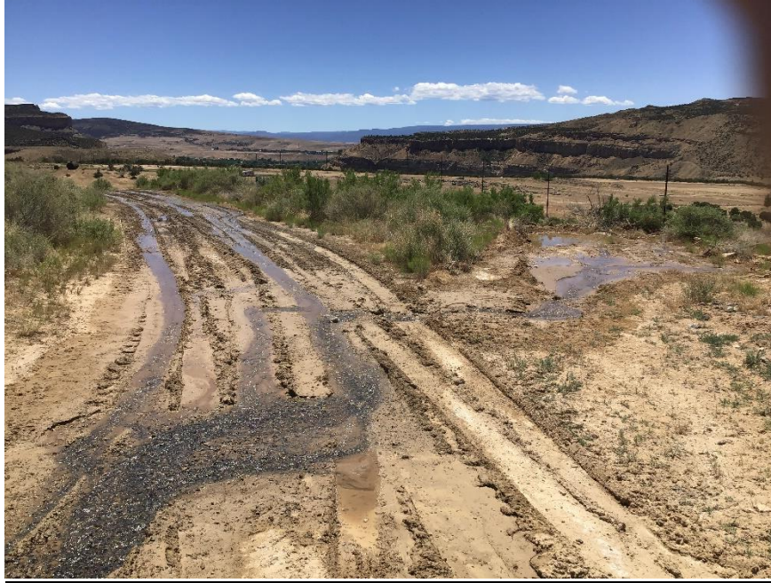
Photo 7: The tail water from the landowner's field running across the access road. The photo was taken looking to the south. The reclaimed barrow area and drainage is located off the photo to the right.
