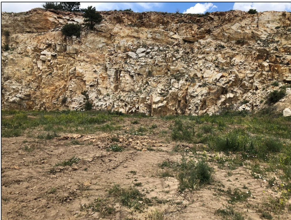
Photo 2. View looking north at northern pit wall with slopes of approximately 0.5H:1V.
