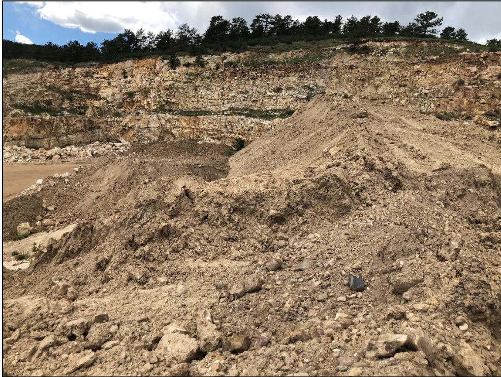
Photo 3. View looking west across northern portion of pit where additional backfill material has been placed since last inspection.
