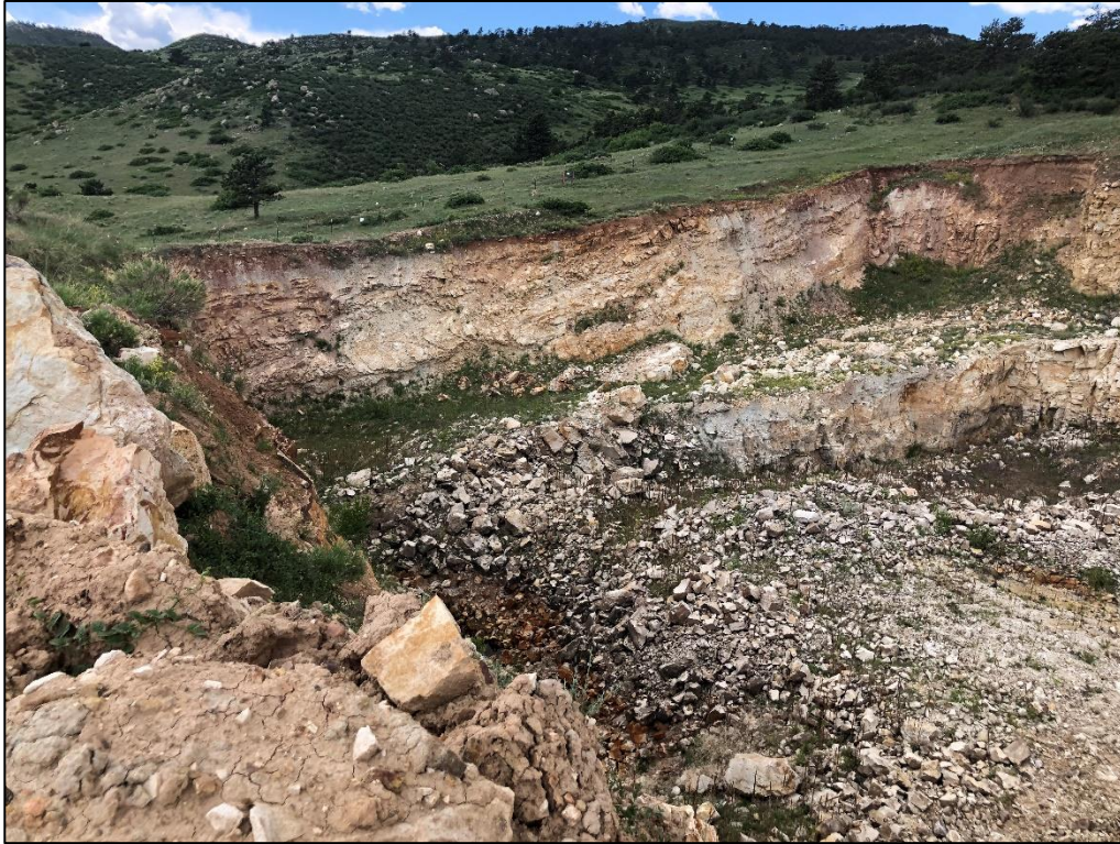
Photo 5. View looking south at southern pit wall with mostly 0.5H:1V slopes.
