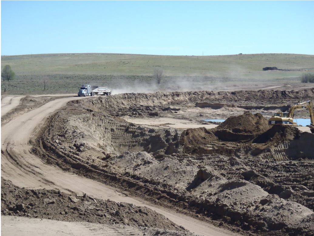
Photo 4. Haul road on west side and typical excavation area – note reservoir water on right (looking NE).
