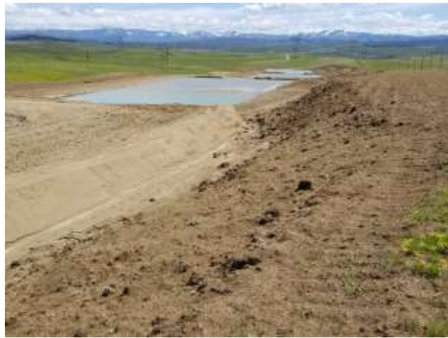
Diversion ditch, slopes seeded, check dams being installed
