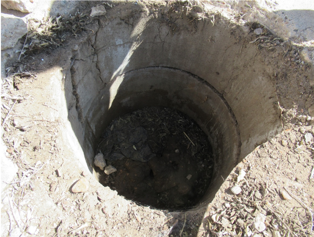
View of backfilled well #23312
