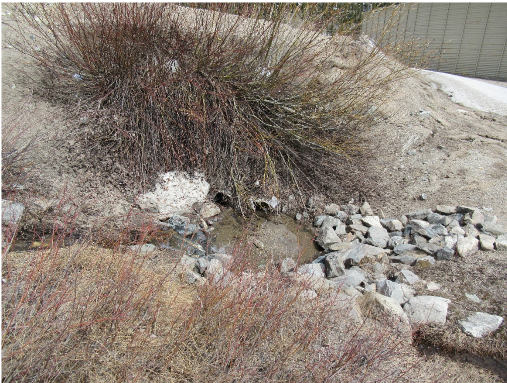
View of partially filled culverts above OF-16
