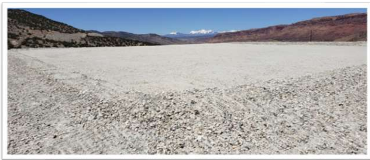
Figure 4: View looking across the Sunday ore pad to the northwest, along the axis of Big Gypsum Valley. The La Sal Mountains, Utah are the snow capped peaks. Note that the working surface of the pad is a finer grain size and is more compacted than the sides (and presumably beneath). I did not observe any liner sticking out the sides or through the top.
