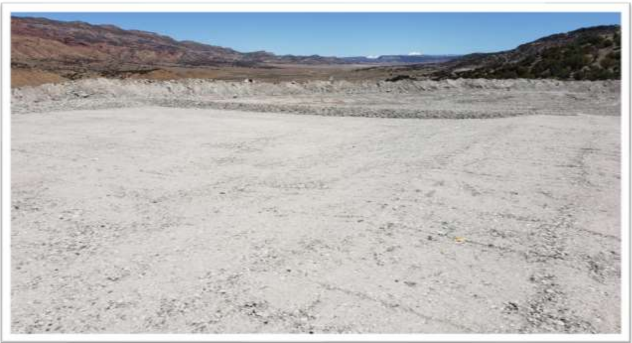
Figure 7: A view looking east-northeast across the ore pad at the West Sunday Mine. The San Miguel mountains are in the distance. This pad was constructed the same as the other pads. This photo does a good job of showing the how the drivable berms were constructed along one edge of the ore pad (the south edge, in this case). These berms are where equipment would access and leave to ore pad to load and unload. The other three sides have steeper, non-drivable berms. Construction and workmanship at this pad were similar to that at the St. Jude and the Sunday Mines.
