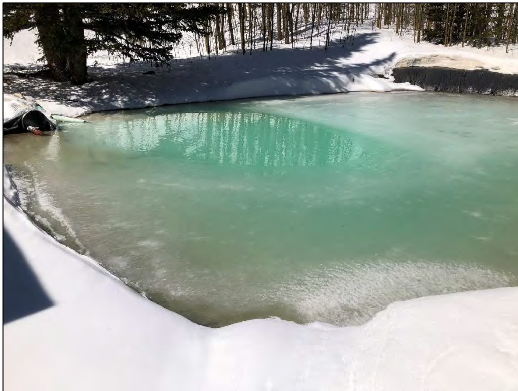
Photo 32. View looking northwest across lined pond #1 in which Cross Mine drainage is discharged for lime treatment before being routed to lined pond #2.
