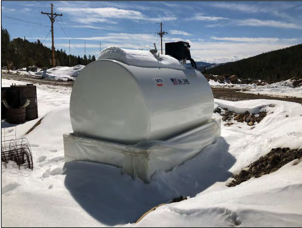
Photo 7. View looking south at new double-walled diesel fuel tank with secondary containment currently stored near the storage shed. This tank is not in use at this time.
