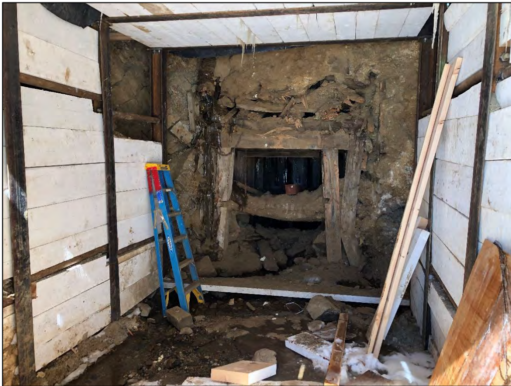
Photo 16. View inside new steel frame entrance constructed around Caribou Mine portal. Water was draining from the portal during the inspection (bottom, left).
