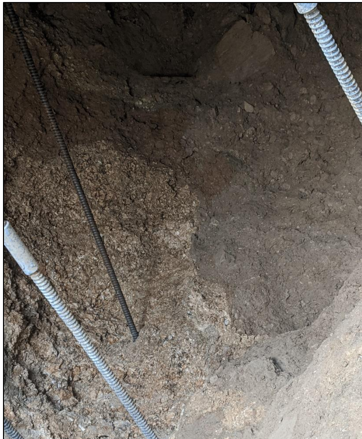
Photograph 5 – Regolith and colluvium exposed in the walls of the collapse void. The threaded bars are some of the spillings which were installed before enlarging the portal excavation.
