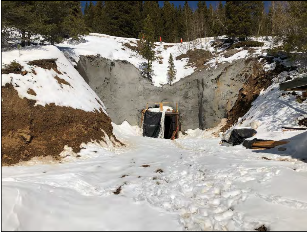
Photo 15. View looking northwest at Idaho Tunnel excavation area, showing new portal location approximately 50-60 feet back from remaining snowshed. Portal daylights to the southeast and is approximately 30 feet below Caribou Road. Note shotcrete applied to slope.
