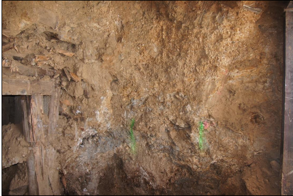
Photograph 4 – Decomposed gneiss overlying weathered and fractured gneiss in the right rib beneath the portal collapse. Green paint marks the approximate location of the next steel sets at 4-ft intervals.
