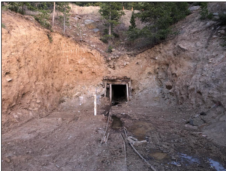
Photograph 7 – Idaho Tunnel Portal following excavation
