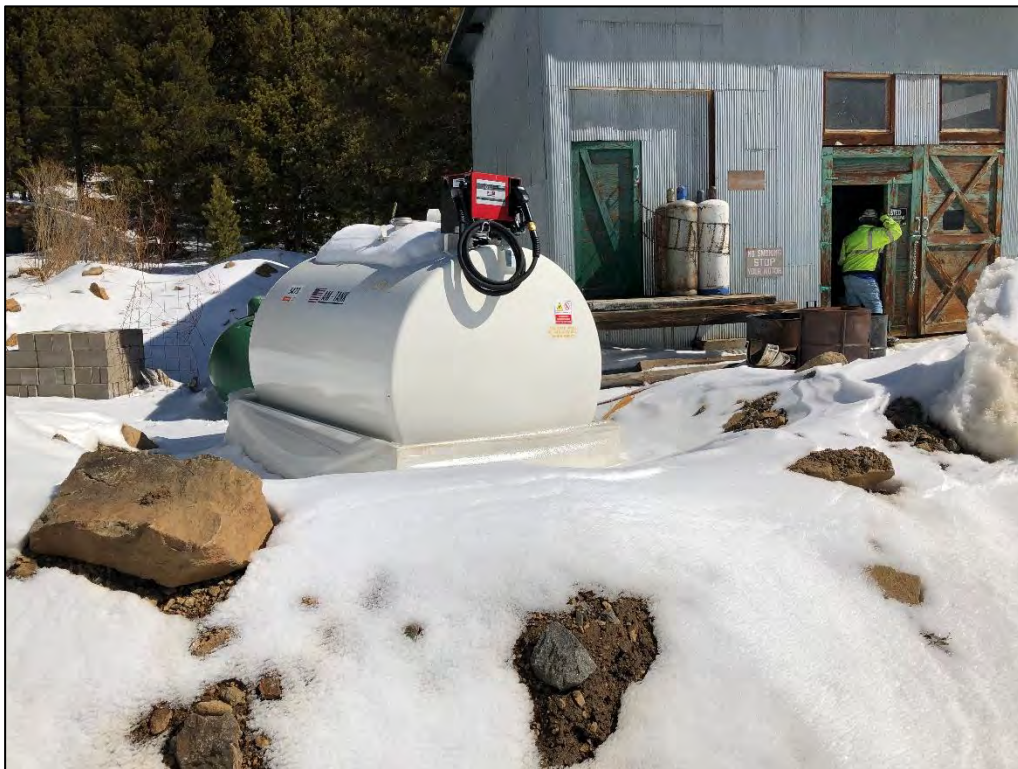
Photo 6. View looking north at new double-walled diesel fuel tank with secondary containment currently stored near the storage shed. This tank is not in use at this time.
