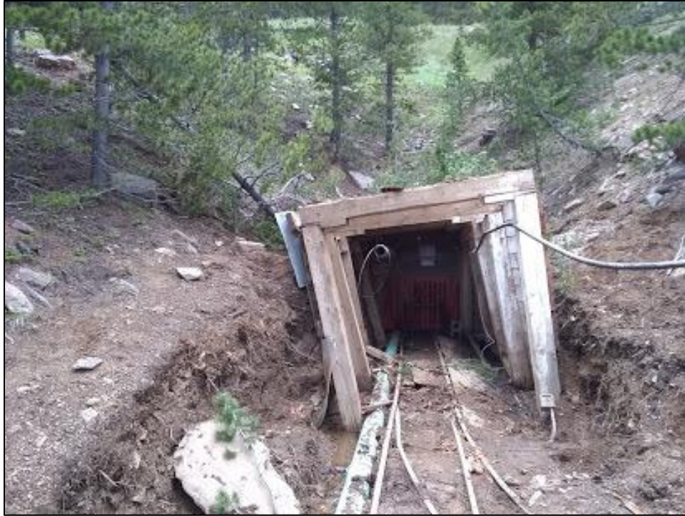
Photograph 1 – Idaho Tunnel Portal prior to Rehabilitation
