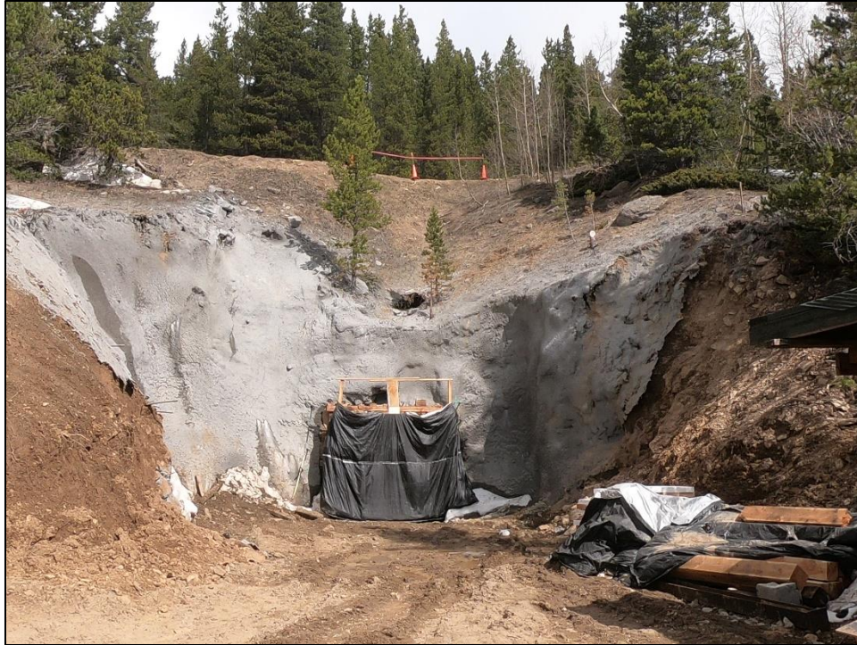
Photograph 2 – Current Condition of the Idaho Tunnel Portal. The three safety cones and caution tape at the top of the slope mark the edge of Country Road 126 (Caribou Road). The crown hole over the void is visible between the two small trees above the portal.
