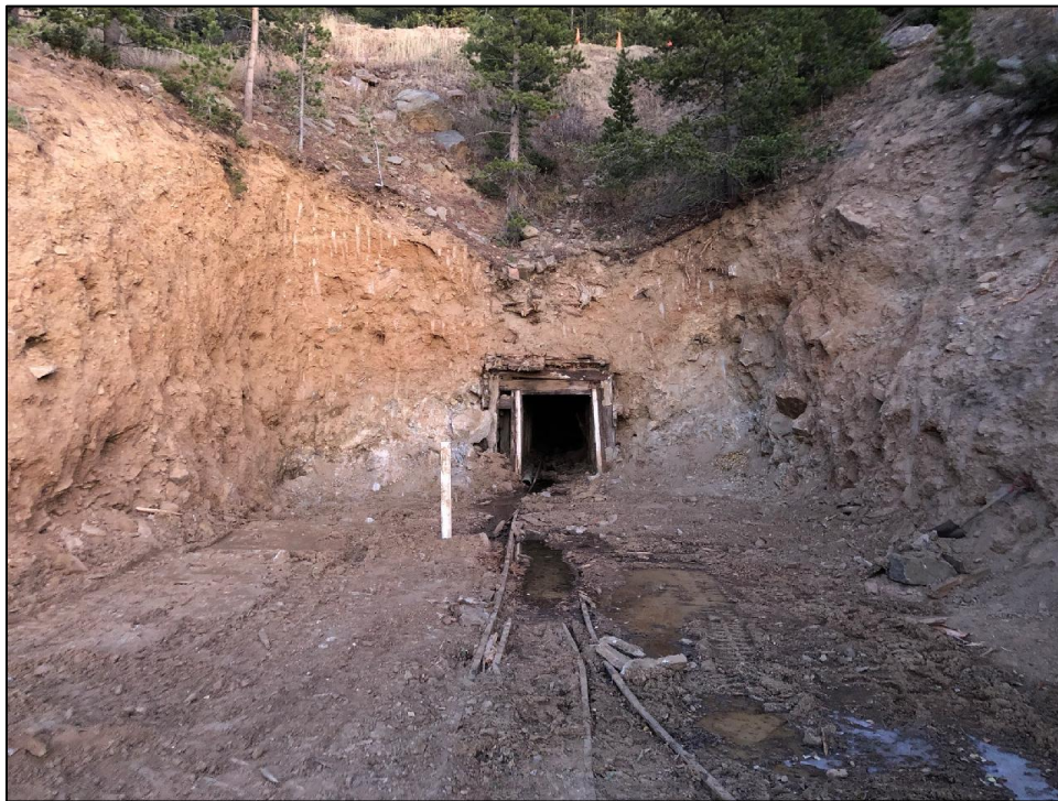
Photograph 7 – Idaho Tunnel Portal following excavation
